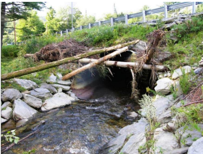
A wide bank full width constricted by the existing culvert.
