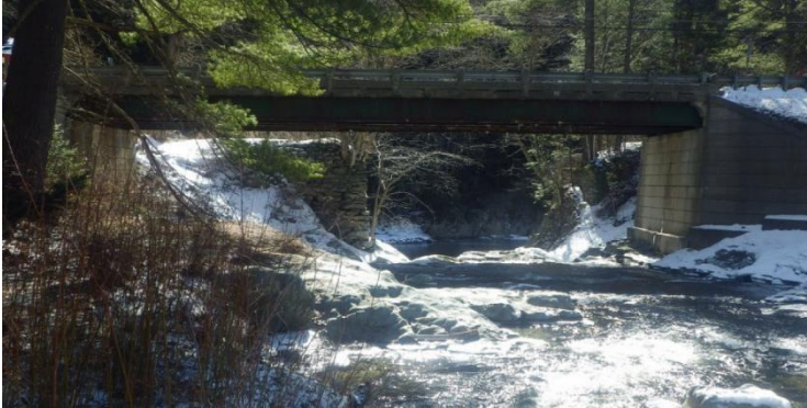
Bridge 84 over the North Branch
