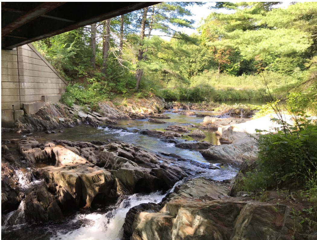
Figure 3.3: Facing upstream; note exposed bedrock throughout including at wingwall location.
