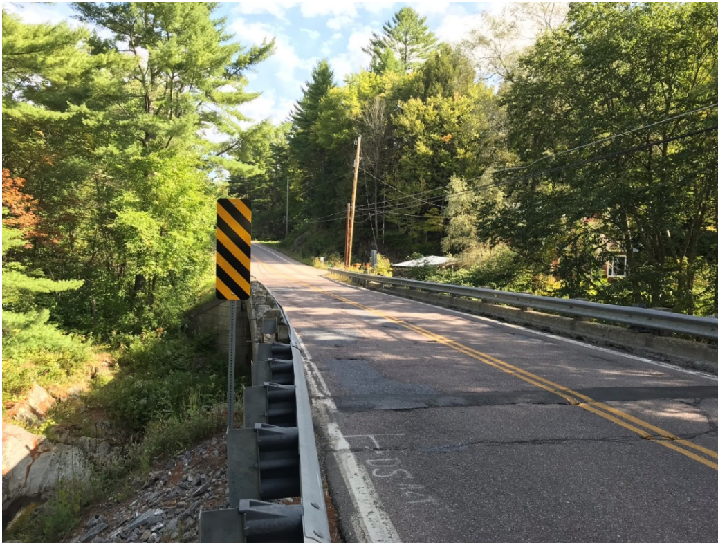
Figure 3.1: Facing north along VT Route 12; note overhead utilities to east of roadway.
