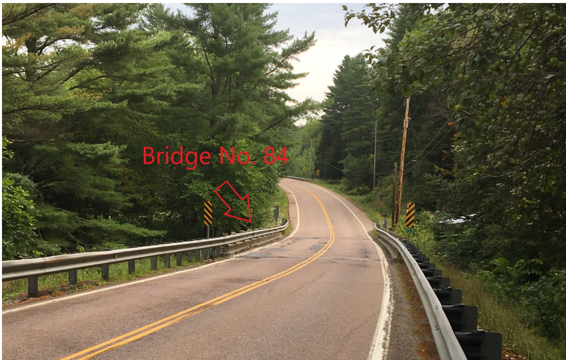
Figure 8: Looking north on VT-12 towards bridge number 84 in Worcester.
