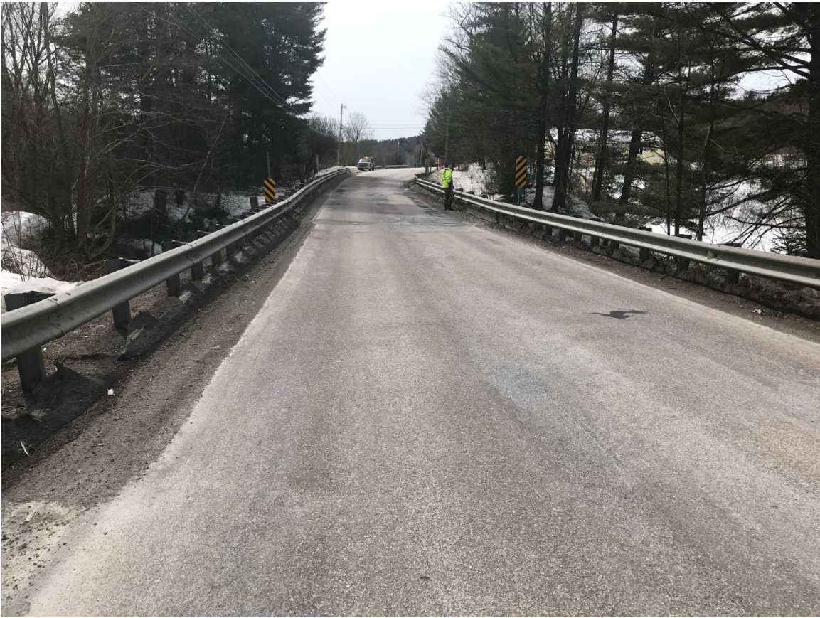
Photo 1: Looking South over Bridge 84
