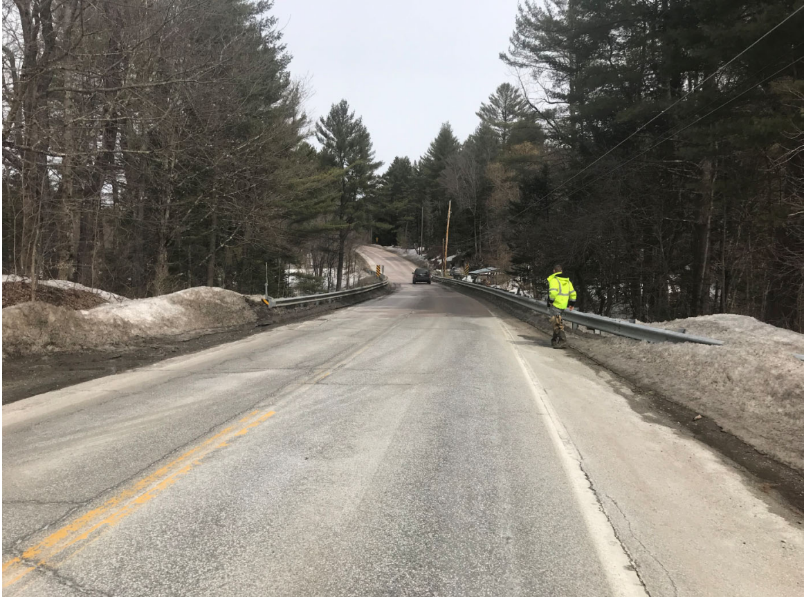
Photo 2: Looking North over Bridge 84
