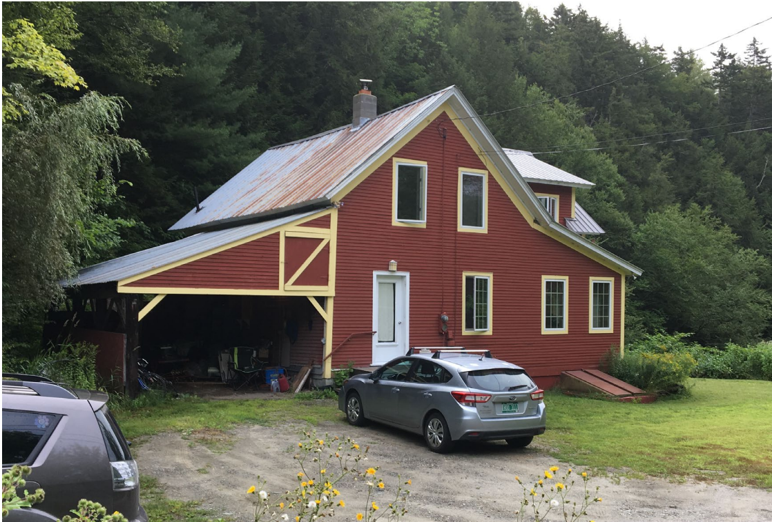
Figure 5: Historic resource at 597 VT-12 that is no longer eligible for the National Register. Door and windows have been replaced and the shed roof additions on either side obscure the original building configuration.
