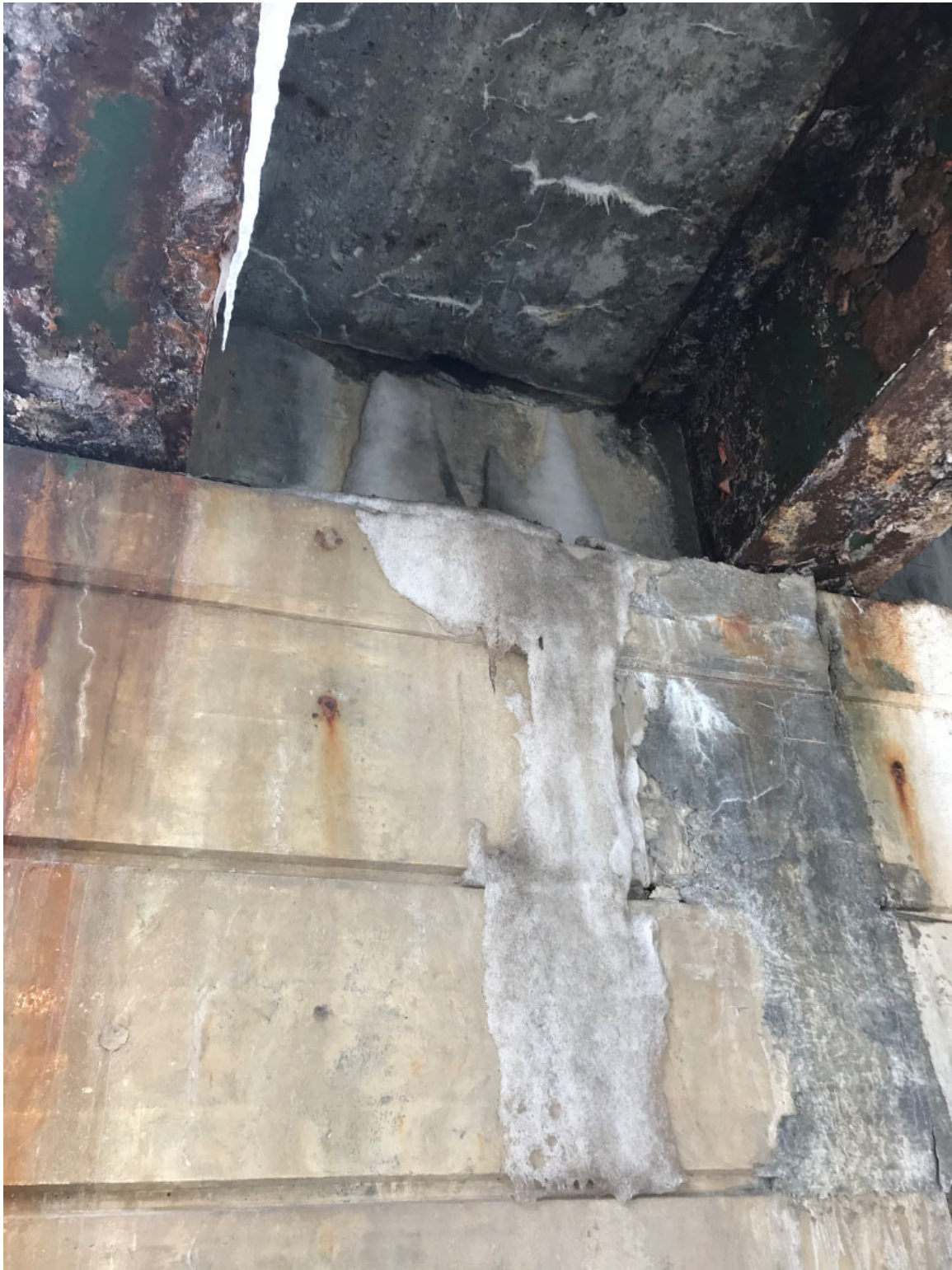
Photo 8: Backwall Leakage
