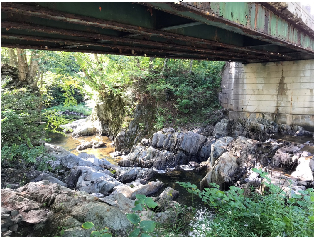
Figure 3.5: Facing downstream; note exposed bedrock throughout.
