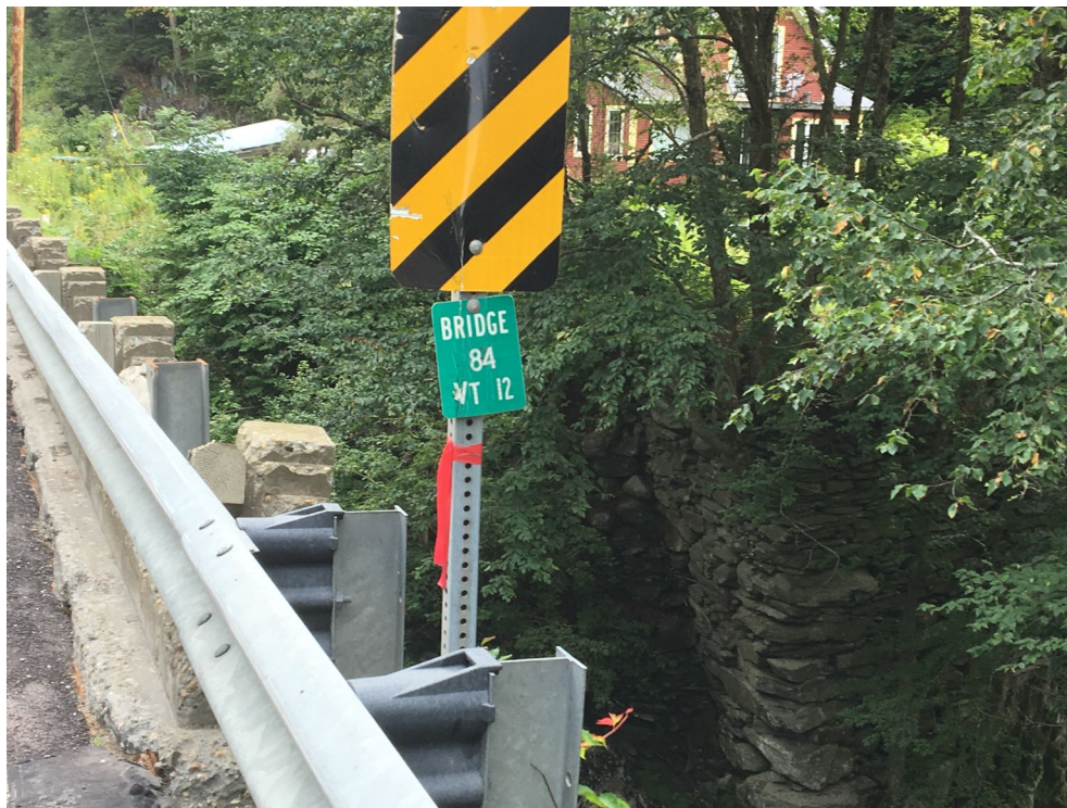
Figure 4: Early dry laid abutments from a previous structure are viewable in the rightmost portion of this image. This is also visible in Figure 2.
