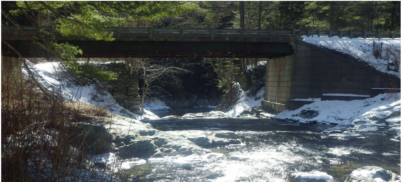
Figure 2: Bridge number 84 in Worcester.
