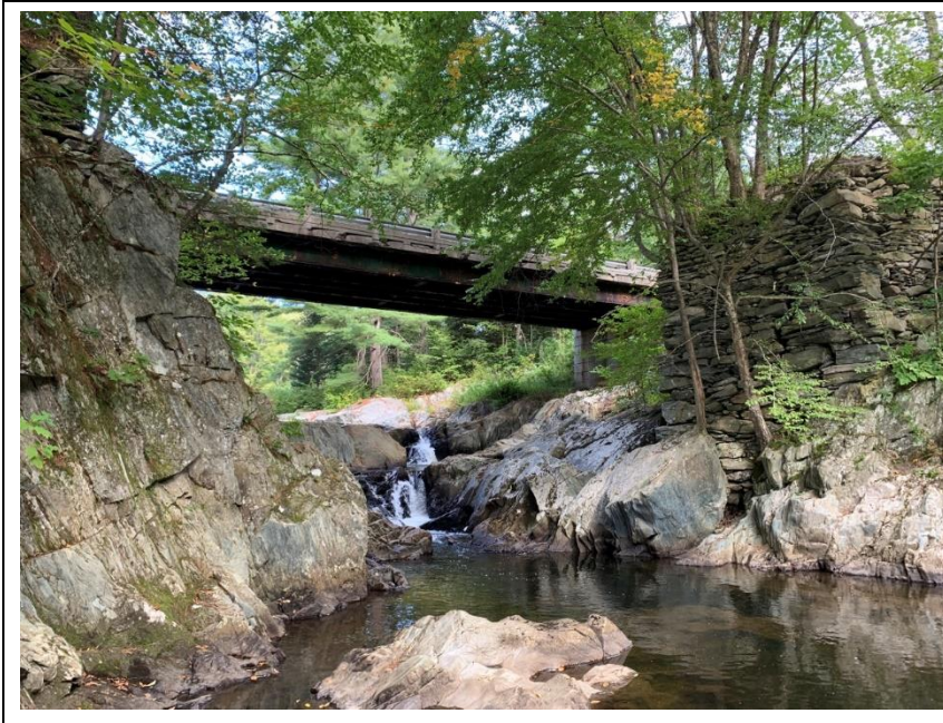
Downstream of structure looking upstream September 10, 2019
