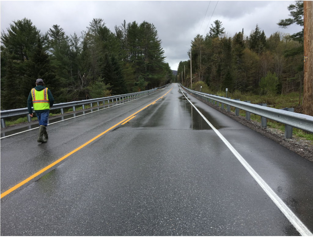
Picture 1: Looking North on VT Route 12 over Bridge 87
