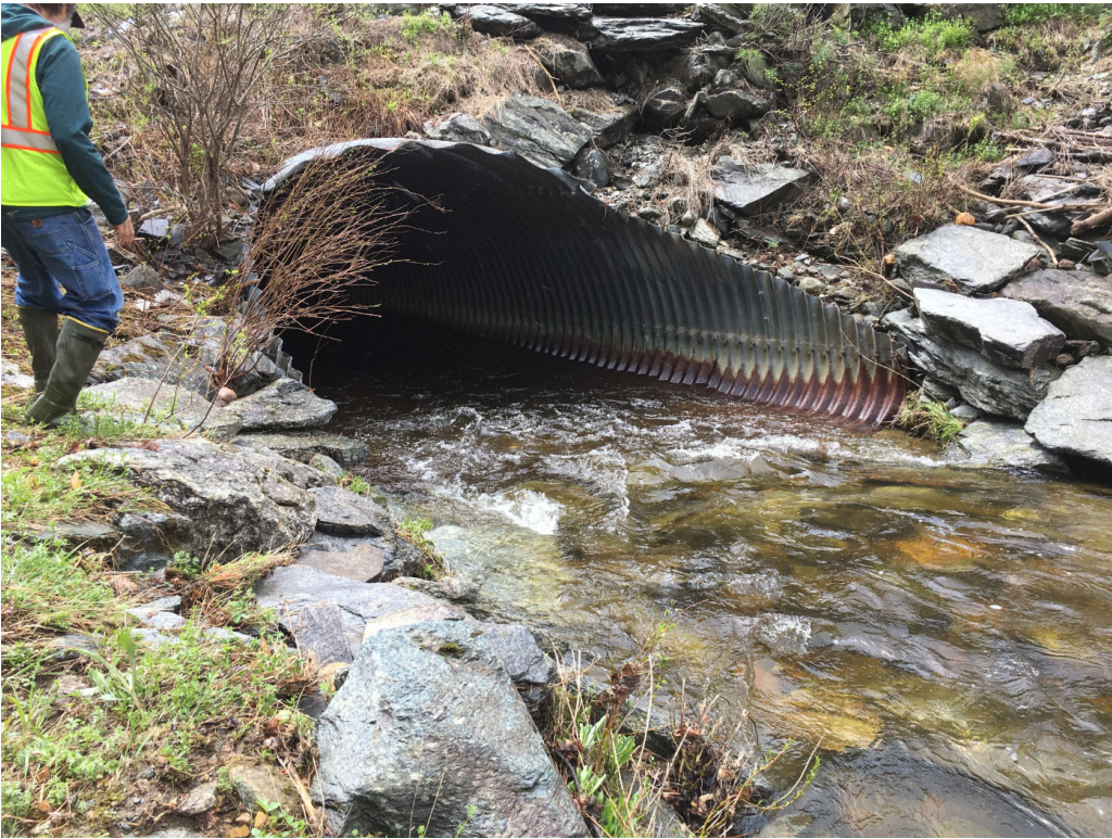
Picture 4: Culvert Inlet
