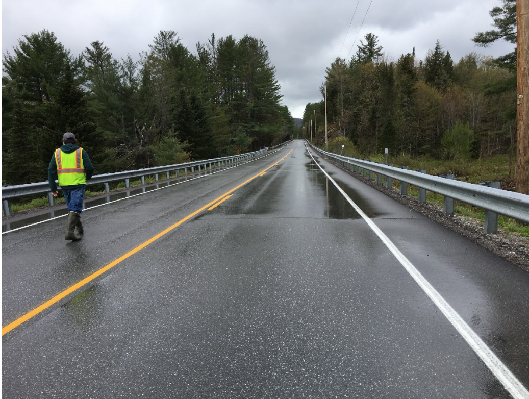
Figure 3.1: Overhead utilities above culvert along VT 12. [Structures photo dated May 2019]
