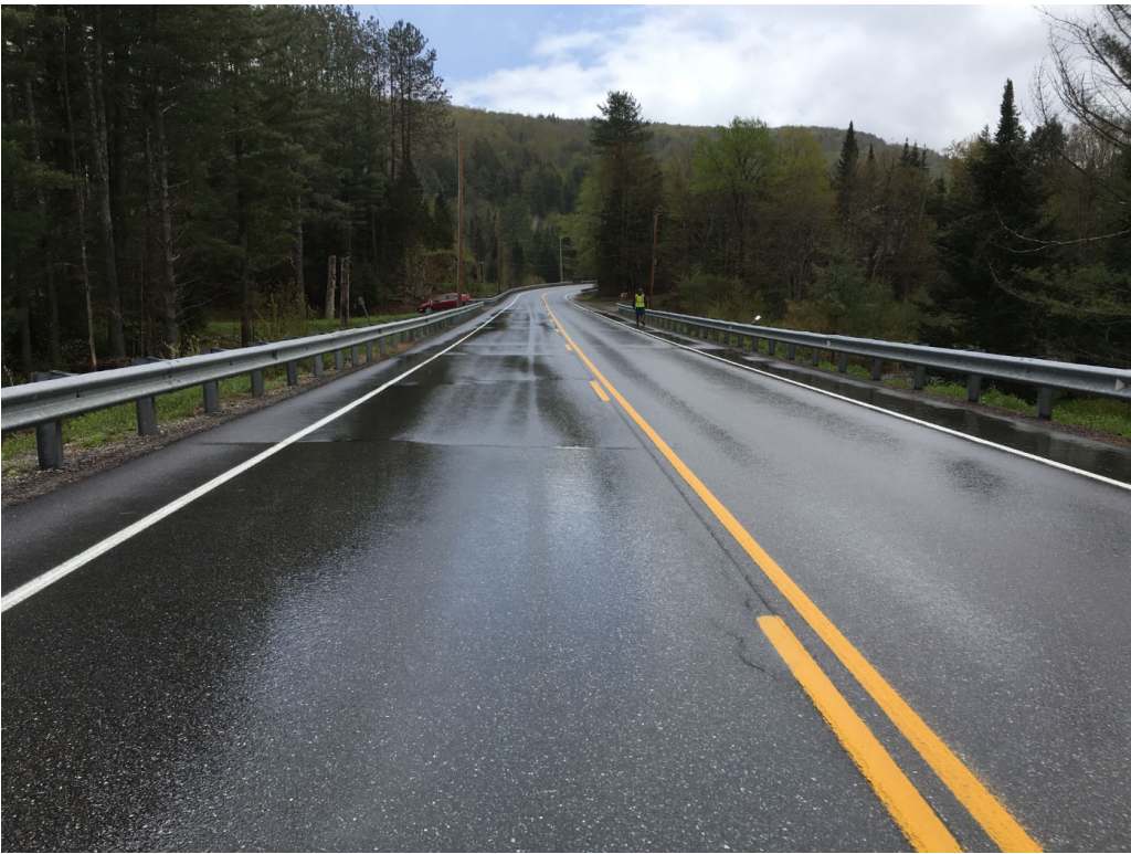
Picture 2: Looking South on VT Route 12 over Bridge 87
