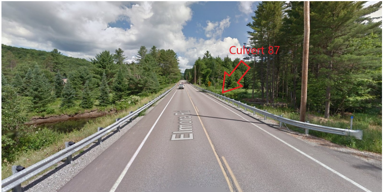
Figure 3: Google Maps view of the survey area and culvert 87.
