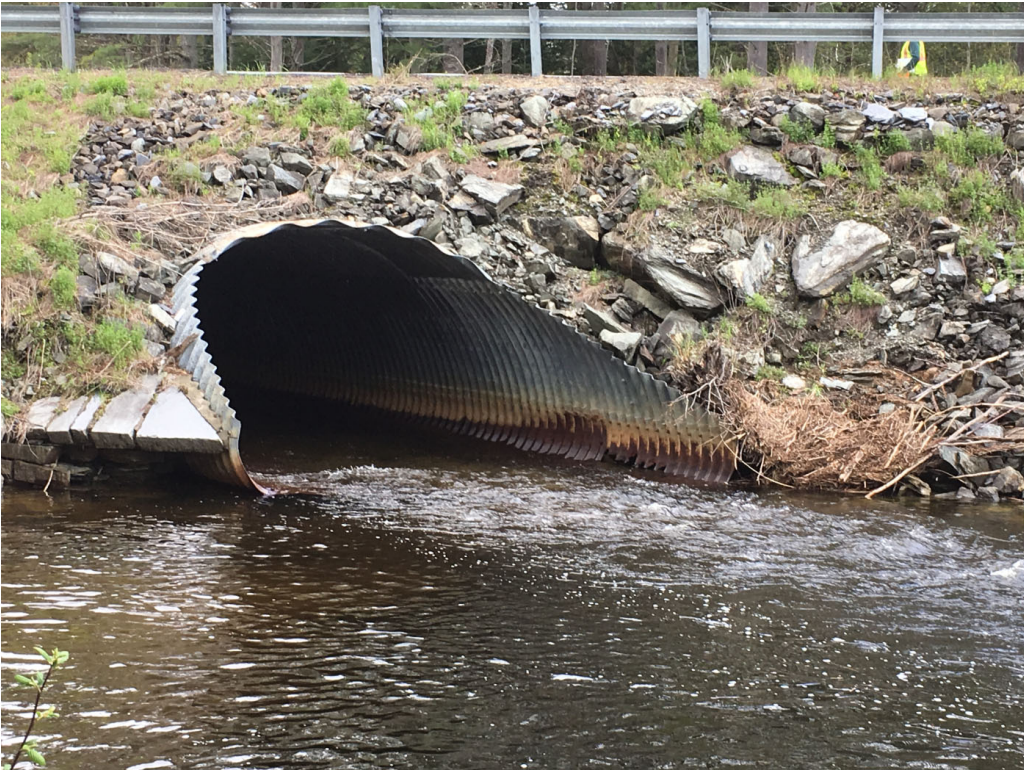
Picture 3: Culvert Outlet
