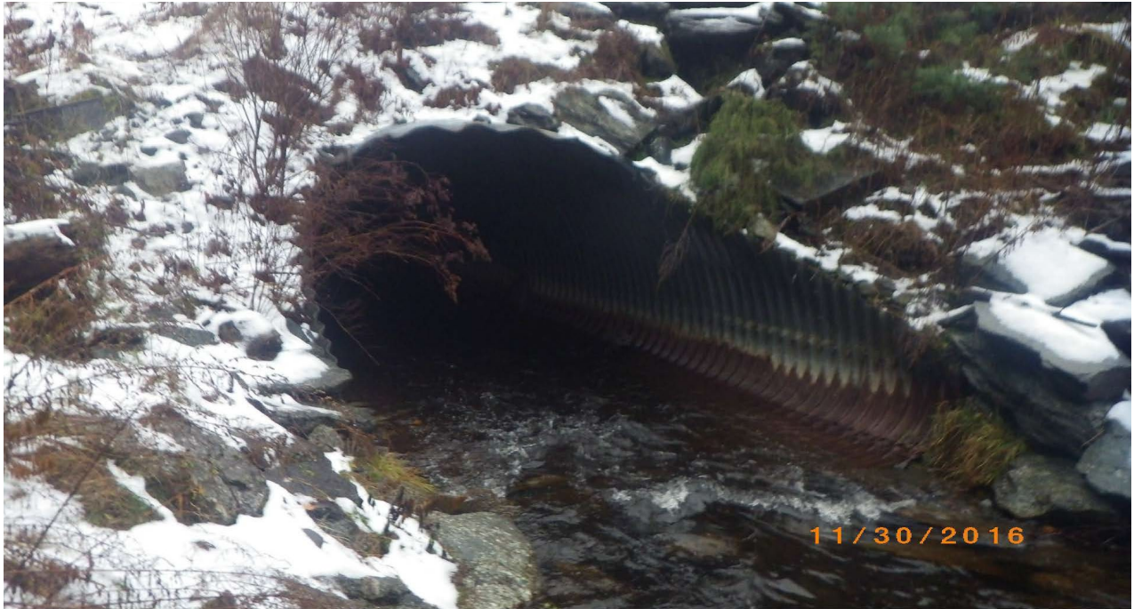
Figure 2: Culvert 87 in Worcester.
