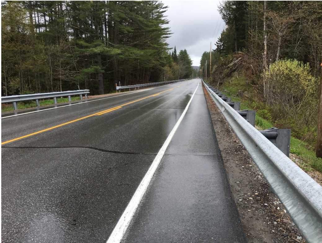
Figure 3.3: Ledge cut north of the culvert. [Structures photo dated May 2019]
