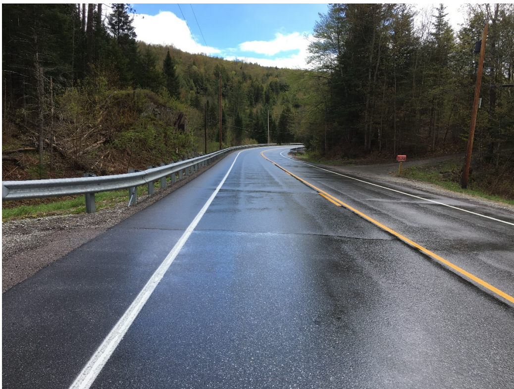
Figure 3.4: Ledge cut located south of the culvert. [Structures photo dated May 2019]
