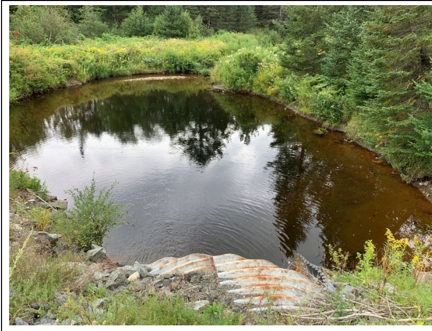
Culvert 87:Downstream pool September 10, 2019
