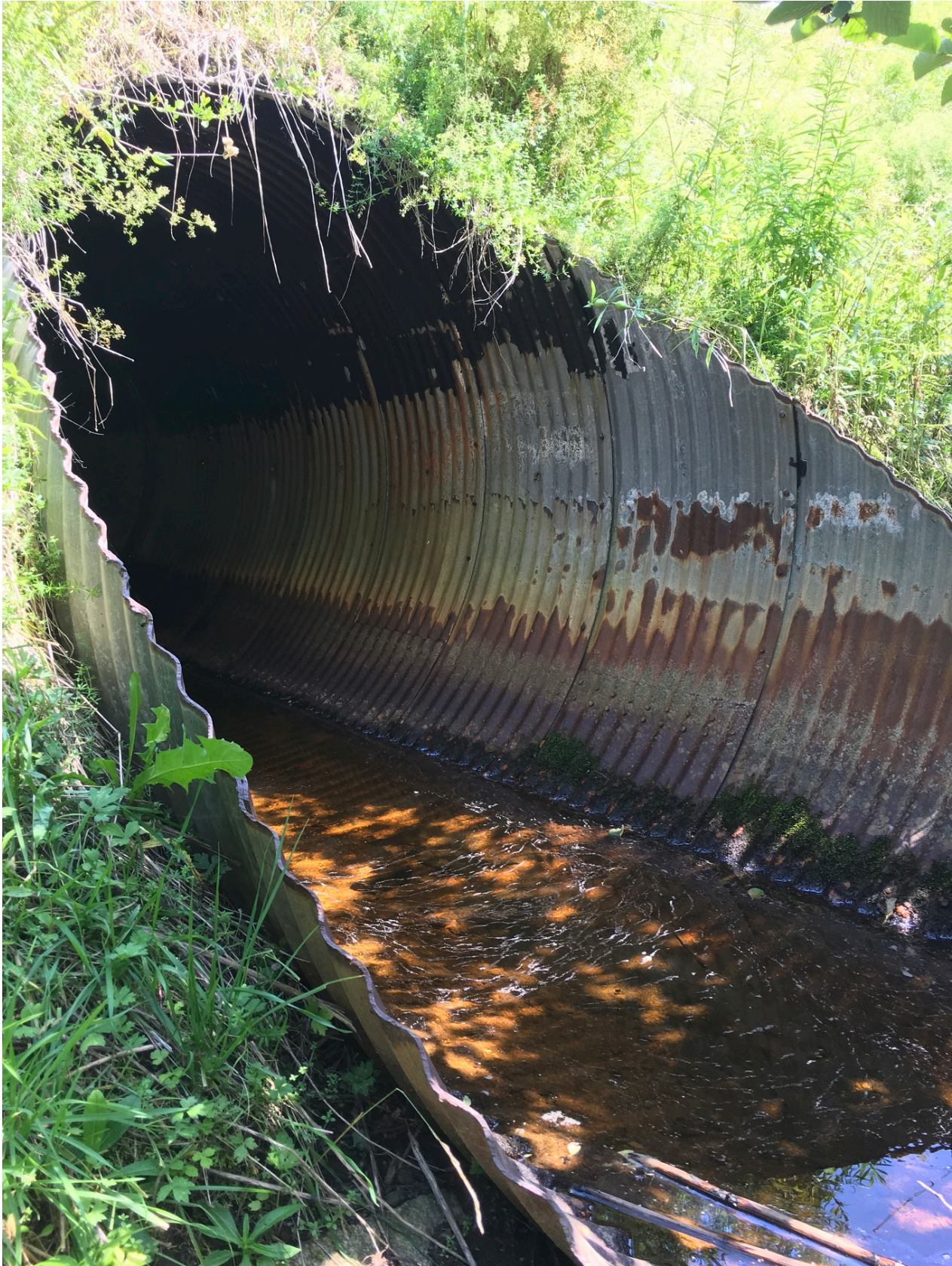
Figure 3: Photo of culvert from west side of road
