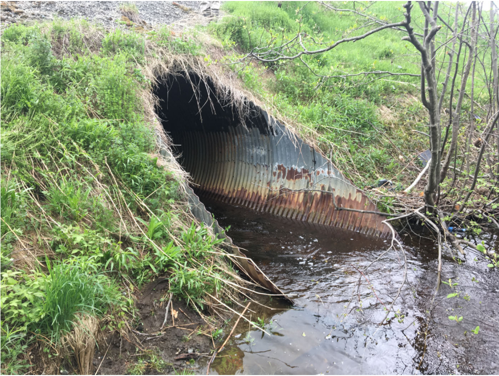
Picture 3: Culvert Outlet
