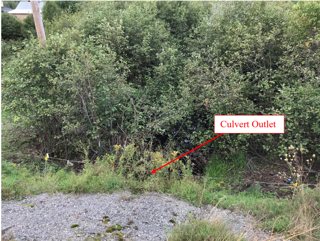
Figure 3.2: Facing downstream; note vegetated embankments adjacent to culvert outlet.
