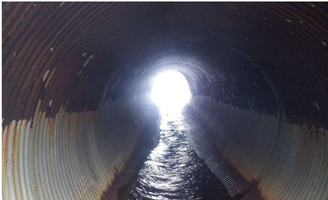
Figure 2: Culvert 94 in Elmore.
