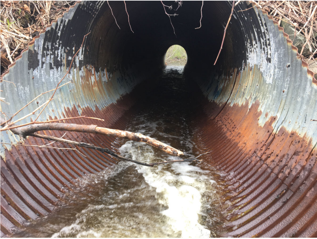
Picture 5: Culvert Barrel
