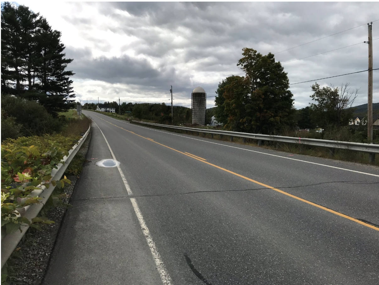
Figure 3.1: Facing south along VT Route 12; note overhead utilities to west of roadway. These utilities are not anticipated to interfere with potential boring operations.
