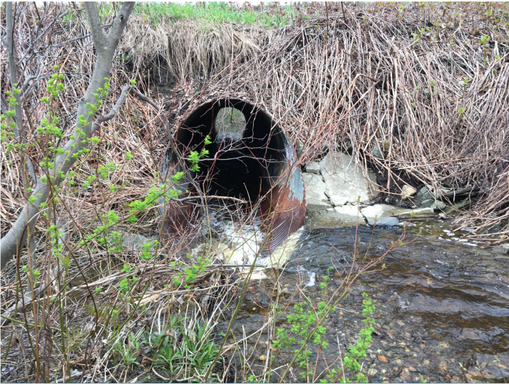
Picture 4: Culvert Inlet
