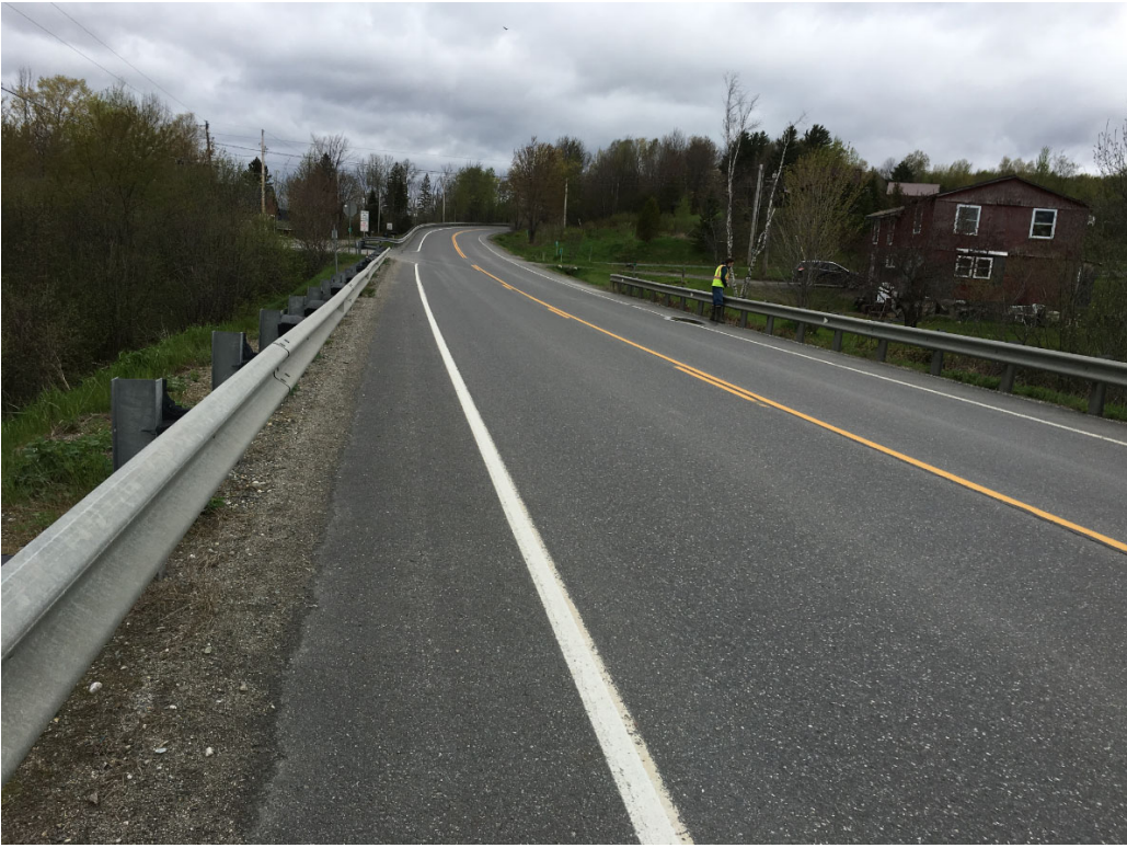
Picture 1: Looking North on VT Route 12 over Bridge 94
