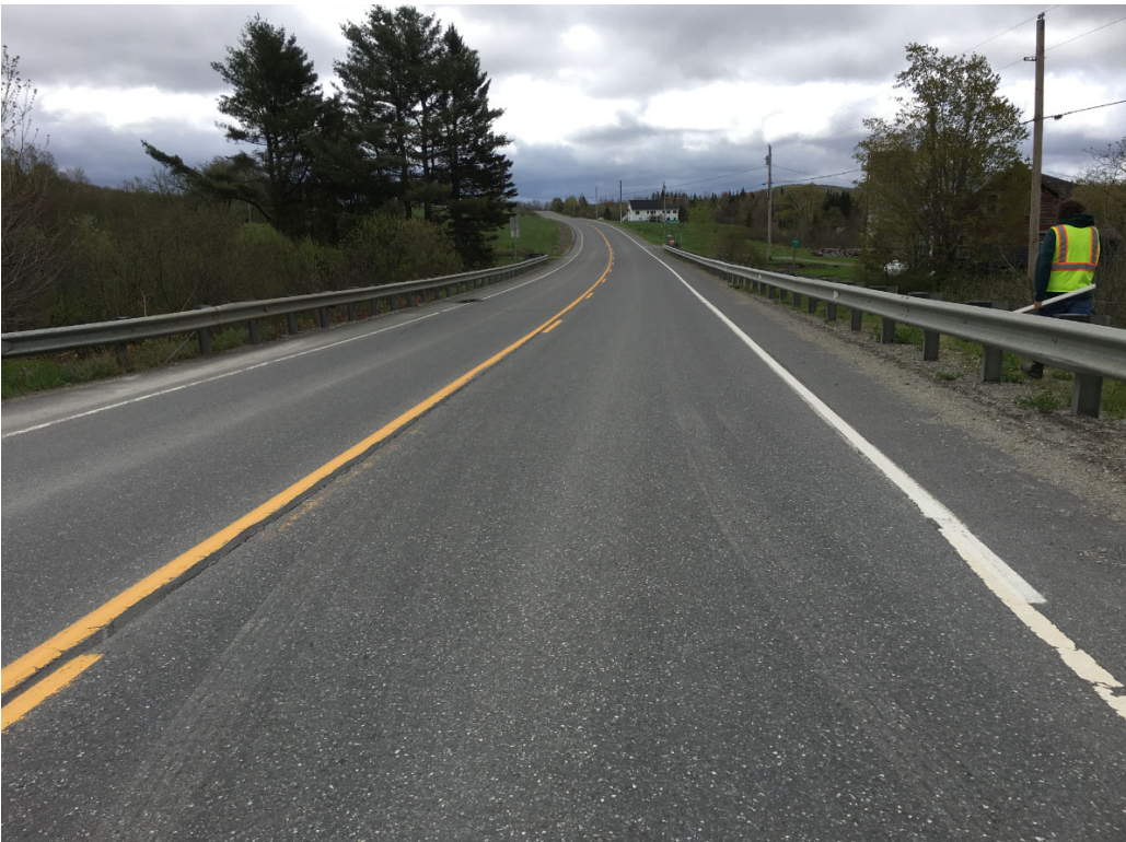
Picture 2: Looking South on VT Route 12 over Bridge 94
