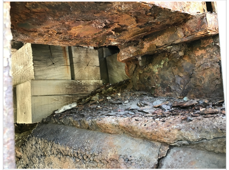
Pier #2 Bay #1 Timber Blocking
