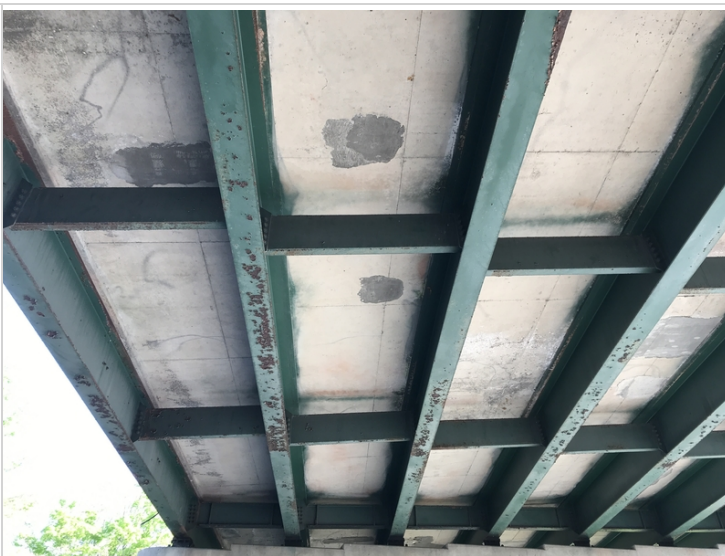
Span #3 Deck Bays #1-2-3 from South End
