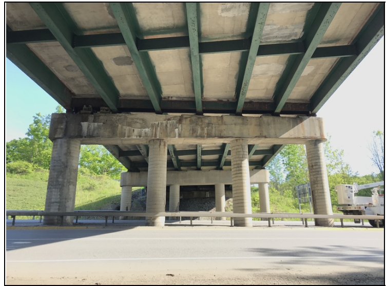
Pier #2 Span #2 and Timber Blocking
