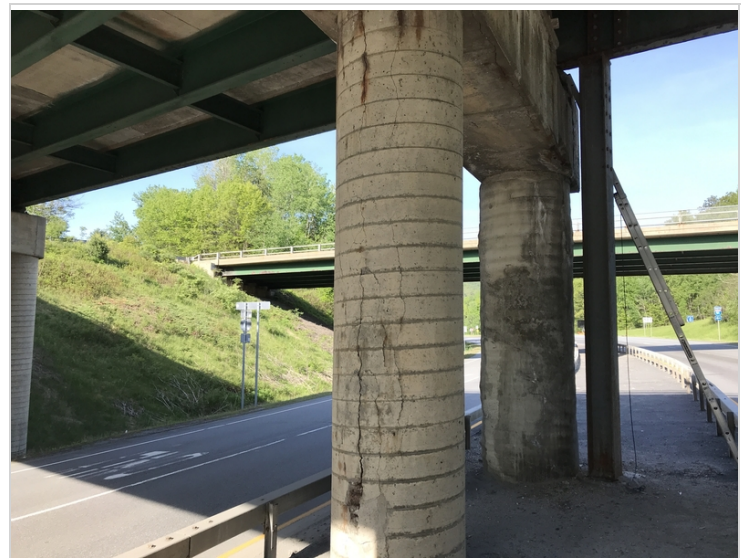
Pier #2 Columns #1 and #2
