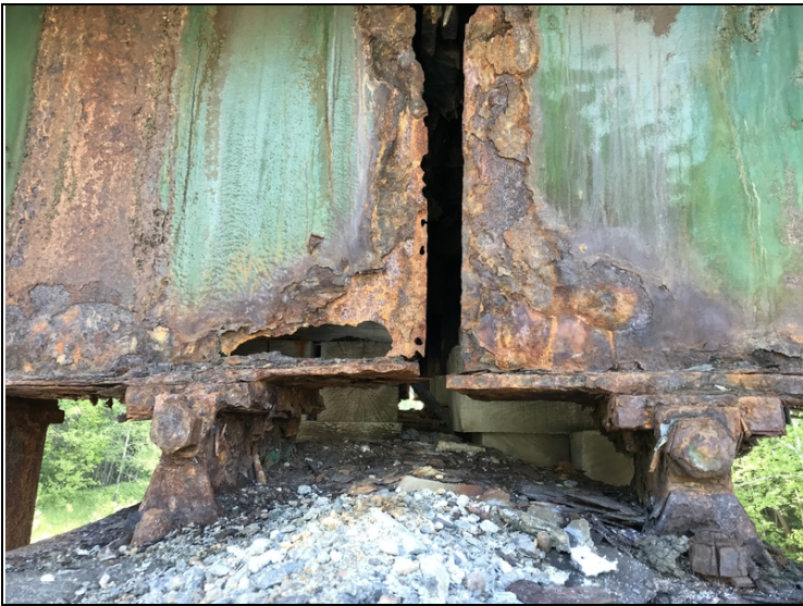
Pier #2 Beams #1 in Spans #2 and #3
