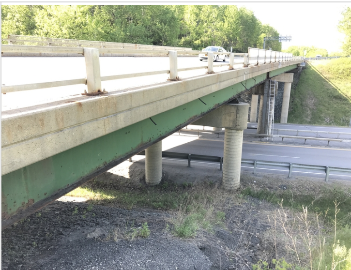
West fascia facing south
