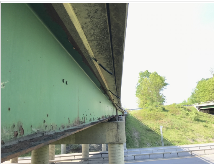
Western Beam / Fascia from Span #4
