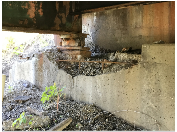
Beam #1 at Abutment #2
