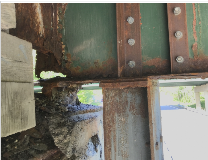
Pier #2 Beam #1 in Span #3 Bracing
