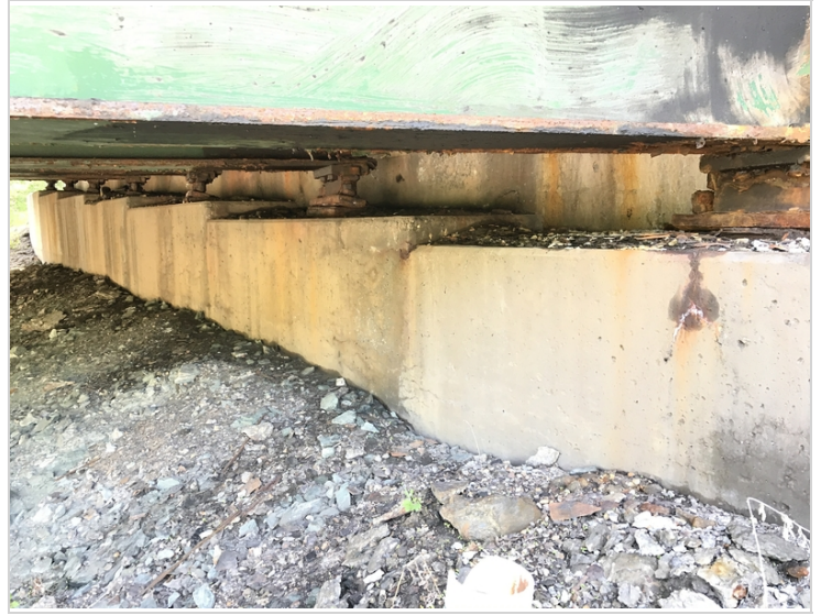
Bearings at Abutment #1
