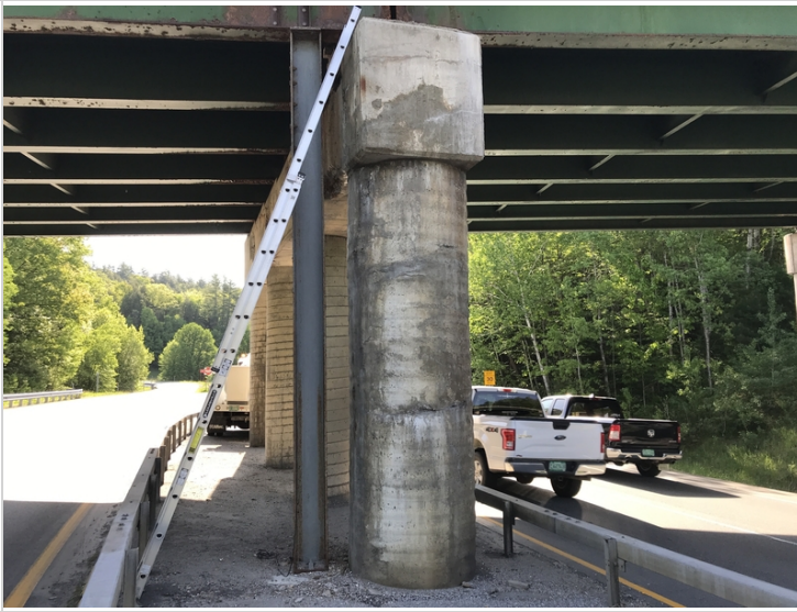
Pier #2 Column #1 and Support Beam for Beam #1 in Span #3
