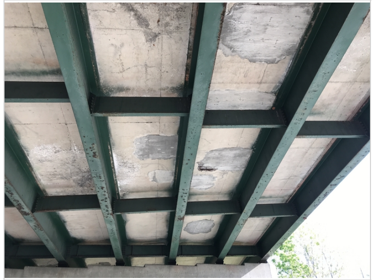
Span #3 Deck Bays #4-5-6 from South End
