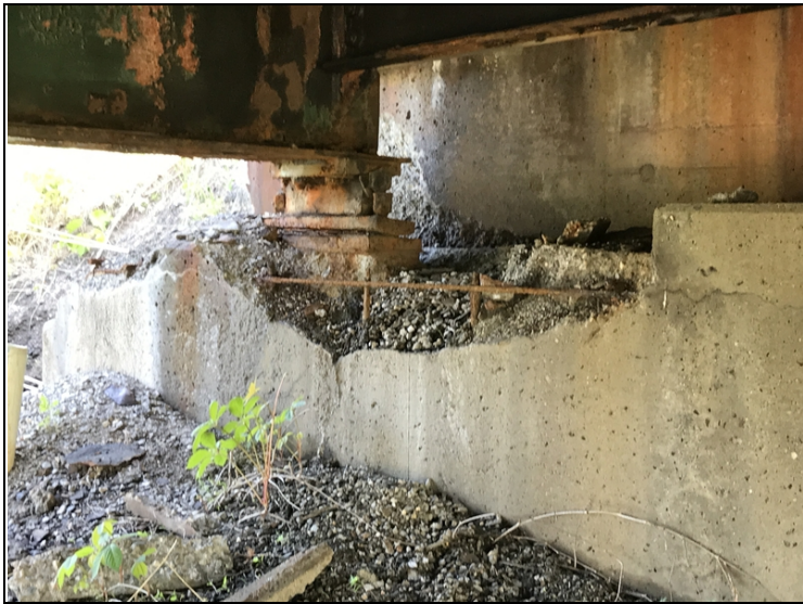
Beam #1 at Abutment #2
