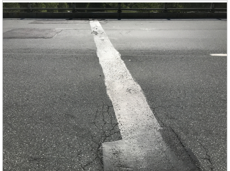
Asphaltic Plug Joint over Pier #2
