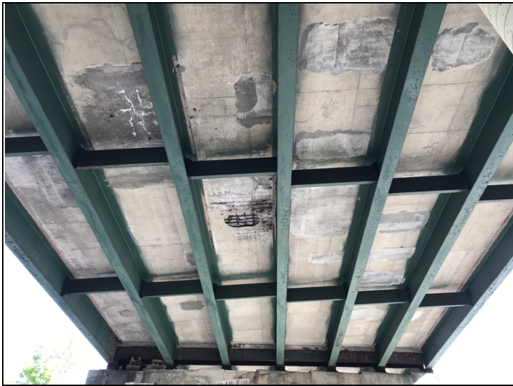
Span #2 Deck Facing North
