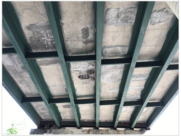
Span #2 Deck Facing North
