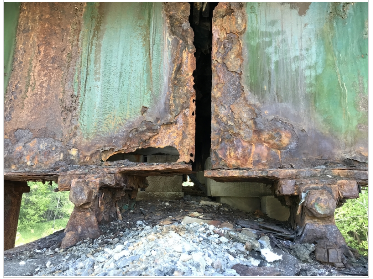
Pier #2 Beams #1 in Spans #2 and #3
