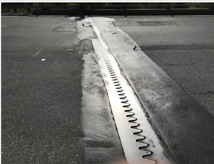
Asphaltic Plug Joint over Abutment #2
