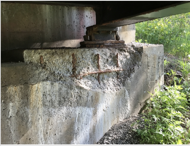
Beam #7 at Abutment #2
