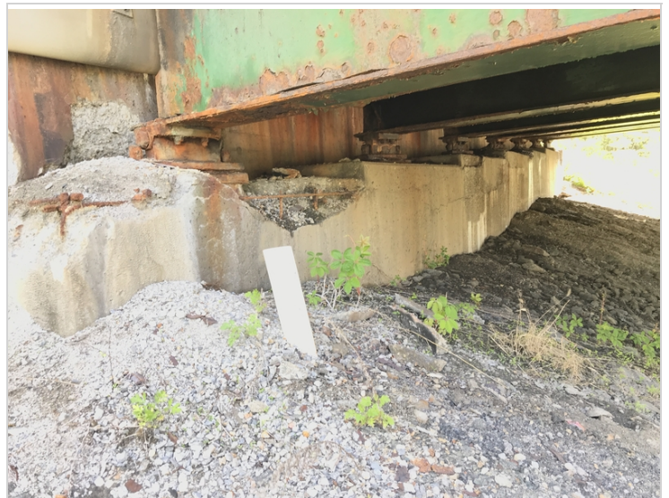
Abutment #2 from West Side
