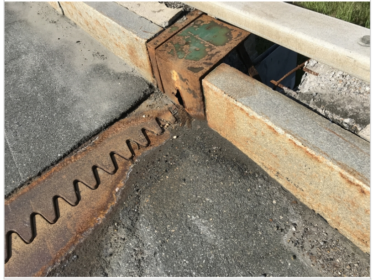
Southwest Corner of Joint over Abutment #1
