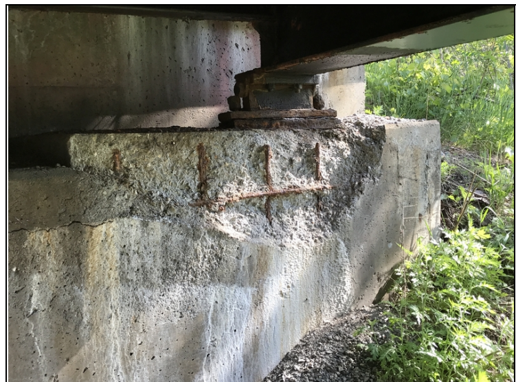
Beam #7 at Abutment #2
