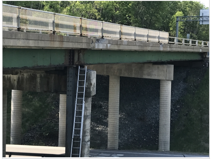
Western Fascia at Midspan
