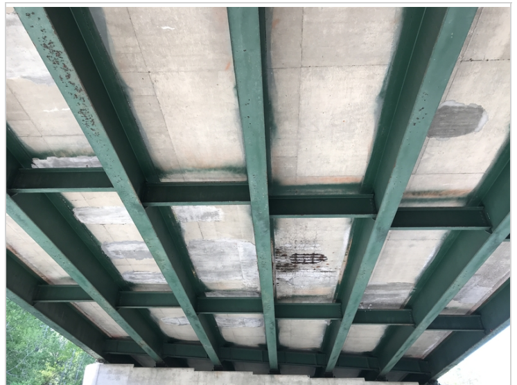
Span #2 Deck from North
