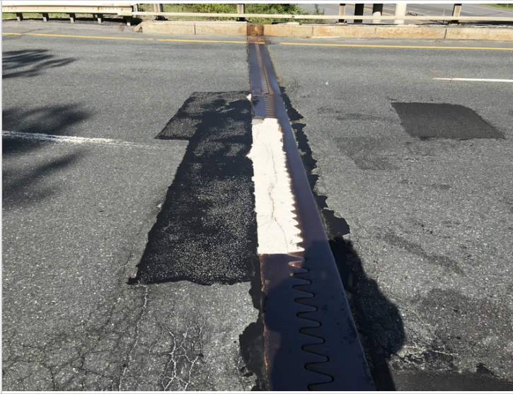
Steel Finger Plate Joint over Abutment #1
