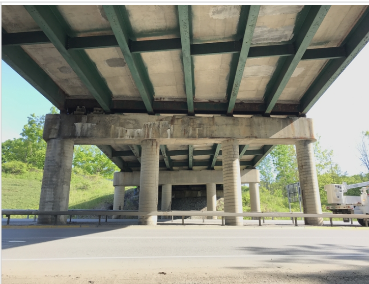
Pier #2 Span #2 and Timber Blocking
