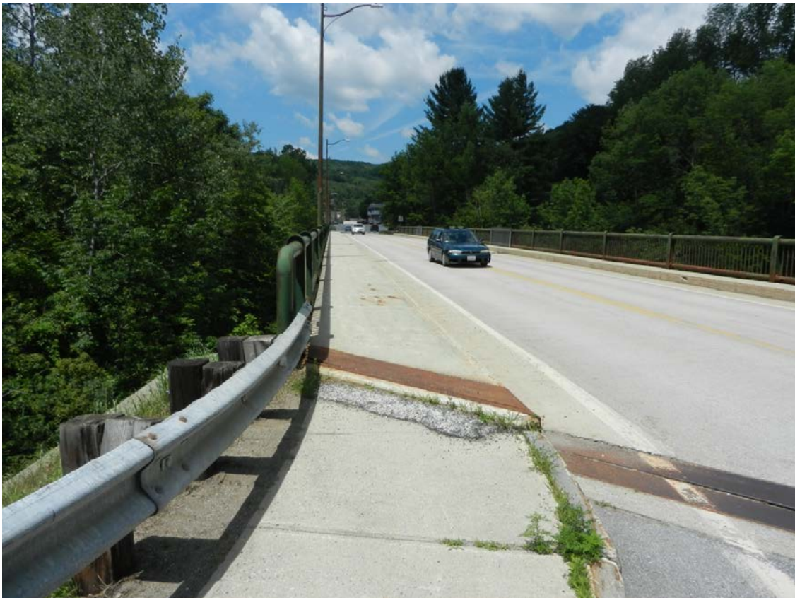
Figure 1. Looking North on VT-100
