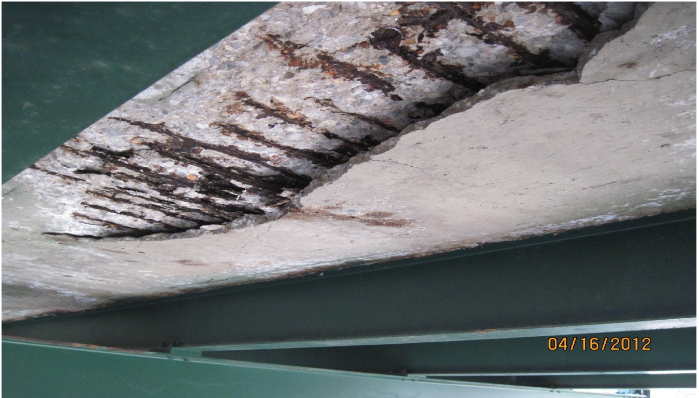
Delaminating Deck
