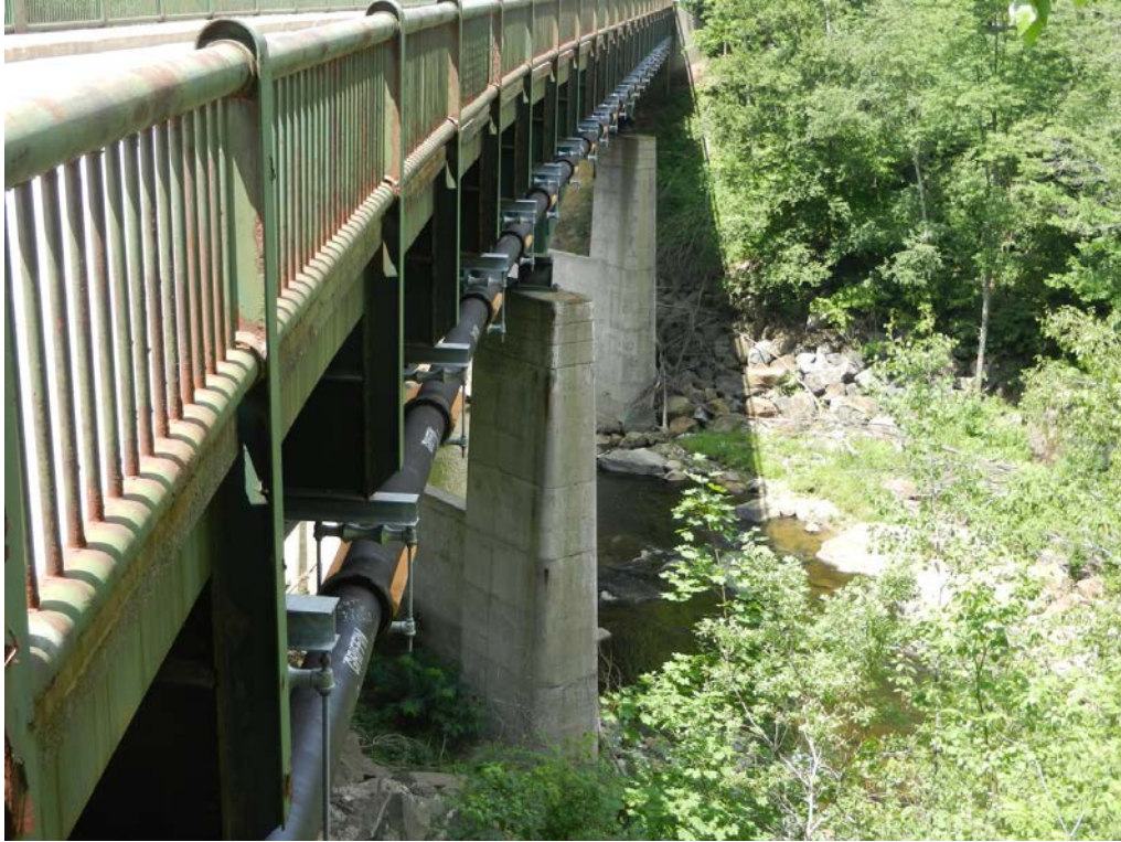
Figure 3. Upstream side of the bridge, looking North on VT-100
