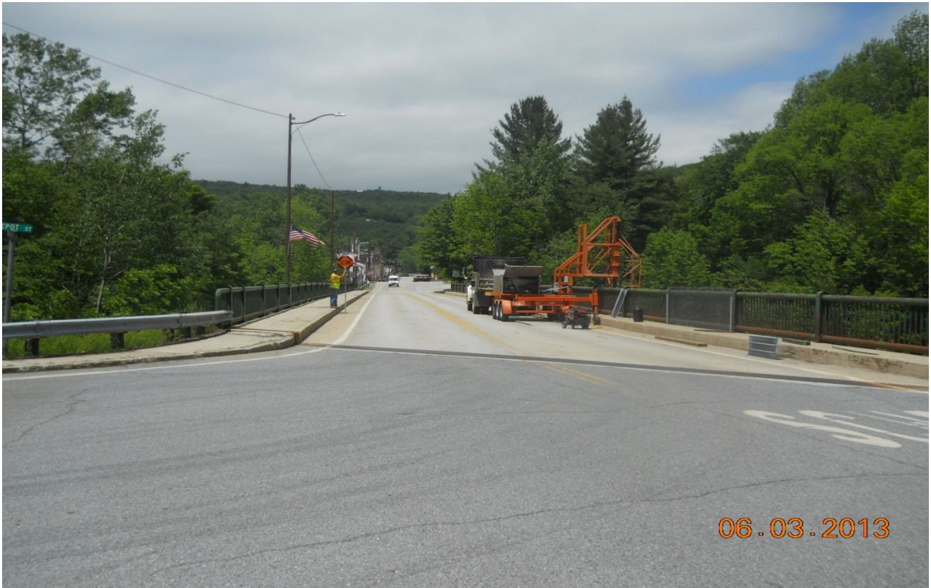
Bridge 25 Looking West
