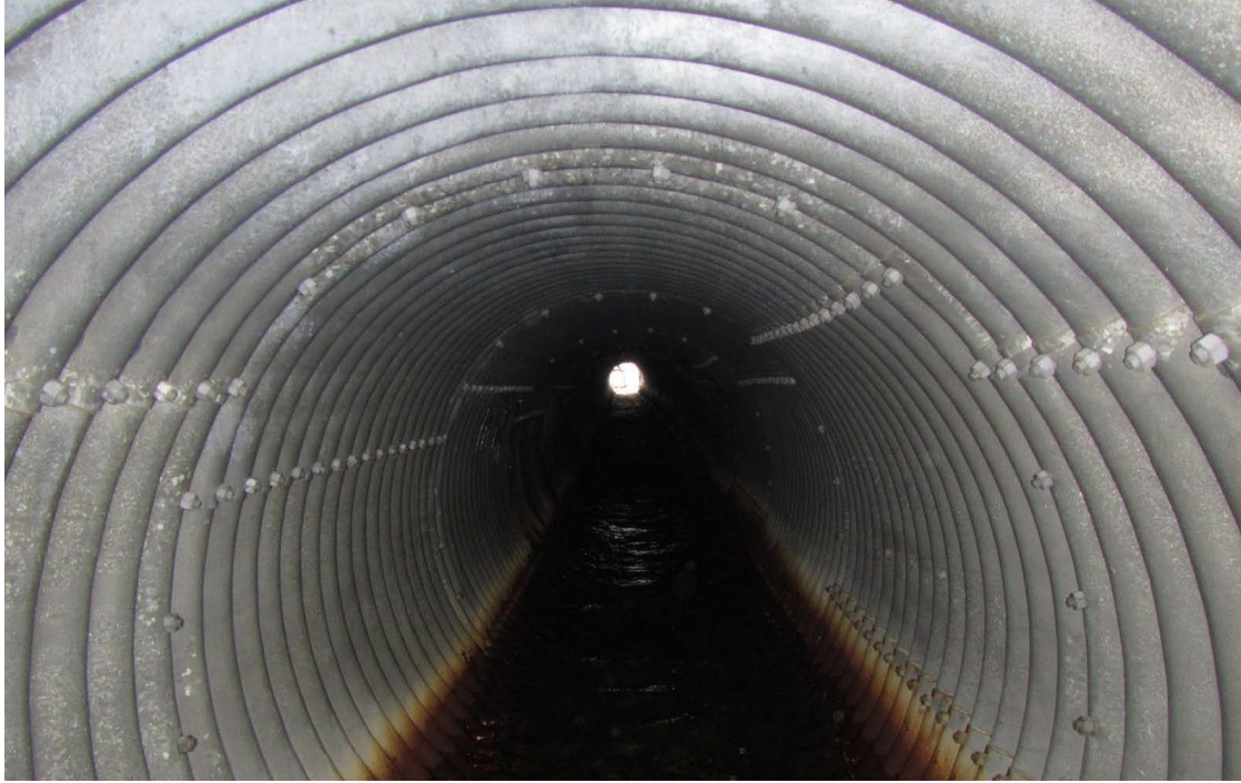
Figure 2: Culvert 90 in Elmore on VT-12.
