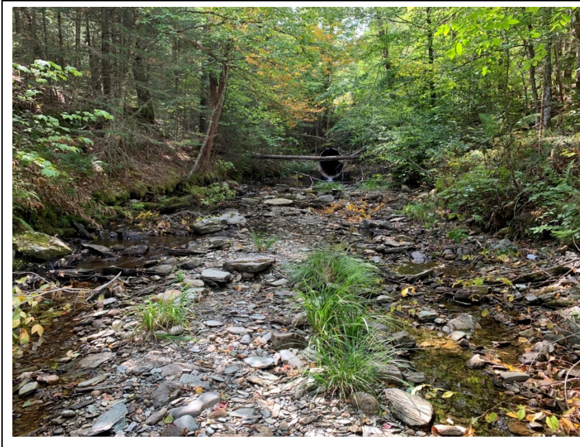
Unnamed Tributary Downstream of Culvert 90 September 16, 2019
