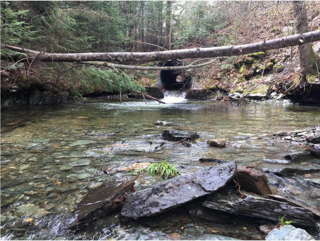
Picture 3: Culvert Outlet
