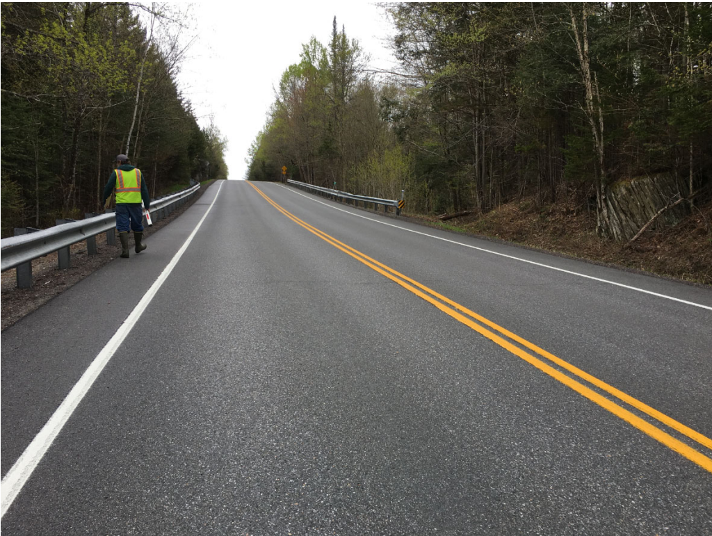
Picture 2: Looking South VT Route 12 over Bridge 90
