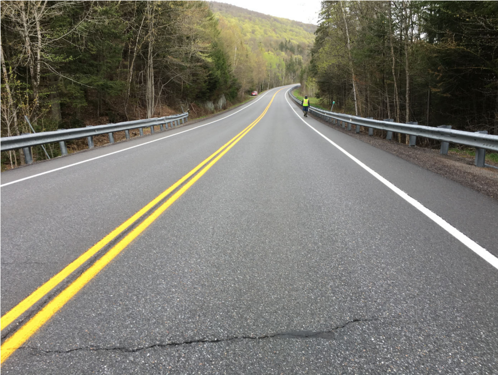
Picture 1: Looking North on VT Route 12 over Bridge 90
