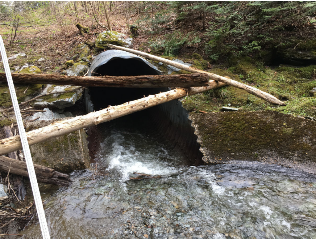
Picture 4: Culvert Inlet
