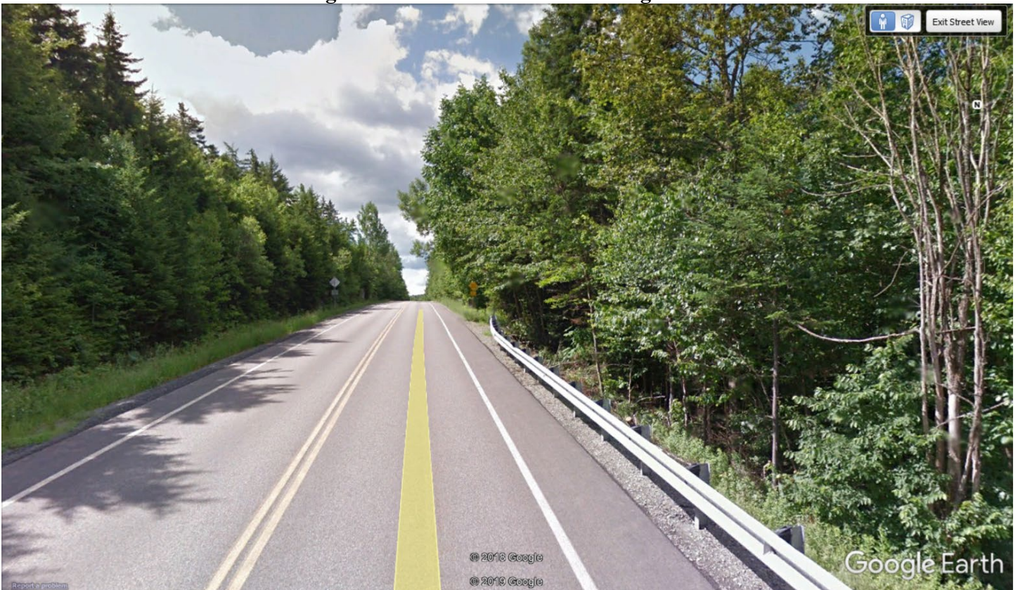
Figure 6: View from the road facing south
