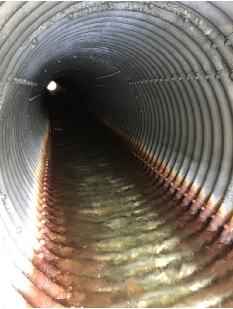
Picture 5: Culvert Barrel
