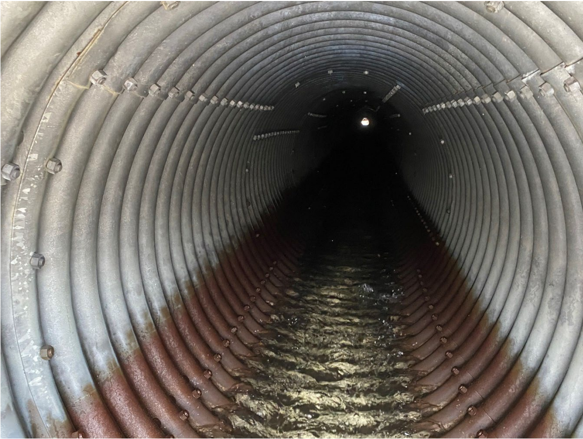
Looking up through culvert to the inlet from the outlet side.
