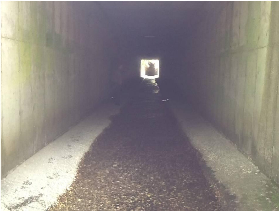
Interior of Pineo Brook culvert, with I-89 median opening visible
