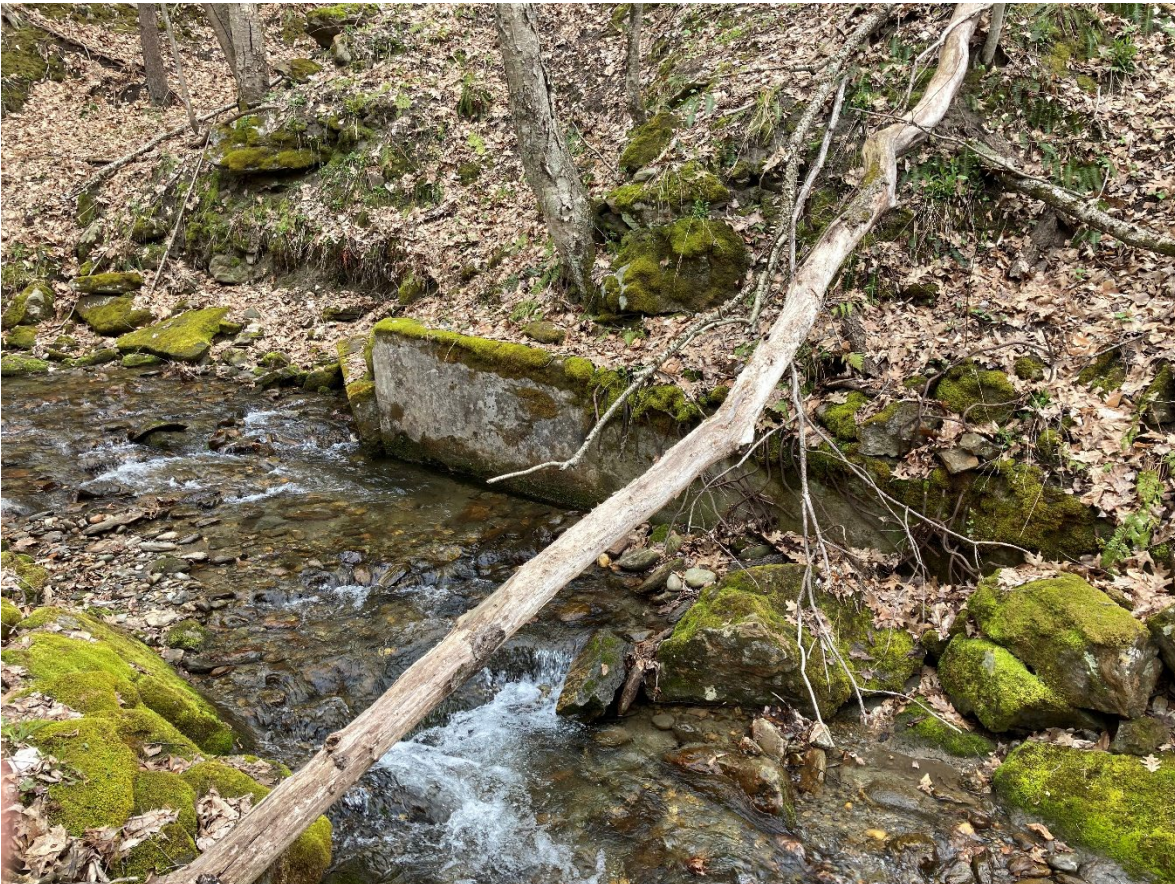
Concrete "wingwall" on east bank upstream of inlet.
