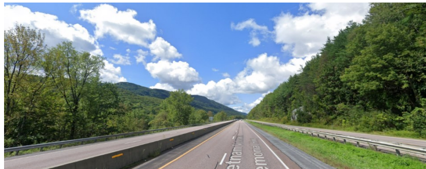
Wide Expanses of High-Speed Roadway and Concrete Median Barrier Increases the Risk of Wildlife Collisions
