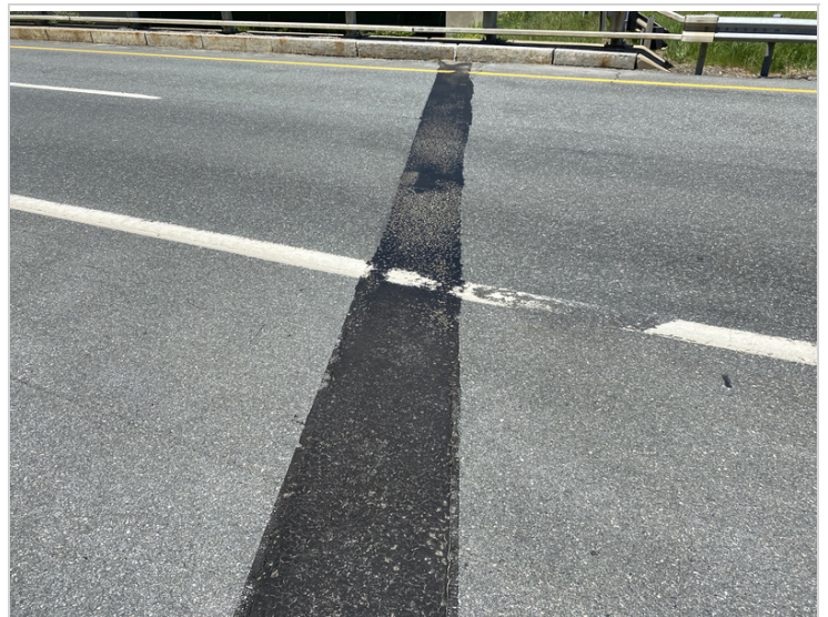
Asphaltic Plug Joint over Abutment #2
