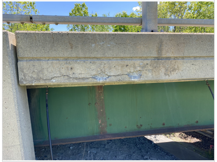
Northwest Corner Fascia
