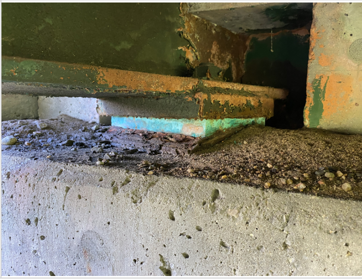
Bronze Bearing #1 at Abutment #2
