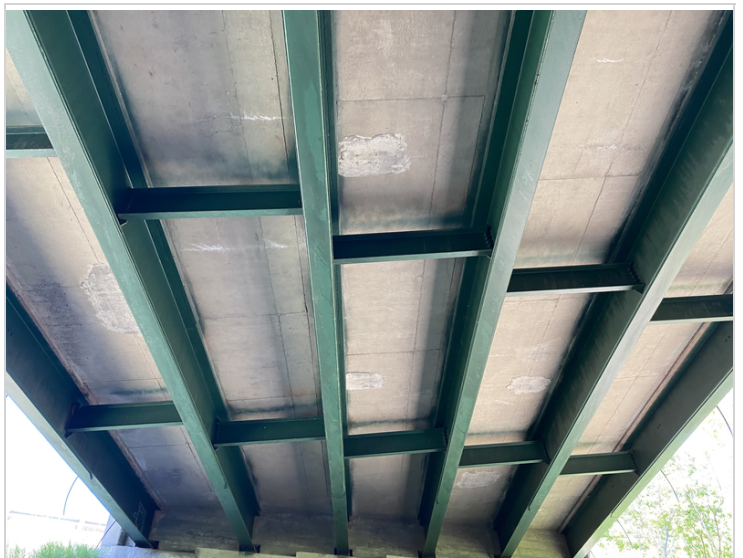
Deck Soffit Northern End
