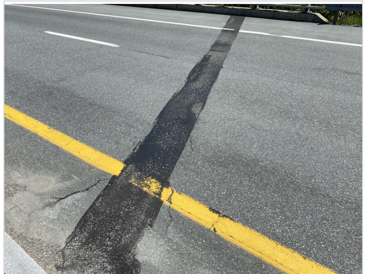
Asphaltic Plug Joint over Abutment #1
