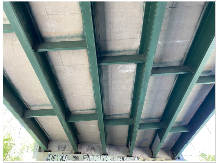
Deck Soffit Southern End
