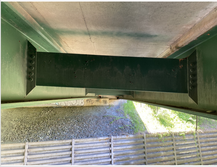
Typical Cross Bracing
