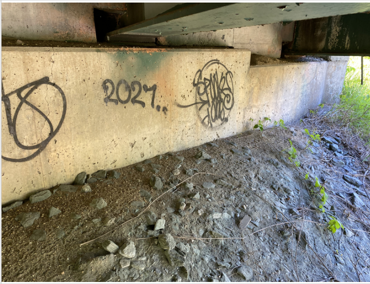
West End Abutment #1
