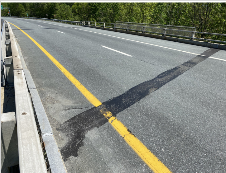
Deck Wearing Surface from Abutment #1
