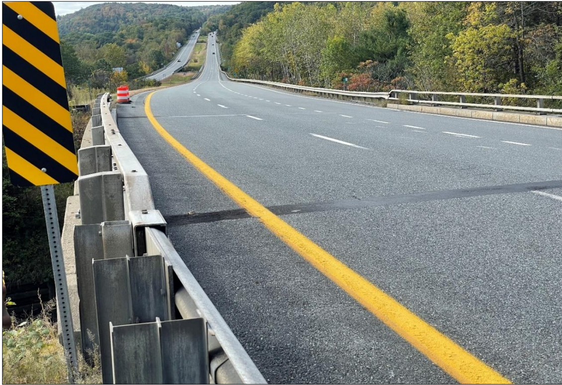
Looking South over Bridge 27S
