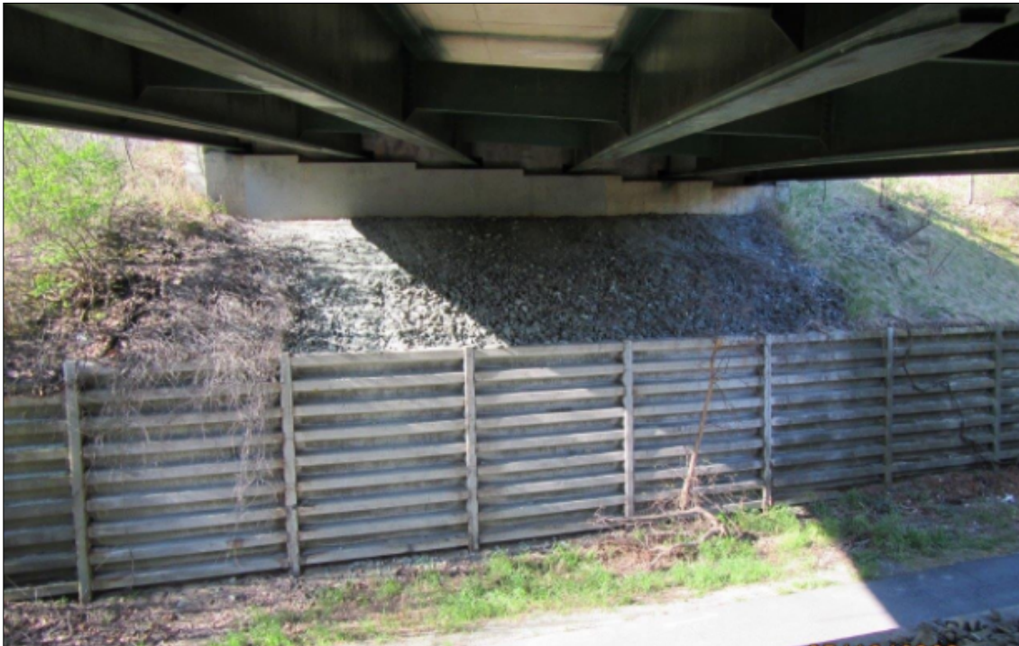
Bridge 27N Abutment and Bin Wall
