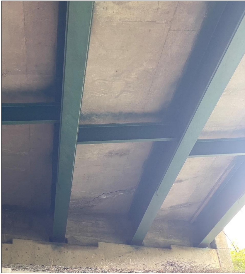
Bridge 27S Deck Underside at Abutment
