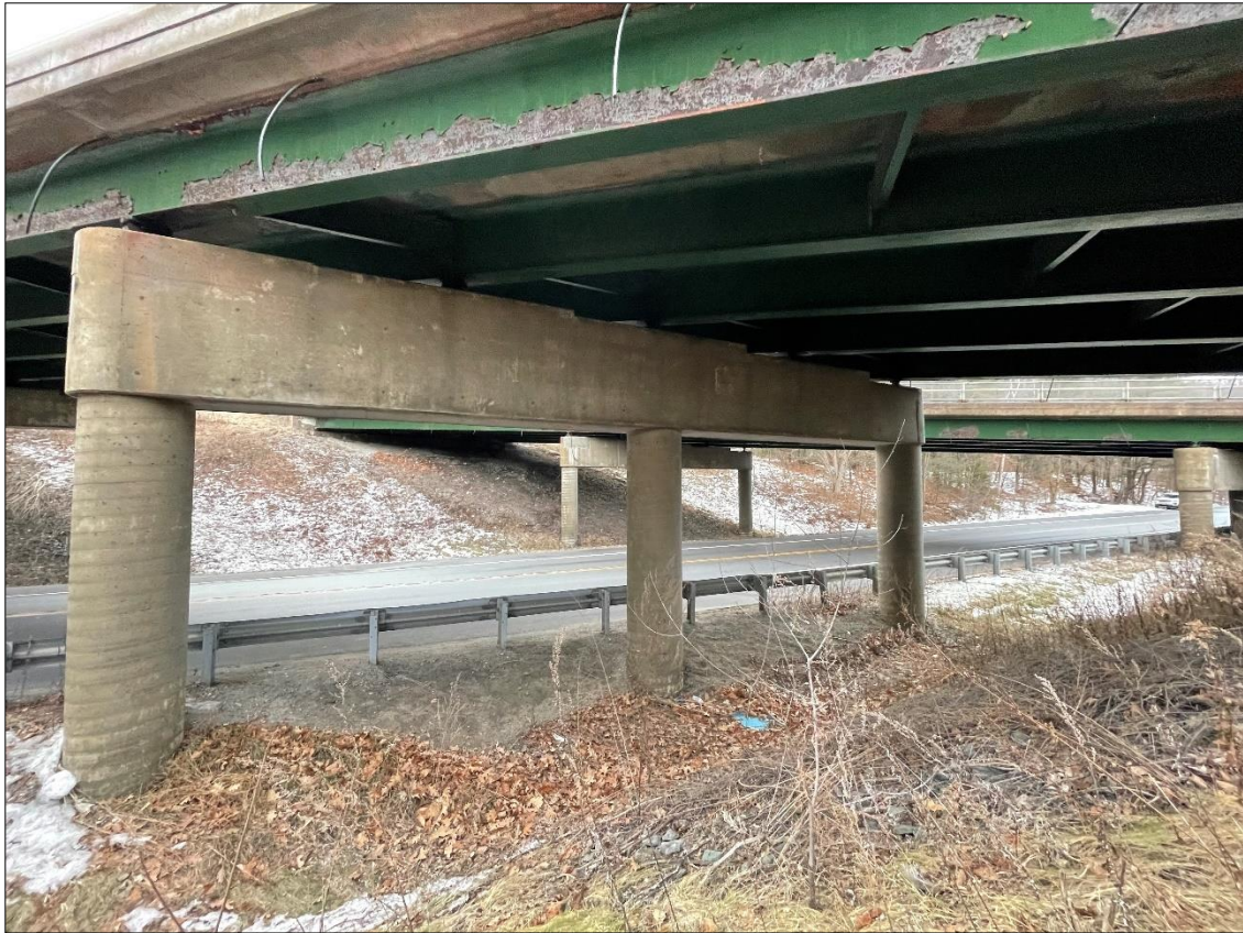
Bridge 25N Southern Pier
