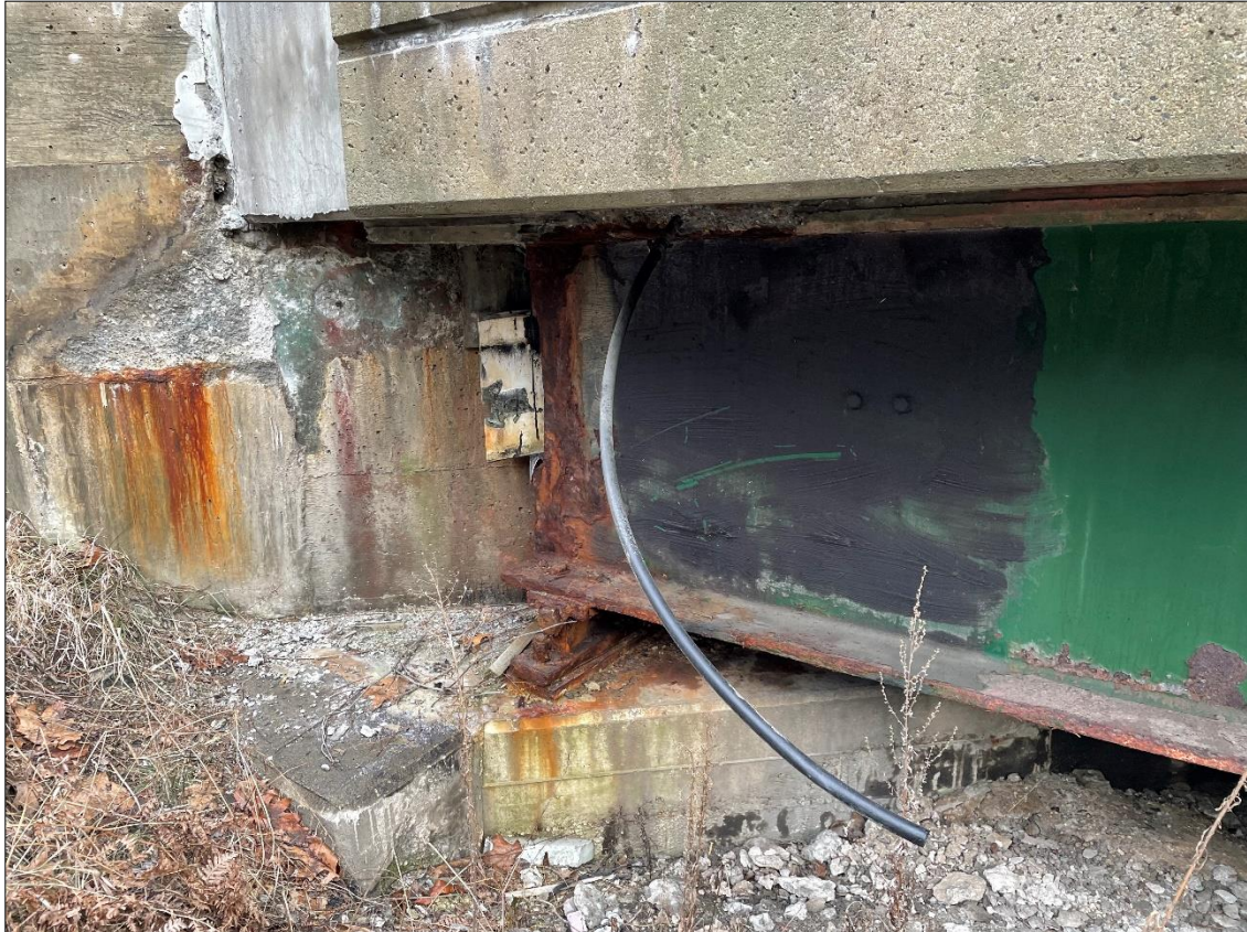
Bridge 25S Northern Abutment Western Fascia
