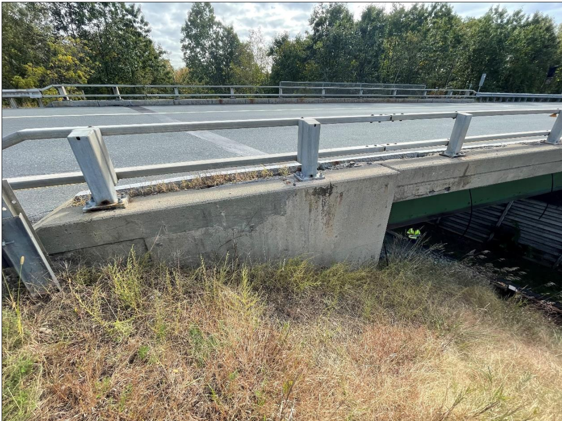
Bridge 27N Wingwall and Deck End
