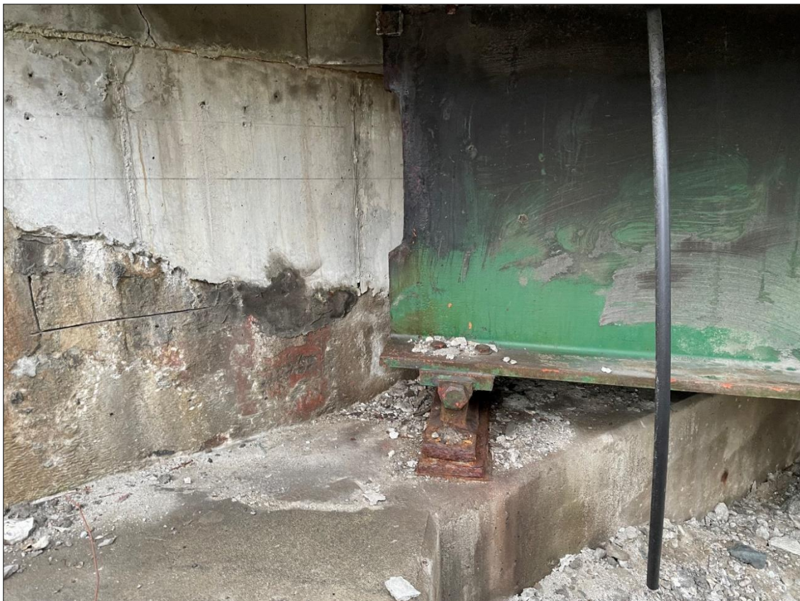
Bridge 25N, Northern Abutment Eastern Fascia
