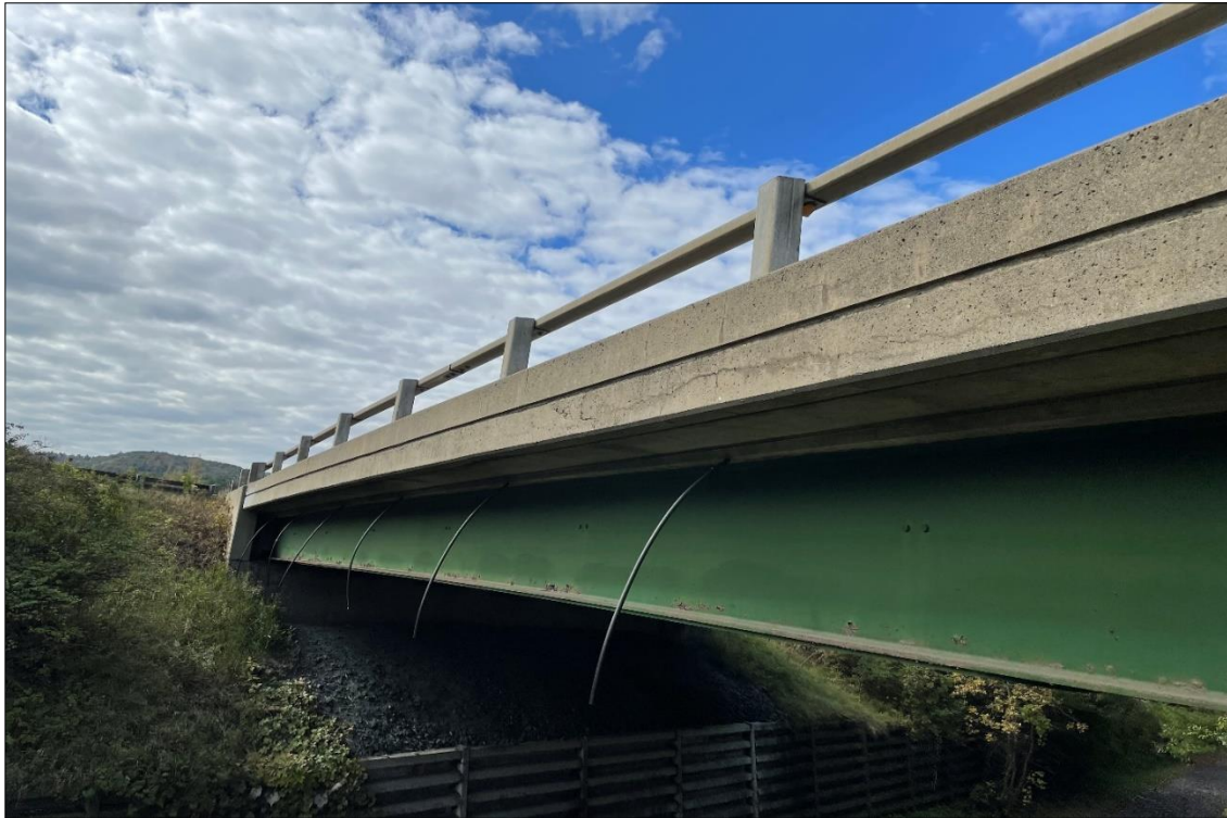
Bridge 27S Median Fascia
