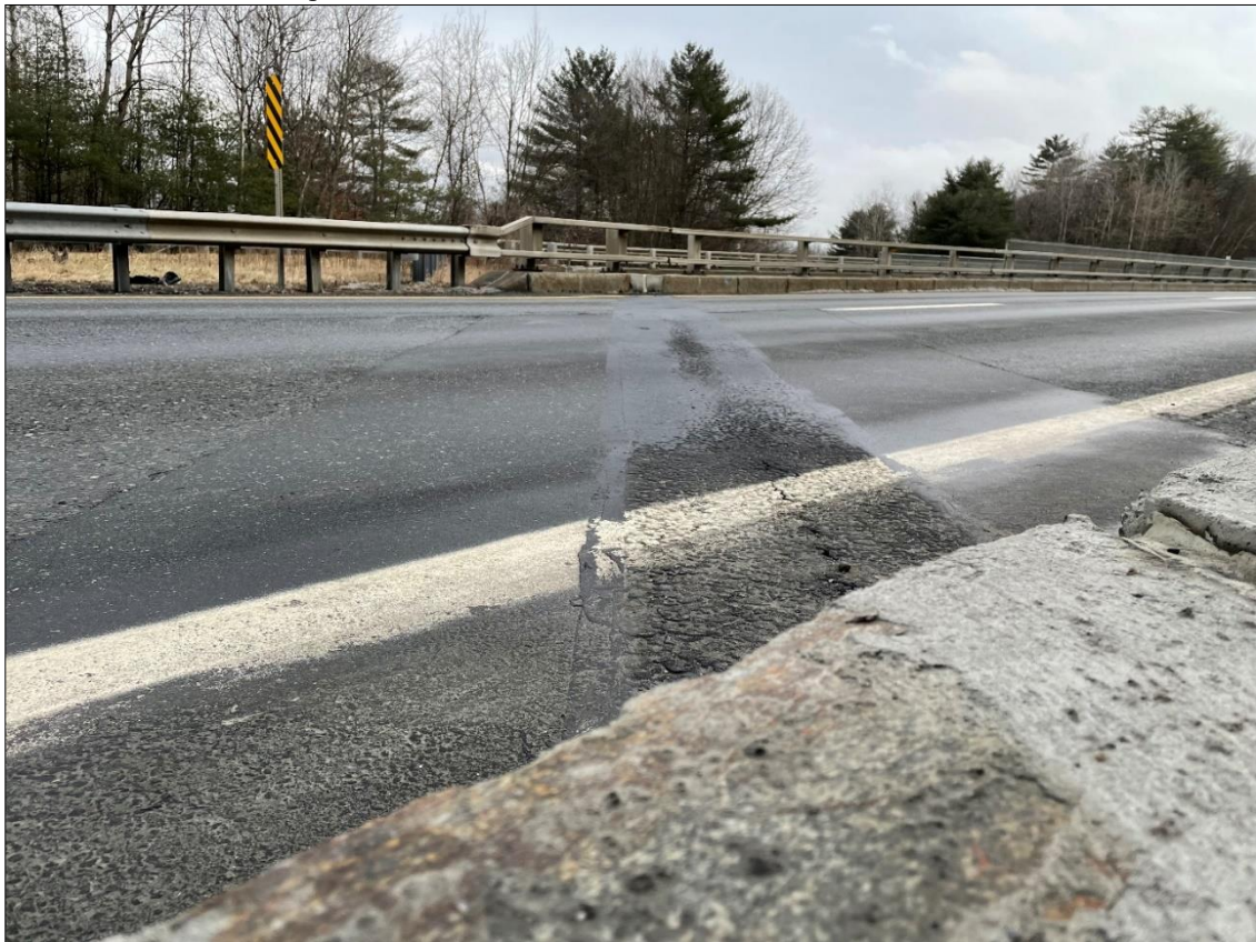
Bridge 25S Northern Deck Joint
