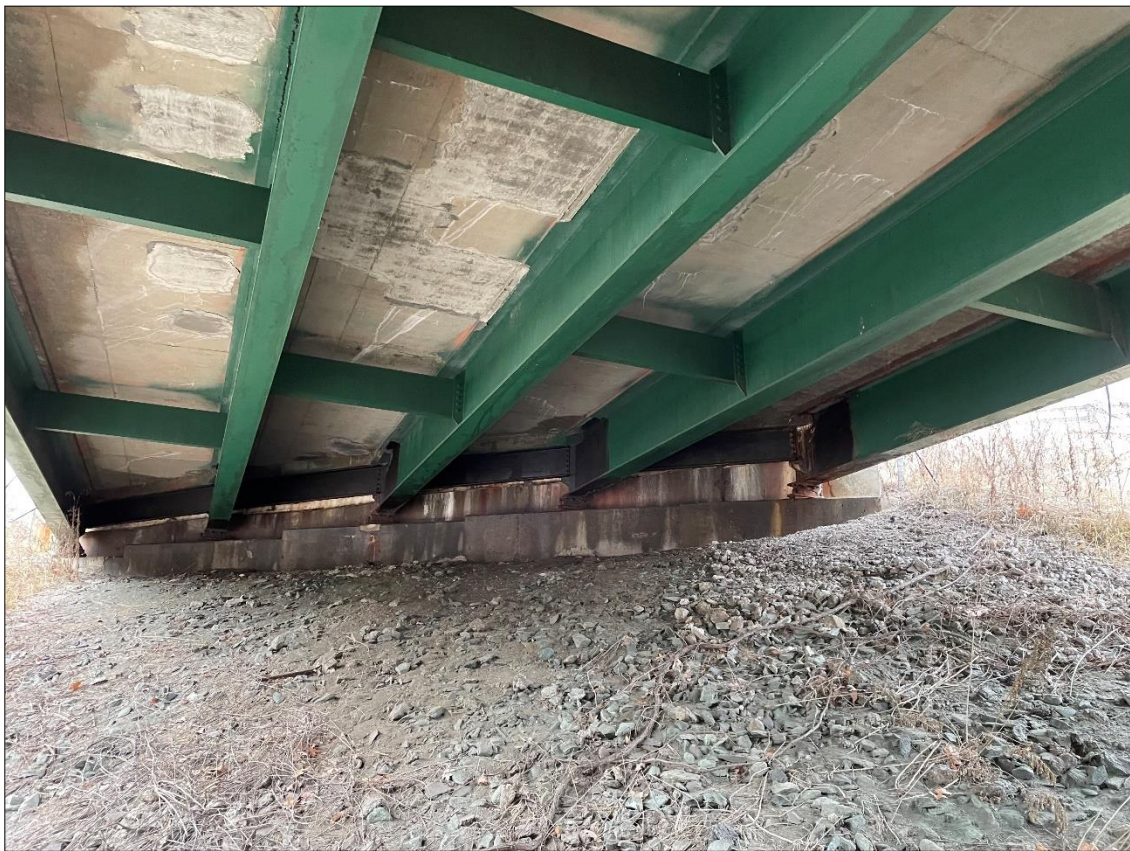
Bridge 25S Deck underside at Northern End
