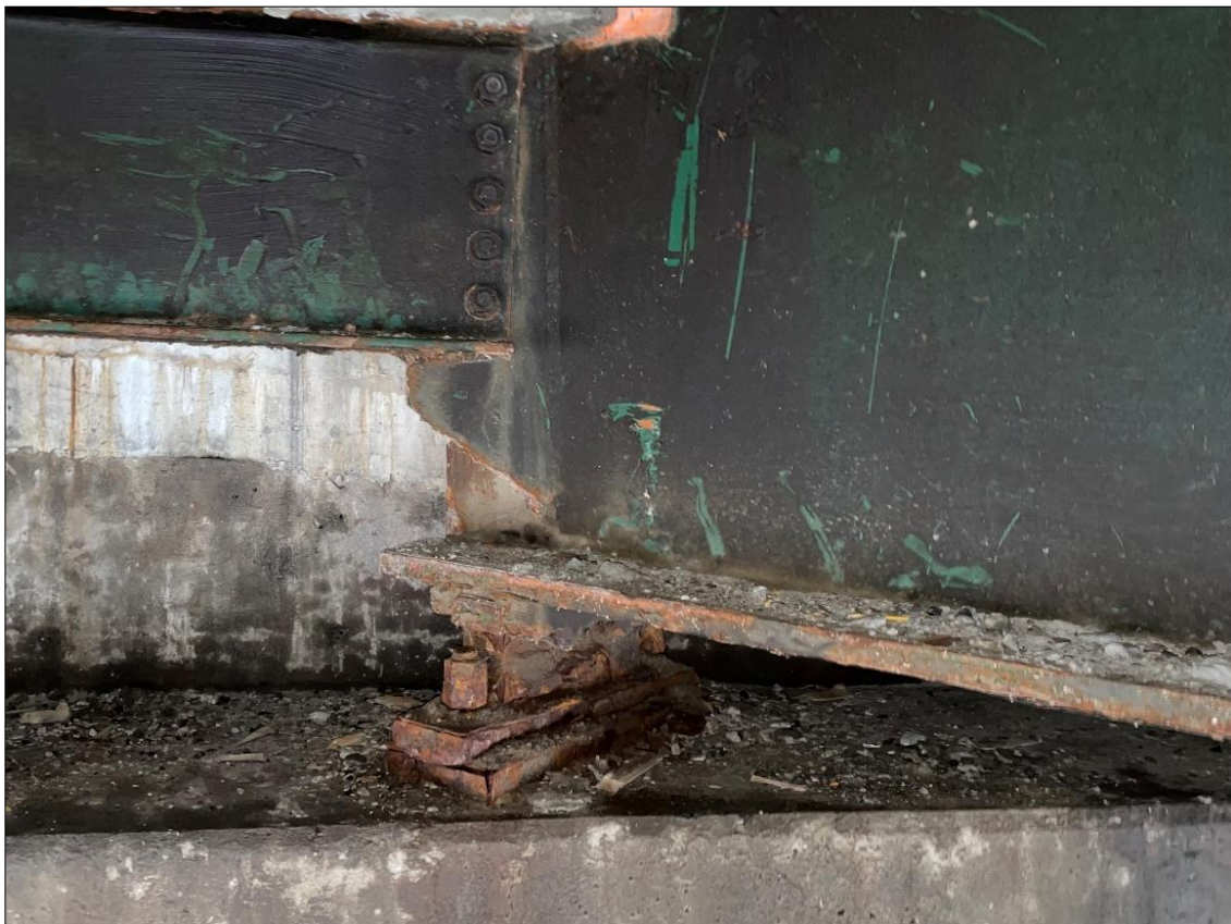
Bridge 25S Southern Abutment Typical Bearing Condition
