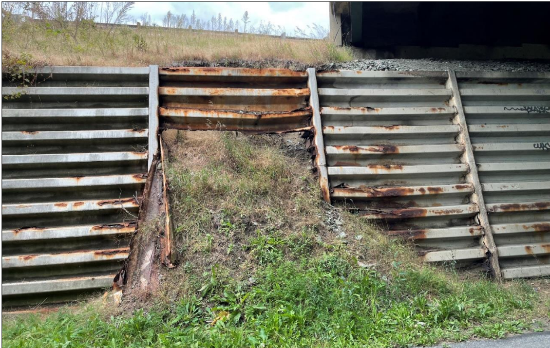
Northern Bin Wall Under 26N Median Fascia
