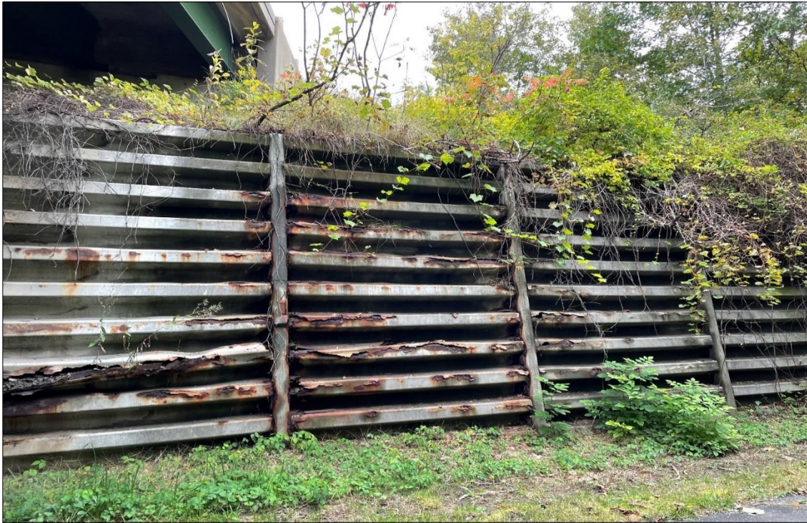
Northern Bin Wall Under 26S Median Fascia
