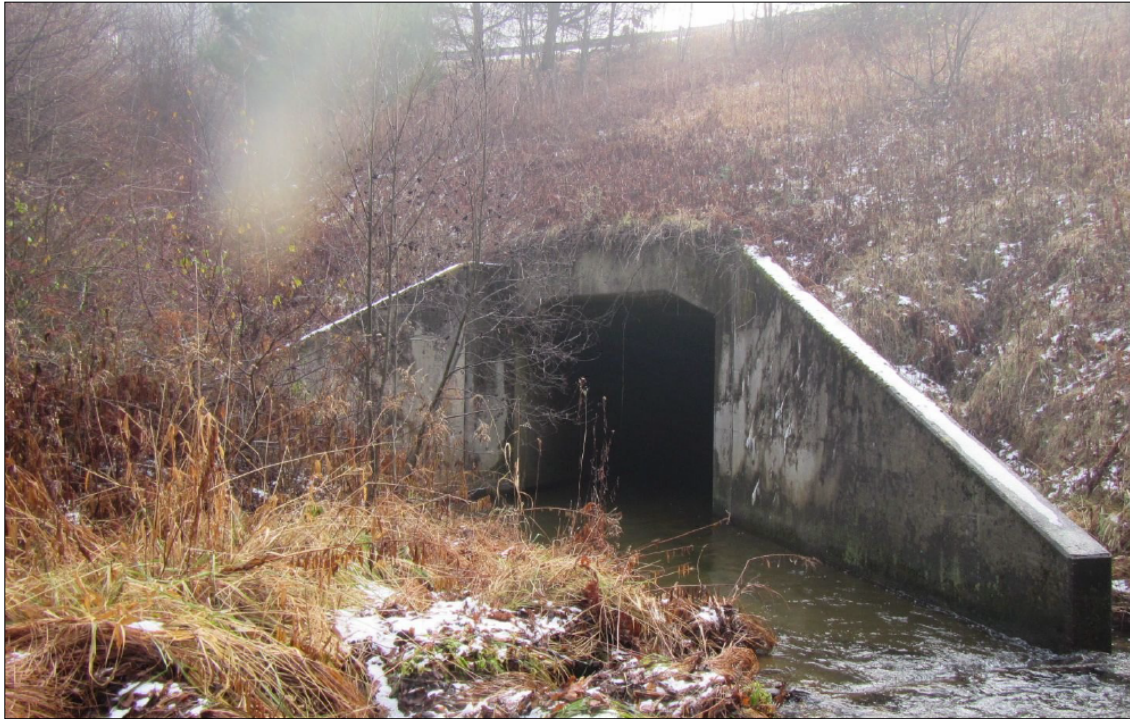
Spencer Brook Culvert un Exit 7 Ramp
