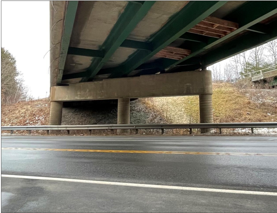
Bridge 25S Southern Pier
