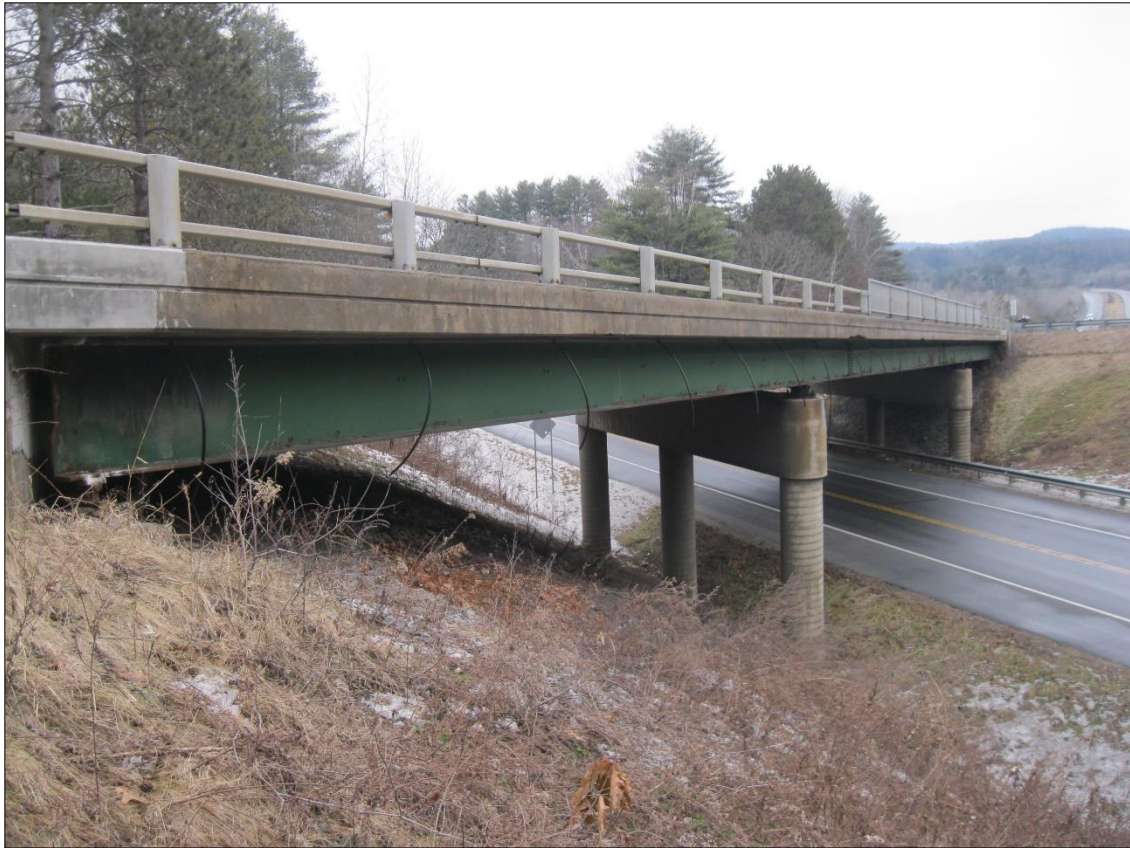
Bridge 25S Median Fascia
