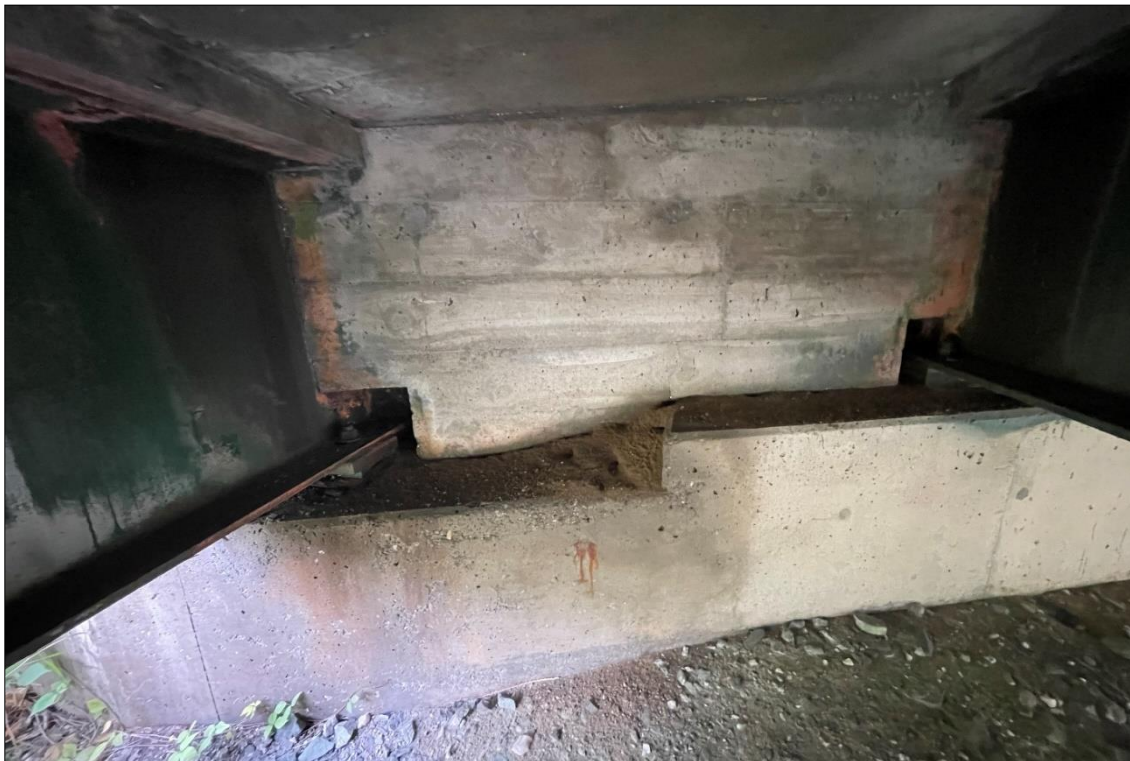
Bridge 27S Abutment Backwall and Seat
