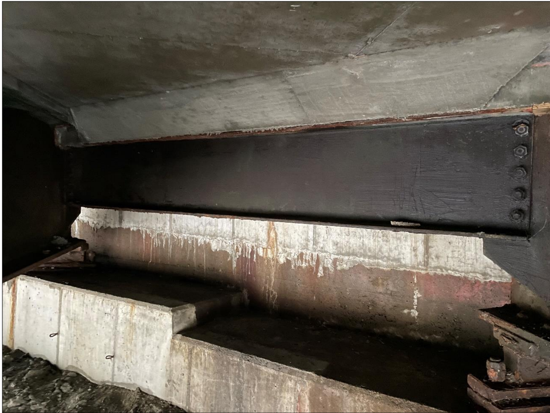
Bridge 25N, Northern Abutment Backwall and Seat
