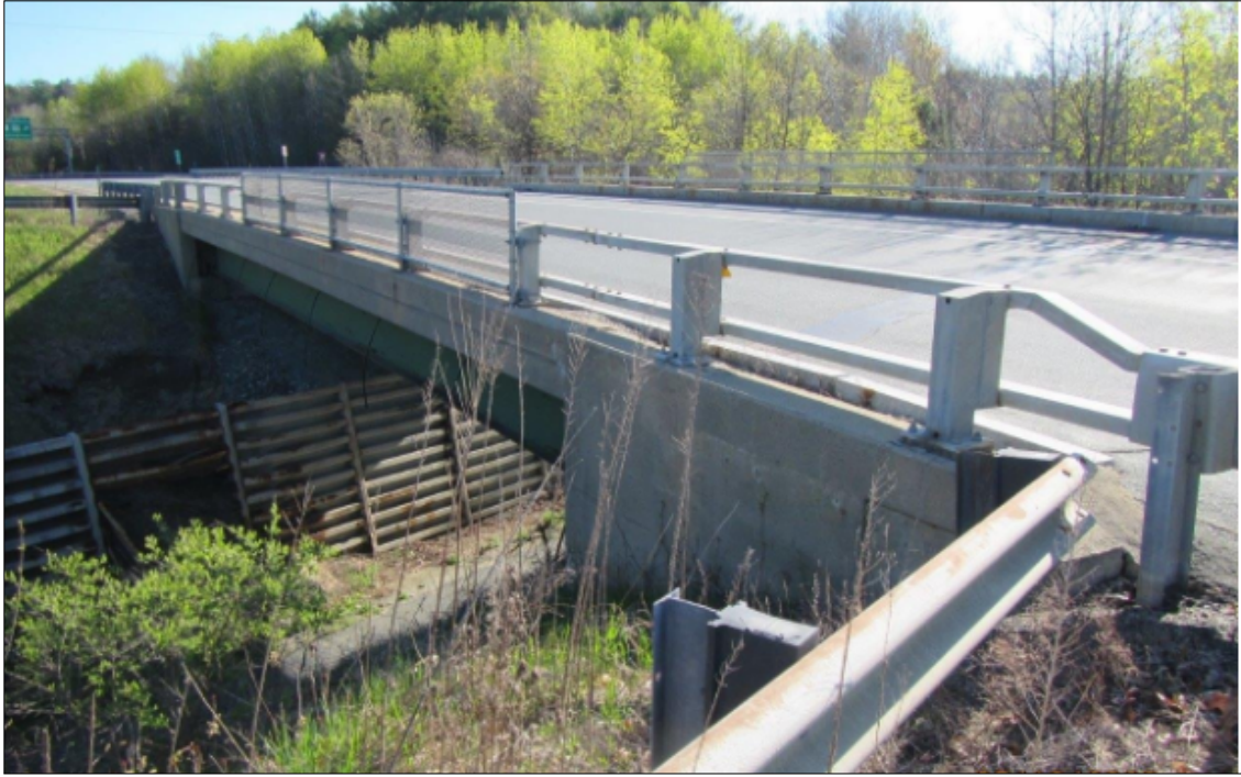
Bridge 27N Median Fascia
