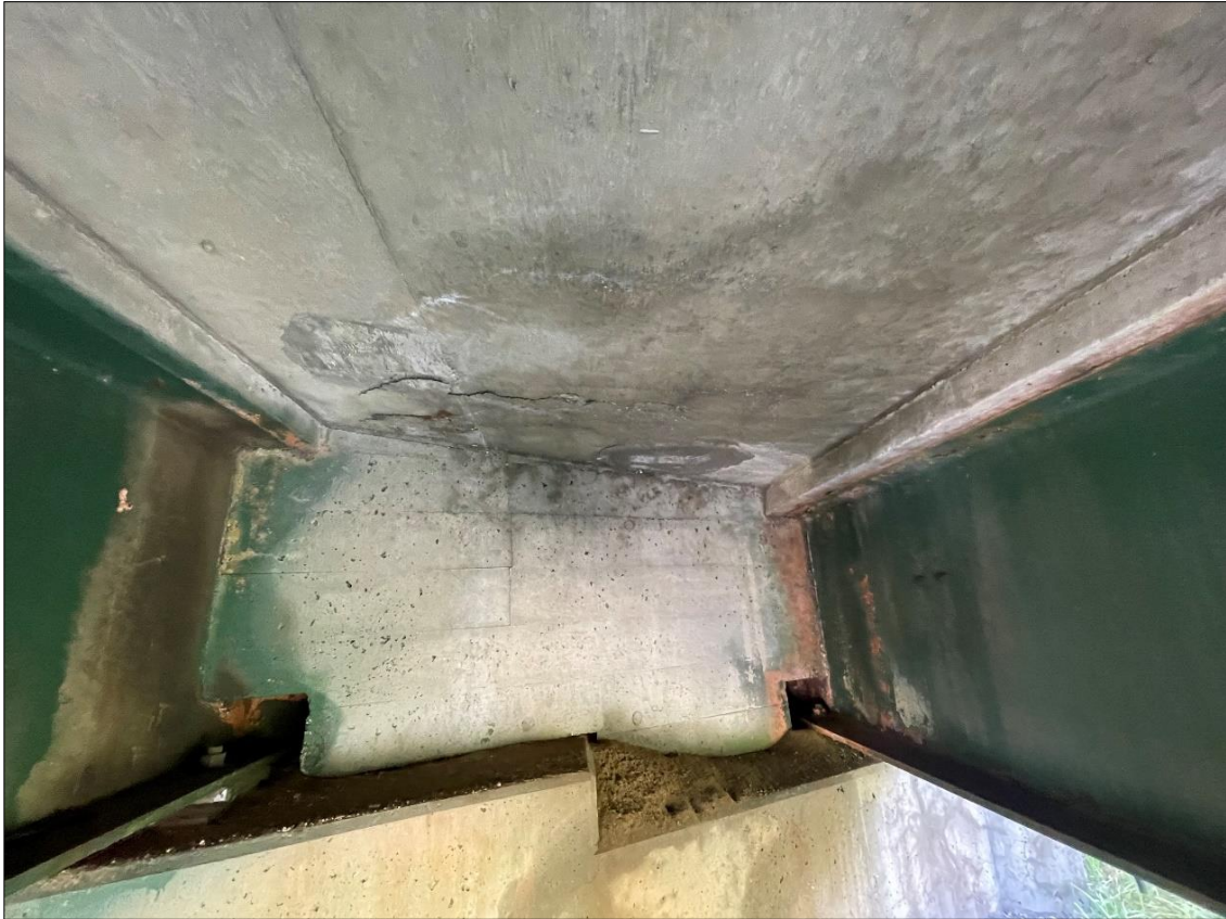
Bridge 27N Abutment Backwall and Seat
