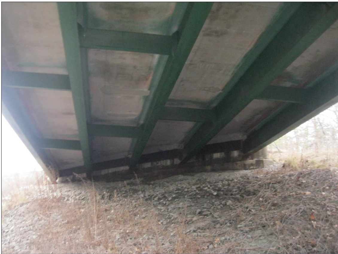
Bridge 25N Deck Underside at Northern Abutment
