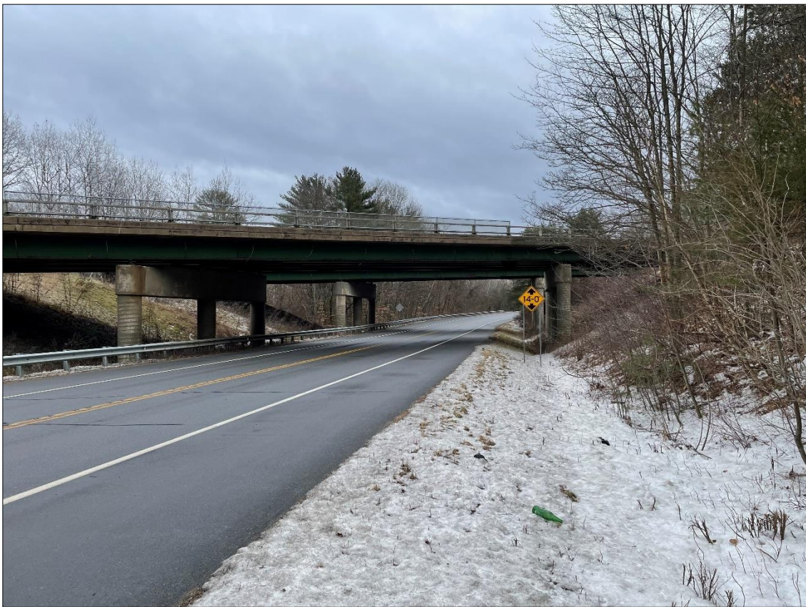
Bridge 25S from Route 5 Looking East
