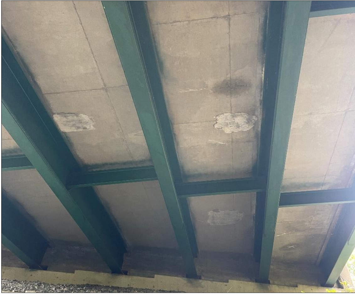
Bridge 27N Deck Underside at Abutment
