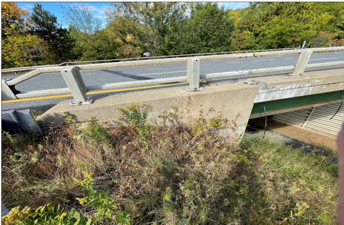
Bridge 27S Median Wingwall and Curb End
