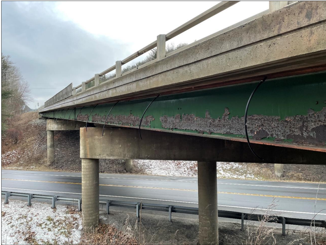
Bridge 25N Eastern Fascia
