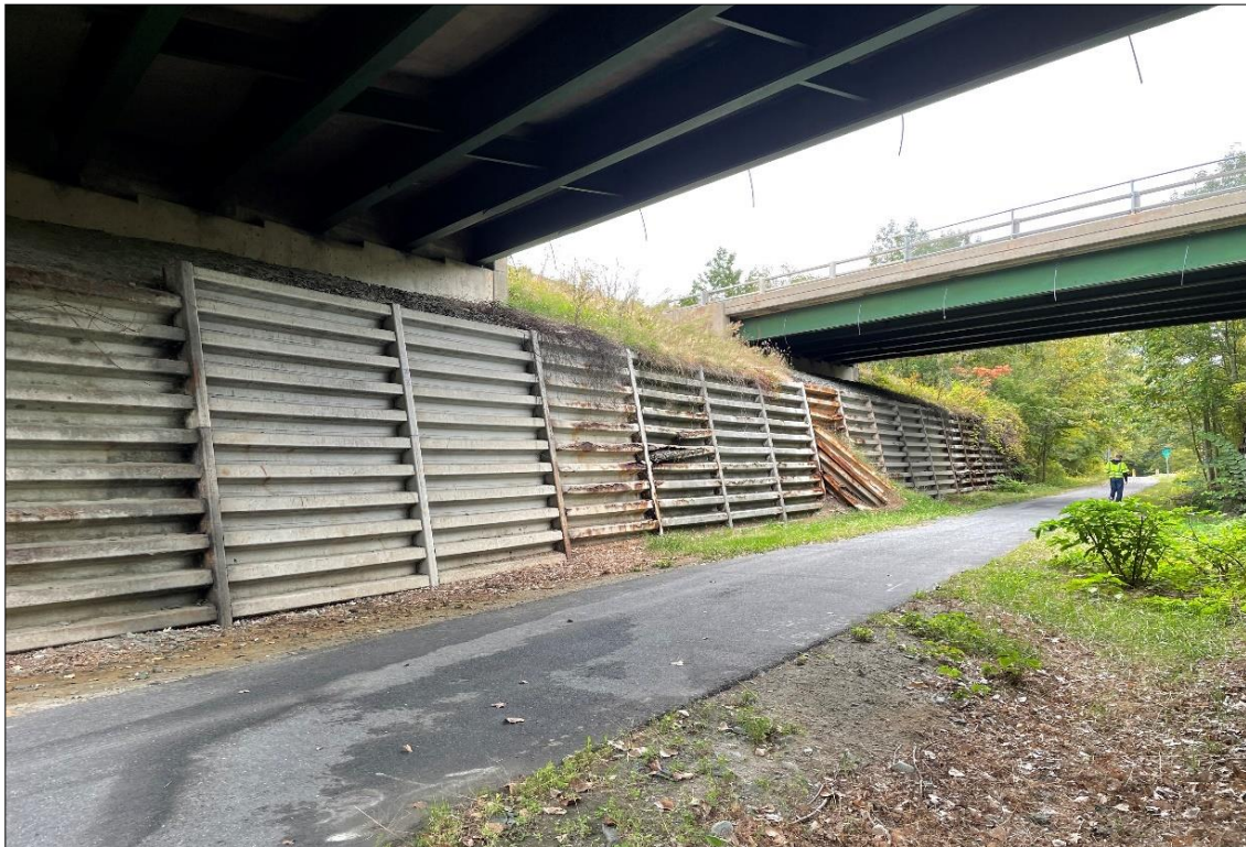
Northern Bin Wall
