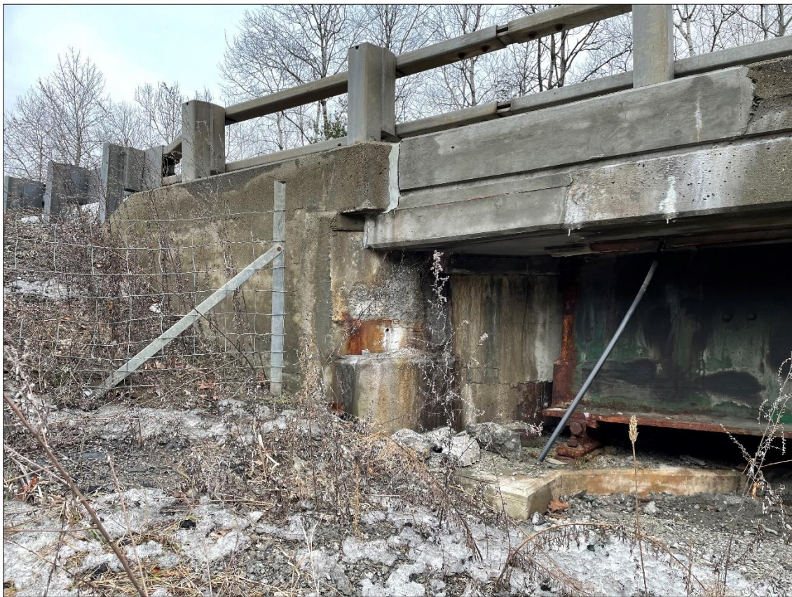
Bridge 25N Northern Abutment Western Fascia
