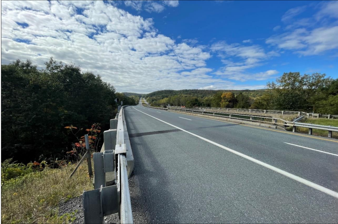
Looking north over Bridge 27N
