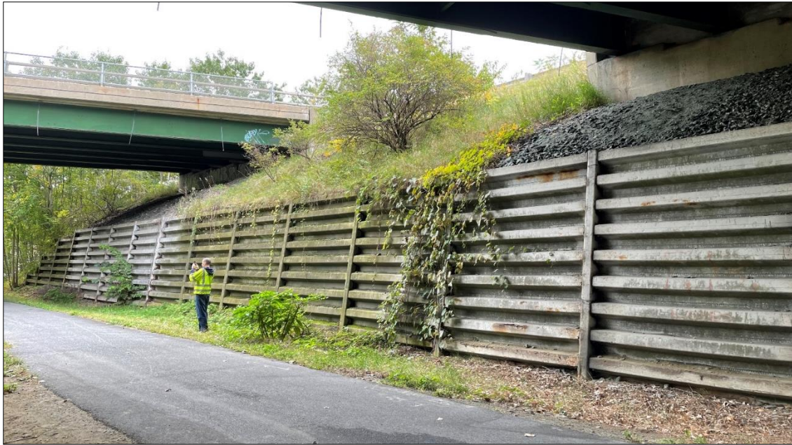
Southern Bin Wall
