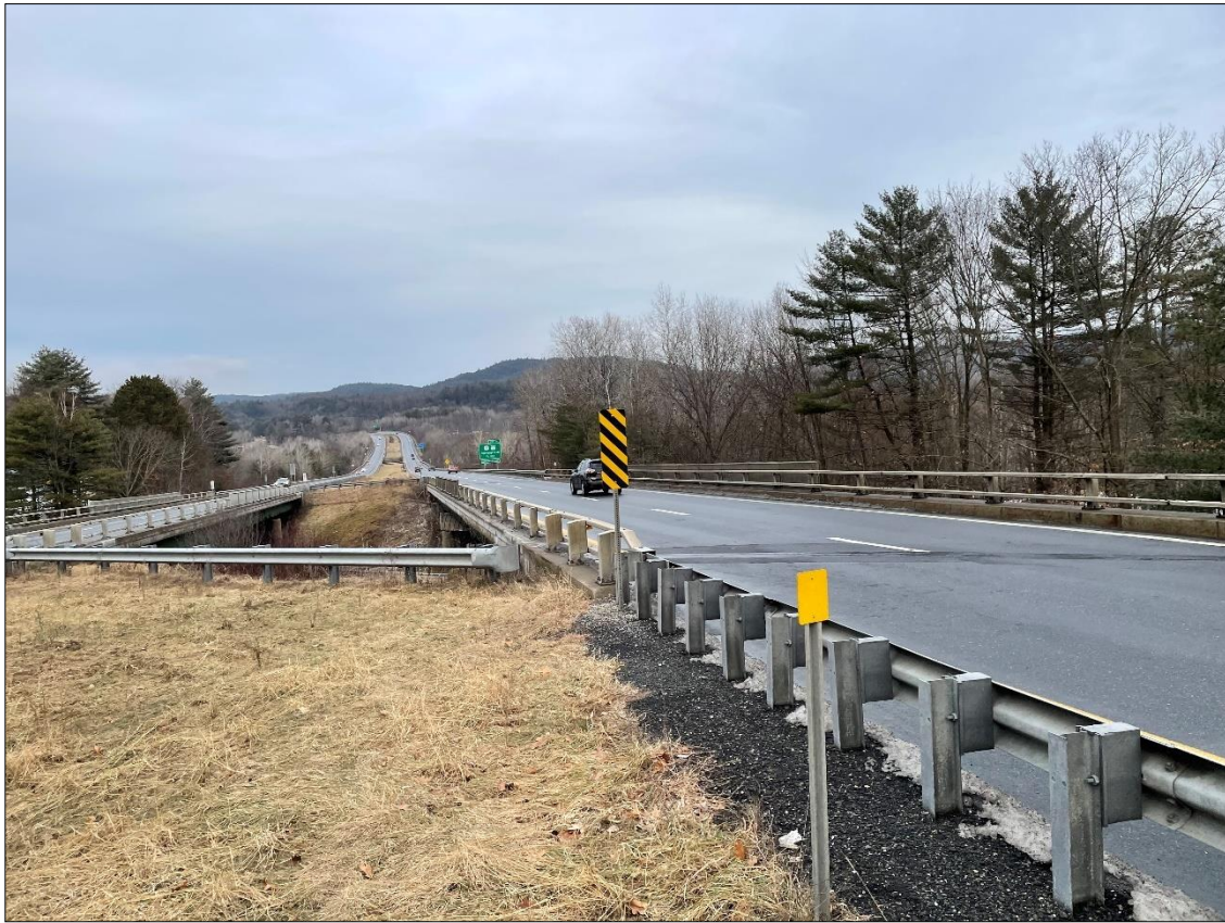
Looking South over Bridge 25N
