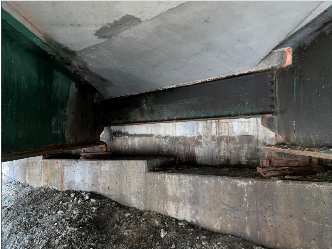
Bridge 25S Southern Abutment and Bridge Seat
