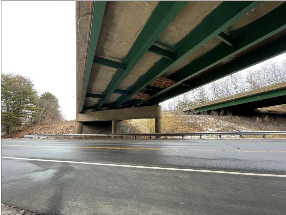
Bridge 25S Deck Underside at Midspan
