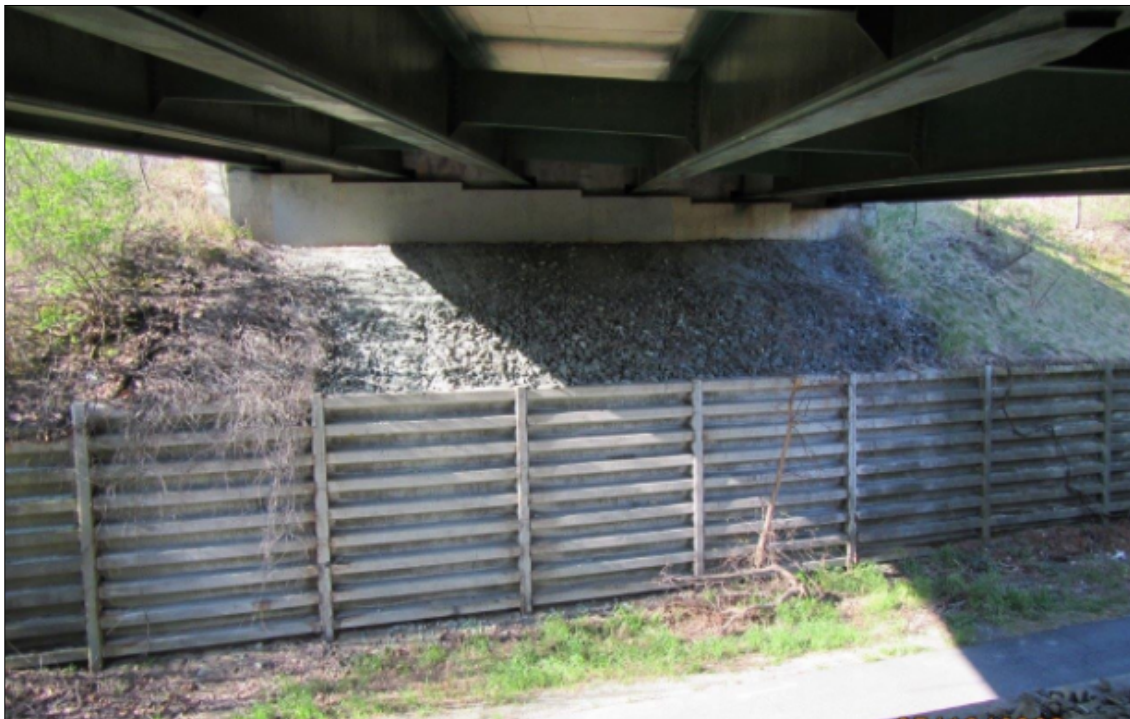
Bridge 27S Abutment and Bin Wall
