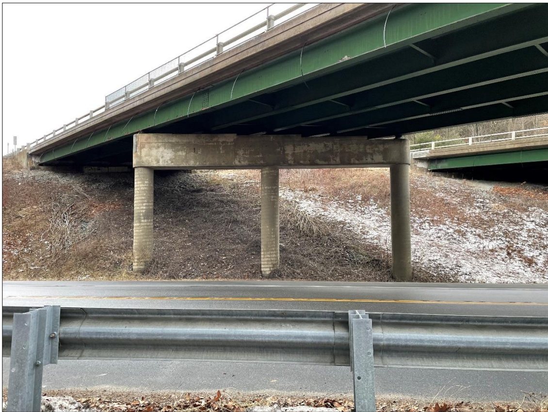
Bridge 25N Northern Pier
