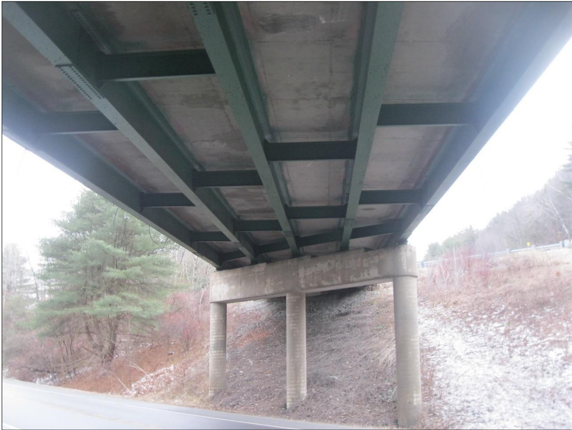
Bridge 25N Deck Underside at Midspan
