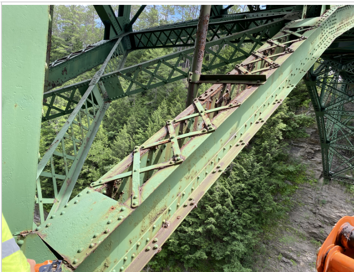
Downstream Bottom Chord between Verticals #2 and #3
