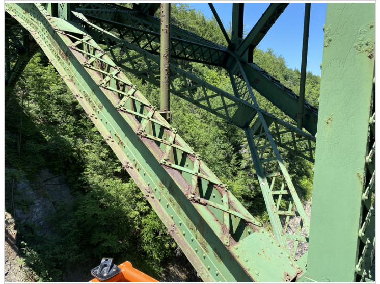
Bottom Chord between Vertical #8 and #9 Downstream
