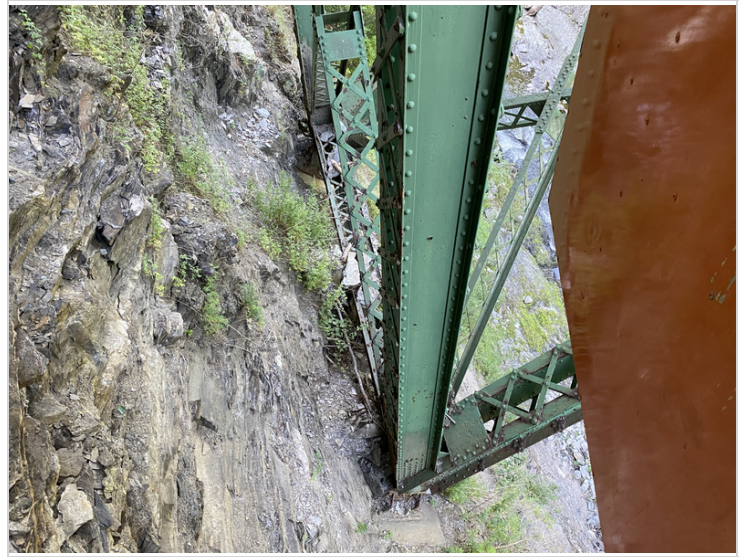
Bearings / Vertical #10 Both Upstream and Downstream
