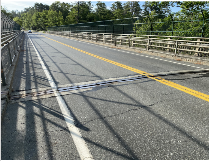
Deck Wearing Surface from Abutment #1 End
