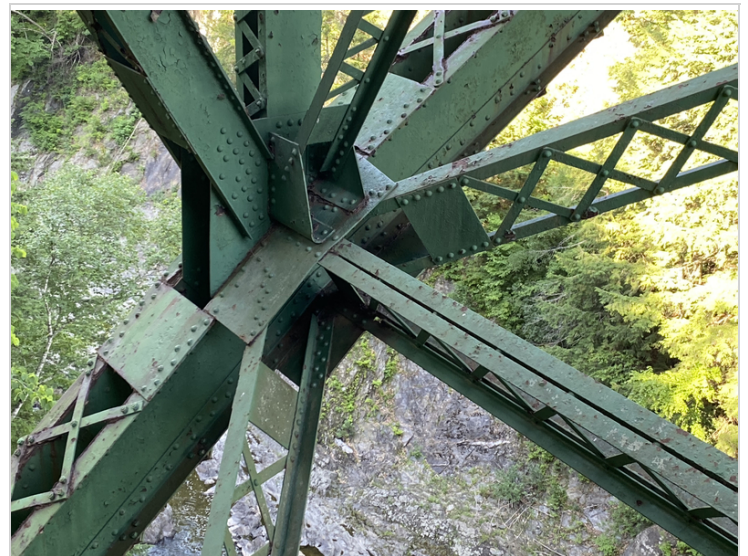
Downstream Gusset at Vertical #9
