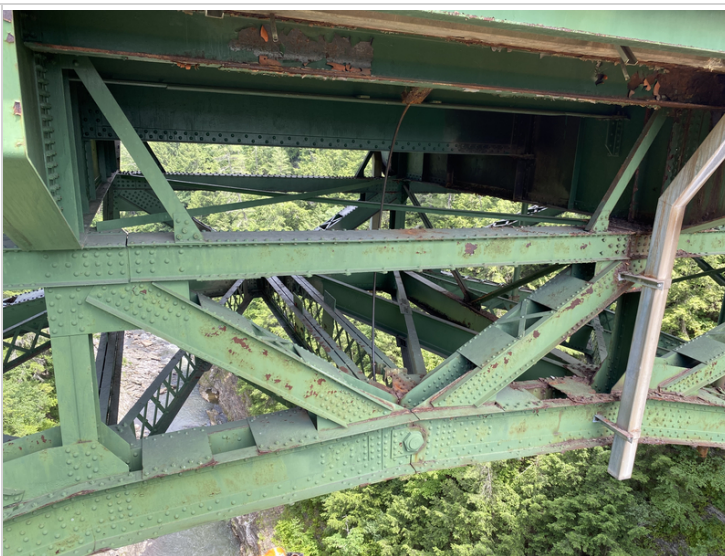
Downstream Center of Arch between Verticals #5 and #6
