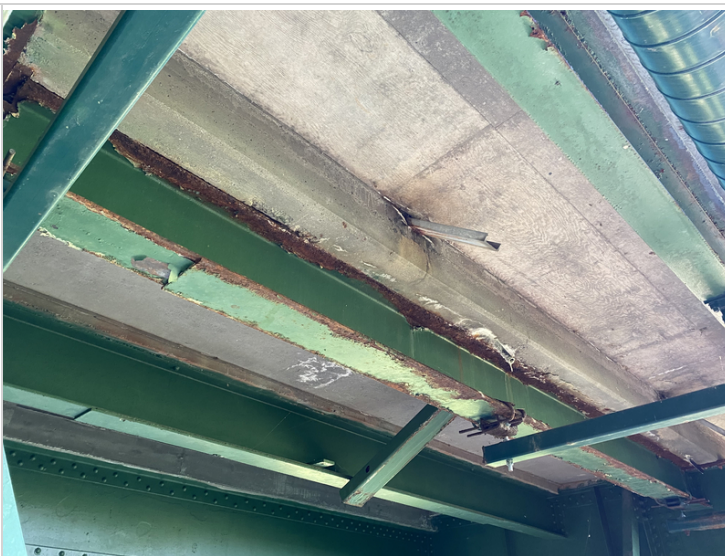
Beam #2 Between Floor Beams #8 and #9
