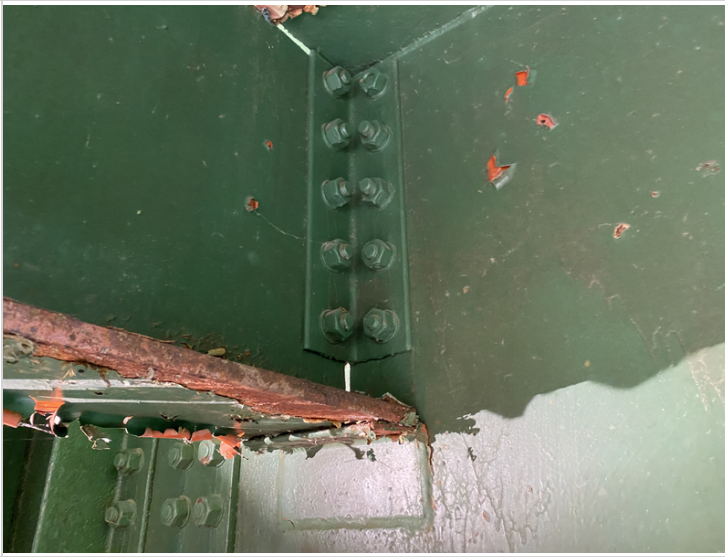
Beam #2 at Floor Beam #10 East Side
