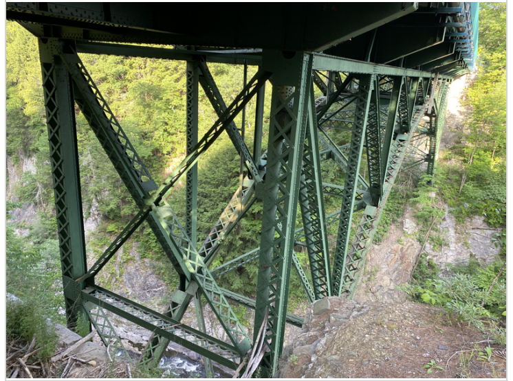
Structure from Upstream Abutment #2
