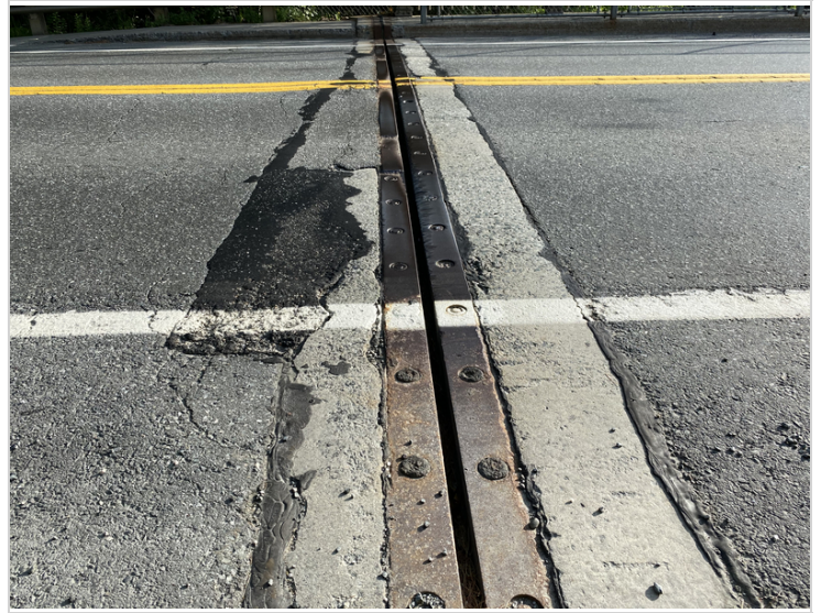
Vermont Type Joint over Abutment #1
