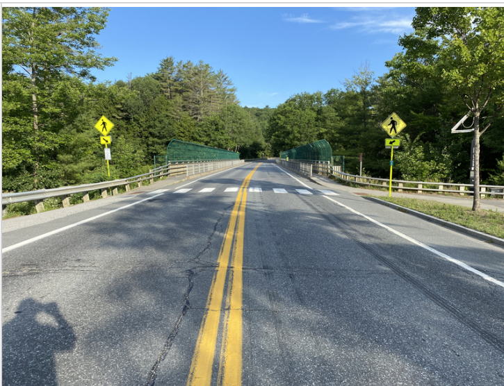
Abutment #2 Approach (Eastern)
