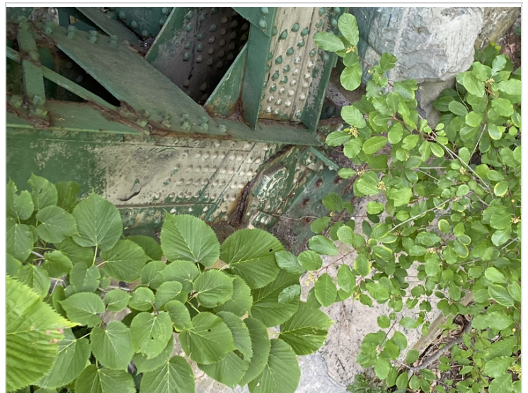
Upstream Bearing at Vertical #1
