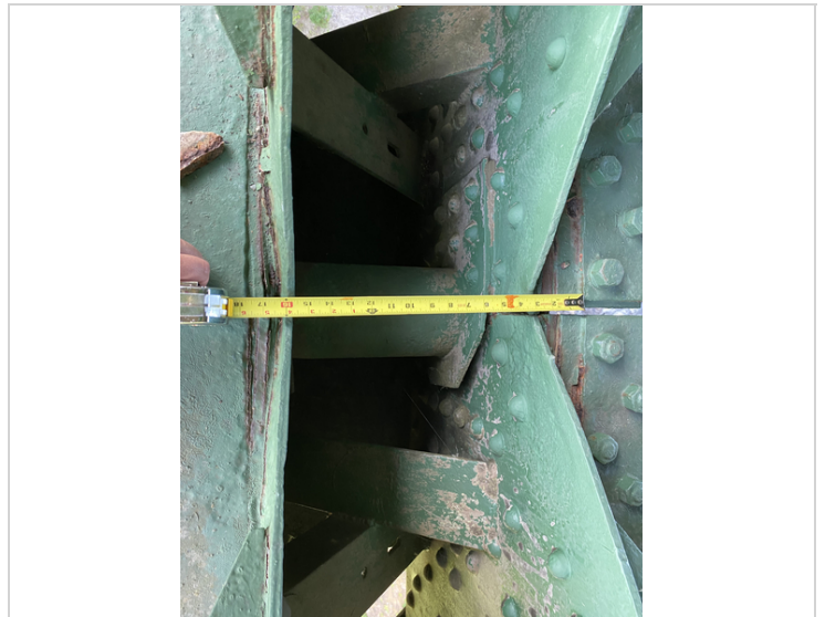
Upstream Center Pin Condition
