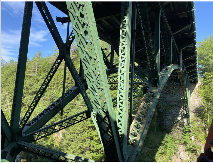
Upstream Arch from Abutment #2
