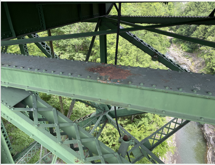
Top Chord between Vertical #3 and #4 Downstream
