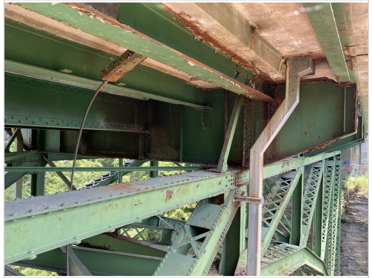
Floorbeam #6 from Downstream West Side
