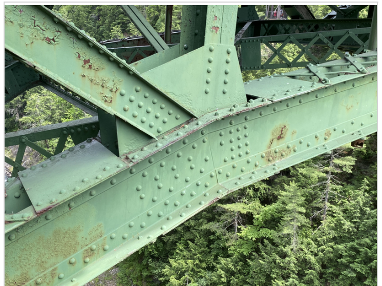
Downstream Bottom Chord at Vertical #4 / Gusset Connection
