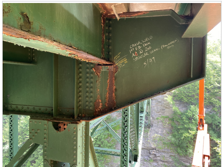
Downstream End of Floor Beam #1
