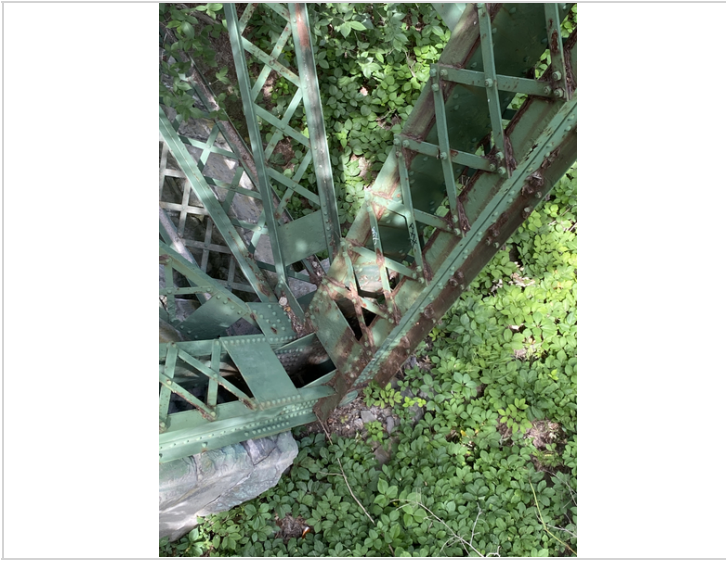
Vertical #1 Upstream / Arch Bearing
