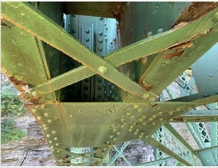
Bottom Chord at Vertical #8 Upstream
