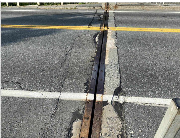
Vermont Type Joint over Abutment #2
