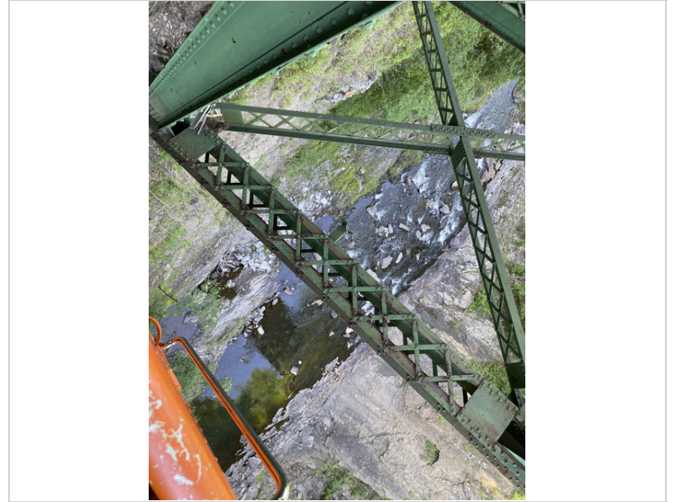
Upstream Bottom Chord between Verticals #9 and #10
