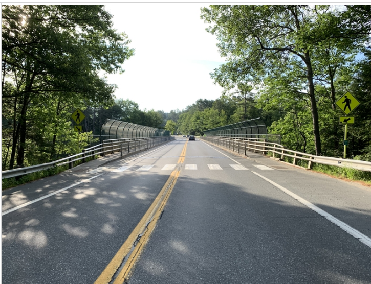
Western Approach (Abutment #1)
