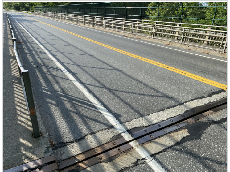
Deck Wearing Surface from Upstream Abutment #1
