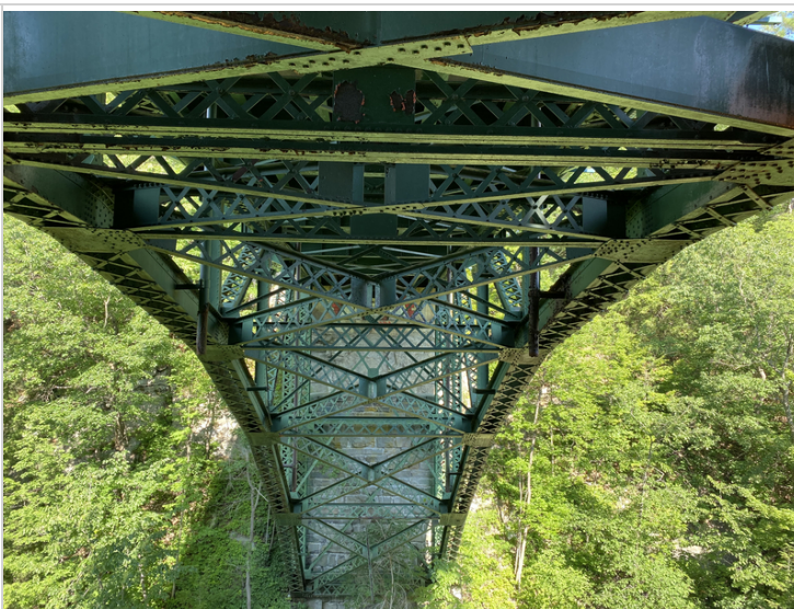
Lower Section of Truss towards Abutment #1
