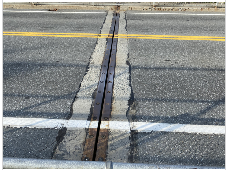
Vermont Type Joint over Center
