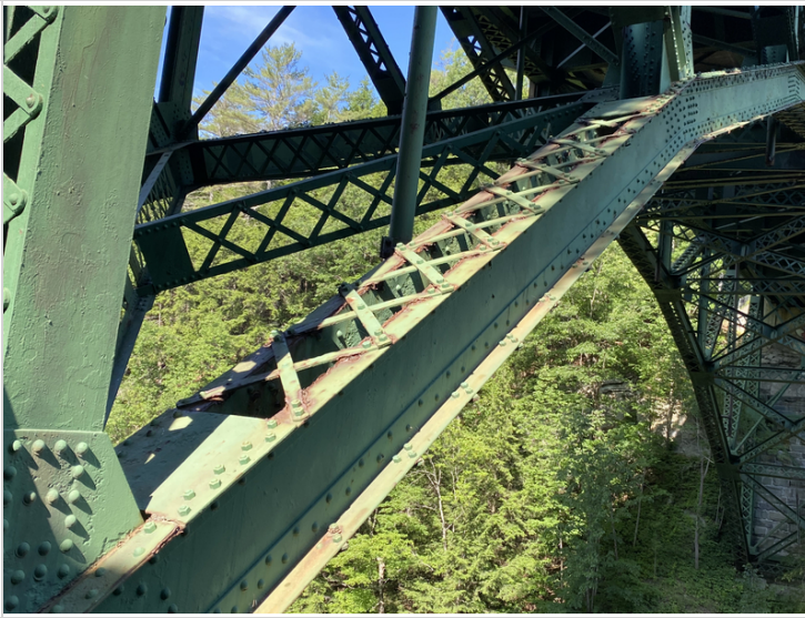
Bottom Chord Upstream between Verticals #8 and #9
