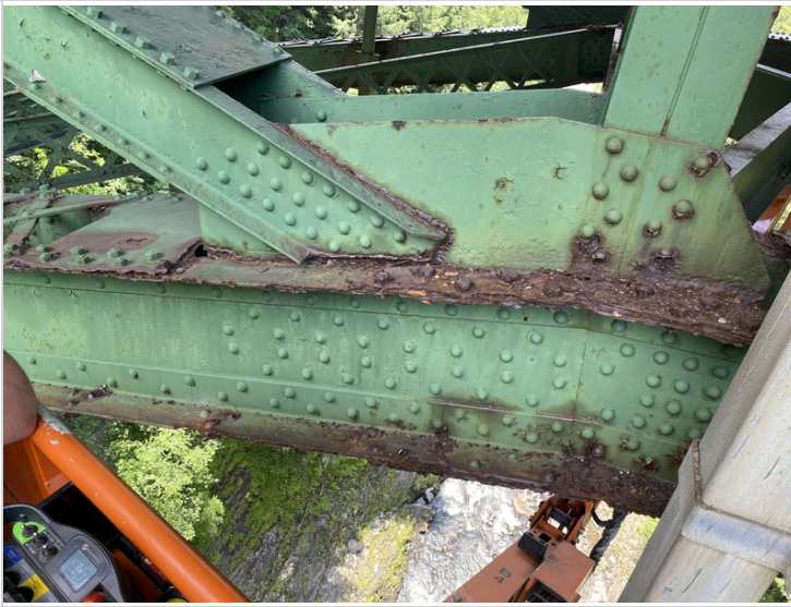
Upstream Bottom Chord / Connection at Vertical #6
