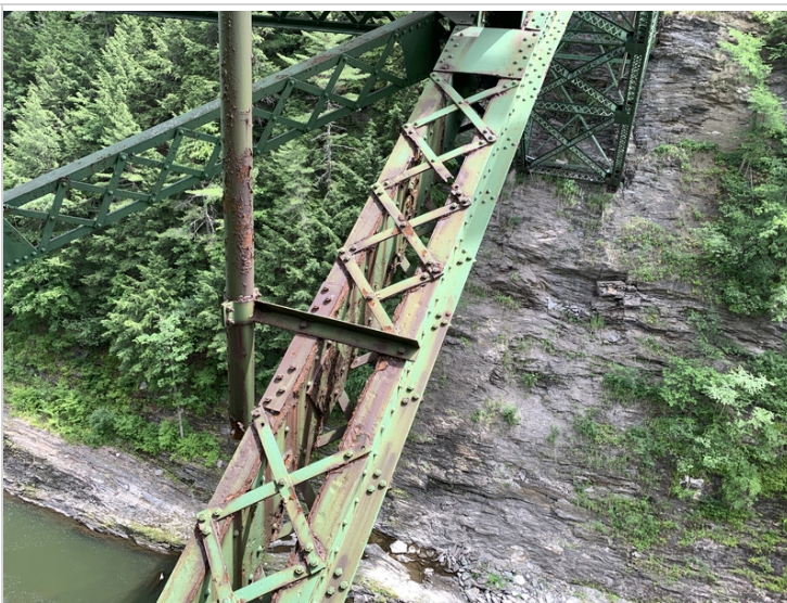
Bottom Chord along Downstream Side
