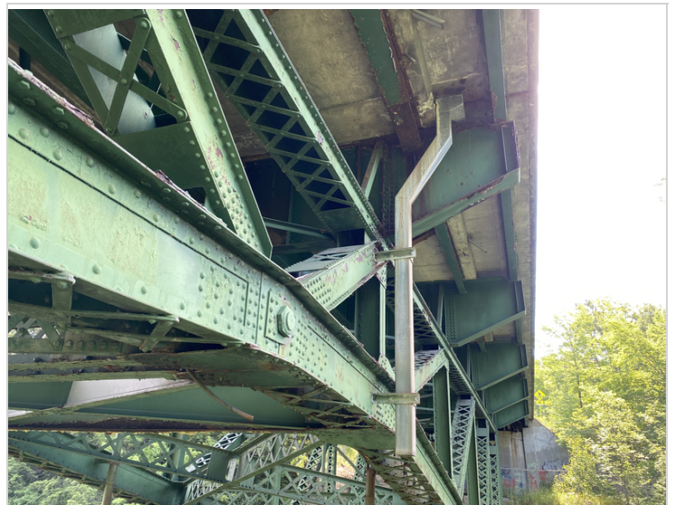
Typical Deck Drain
