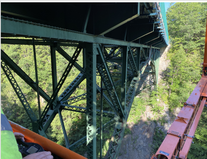
Structure from Upstream Abutment #2
