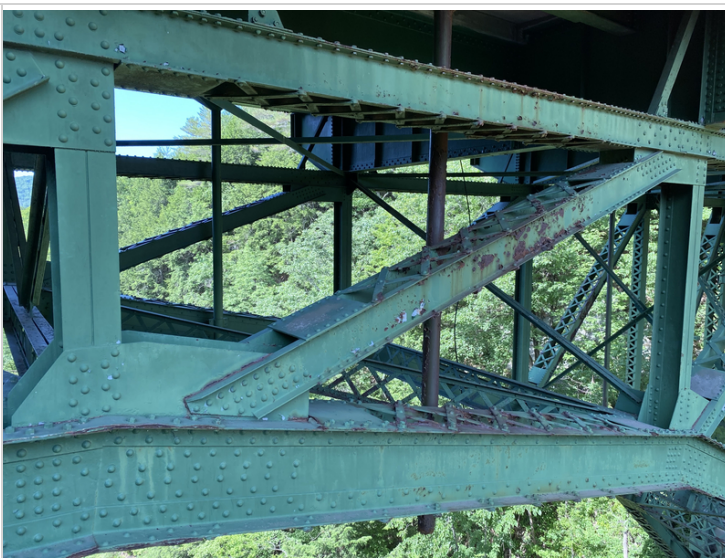
Upstream Arch Section between Floorbeams #4 and #5
