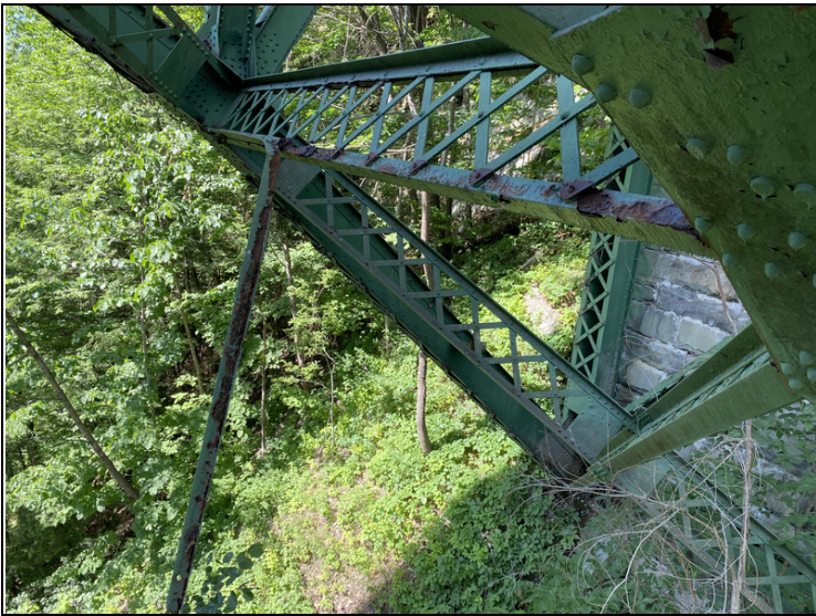
Cross Bracing between Vertical #2
