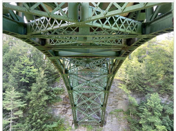
Lower Portion of Arch towards Abutment #2 End
