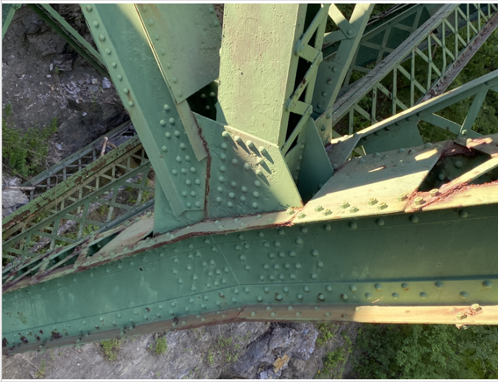
Lower Gusset at Vertical #9 Upstream
