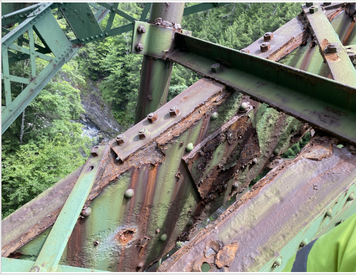
Downstream Bottom Chord between Verticals #2 and #3
