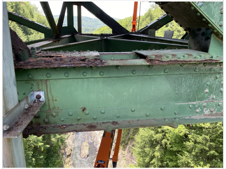
Upstream Bottom Chord between Pin and Vertical #6
