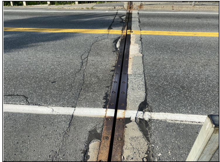
Vermont Type Joint over Abutment #2
