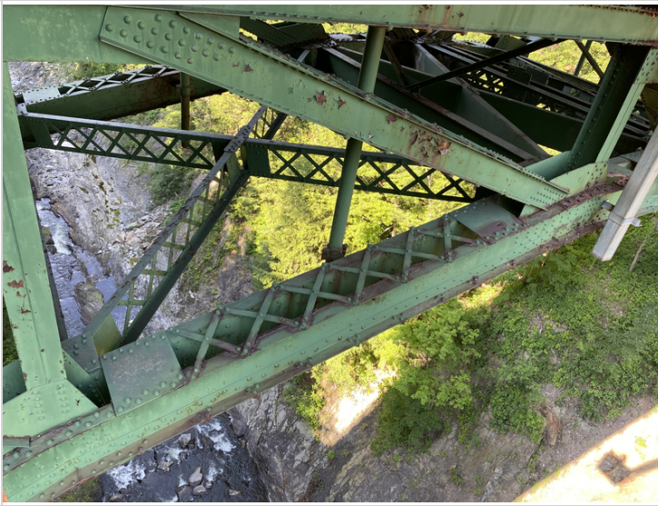
Bottom Chord between Verticals #6 and #7 Upstream
