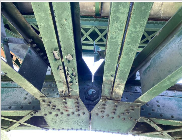
Pin at Center of Arch Upstream
