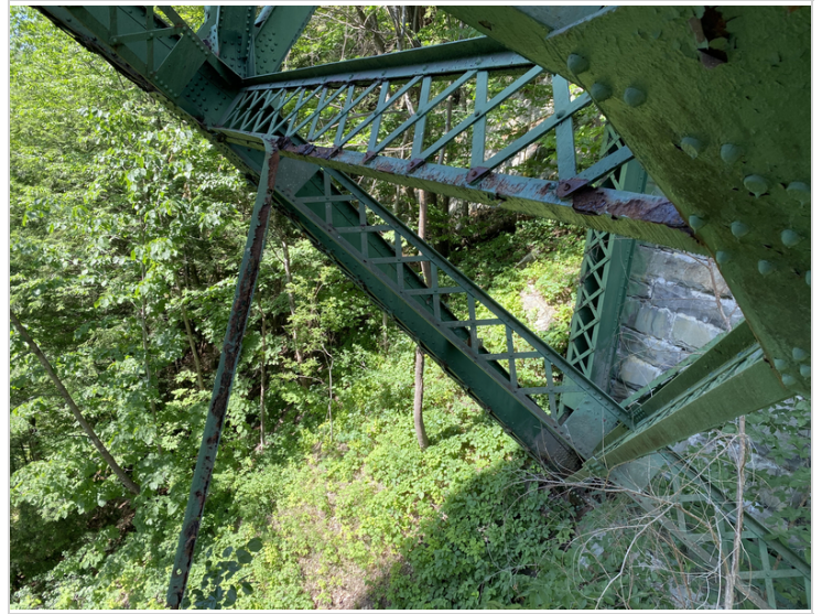
Cross Bracing between Vertical #2
