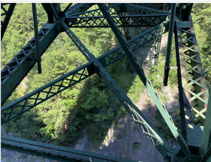
Cross Bracing between Verticals #8 and #9
