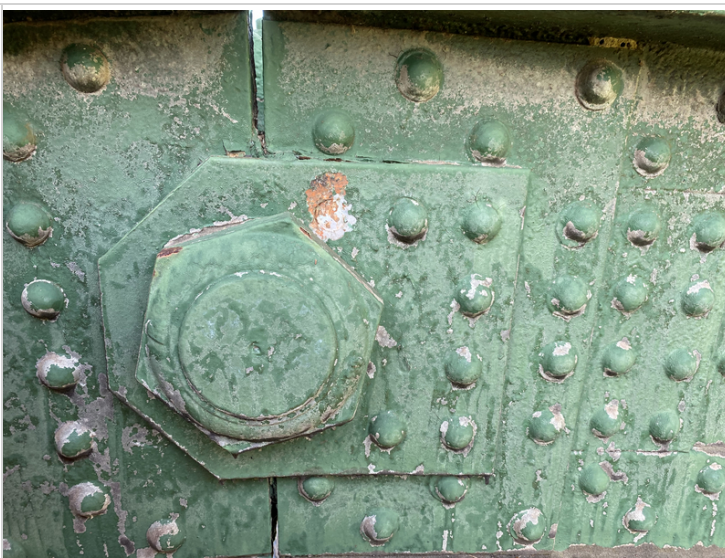
Upstream Center Pin
