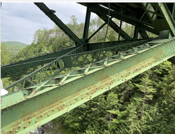
Bottom Chord between Verticals #3 and #4 Downstream
