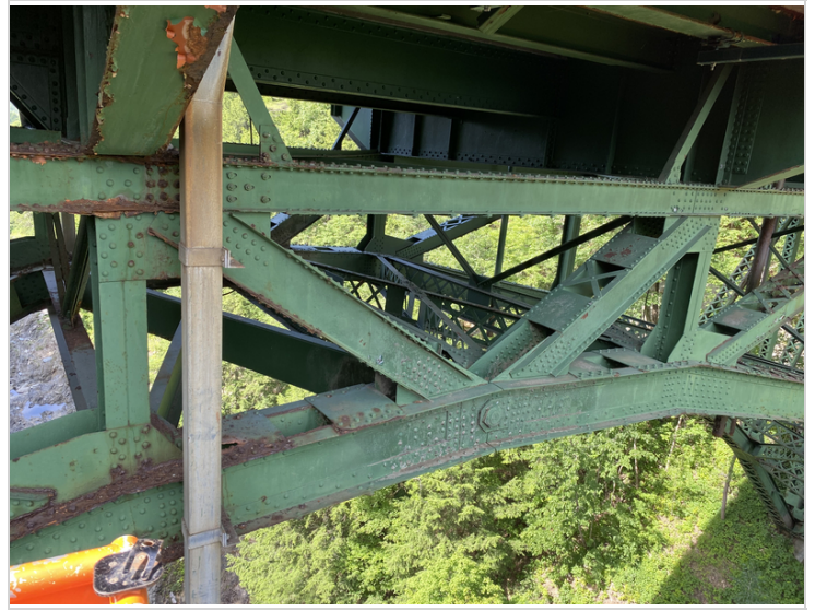
Upstream Center Section between Floorbeams #5 and #6
