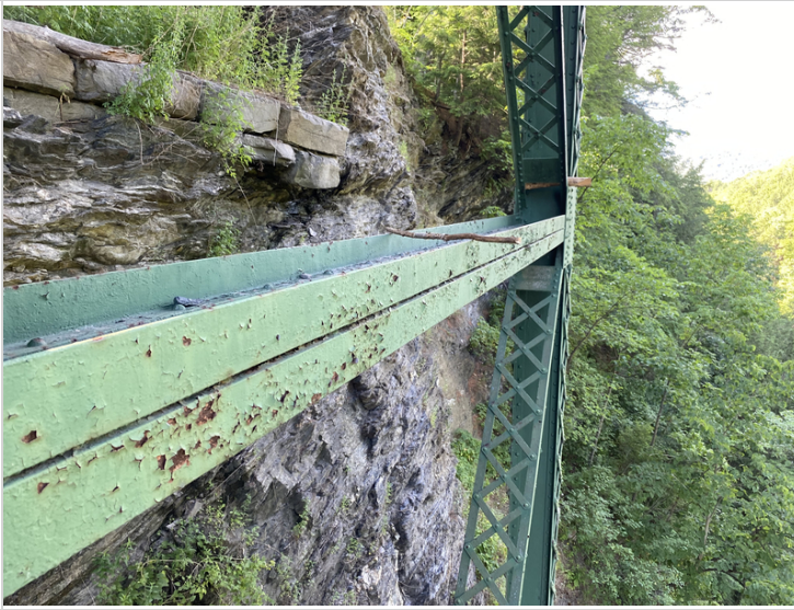
Cross Bracing below Floor Beam #10
