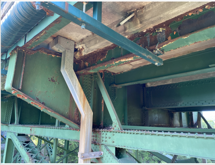
Beam #2 at Floor Beam #6
