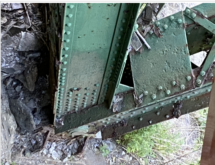
Upstream Bearing below vertical #10
