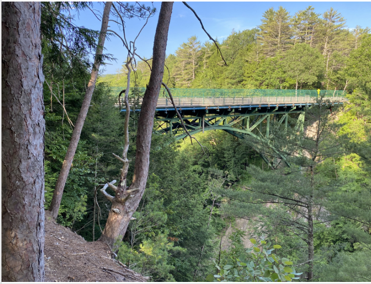
Upstream Structure Elevation
