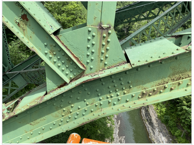
Downstream Bottom Chord at Vertical #3 / Gusset
