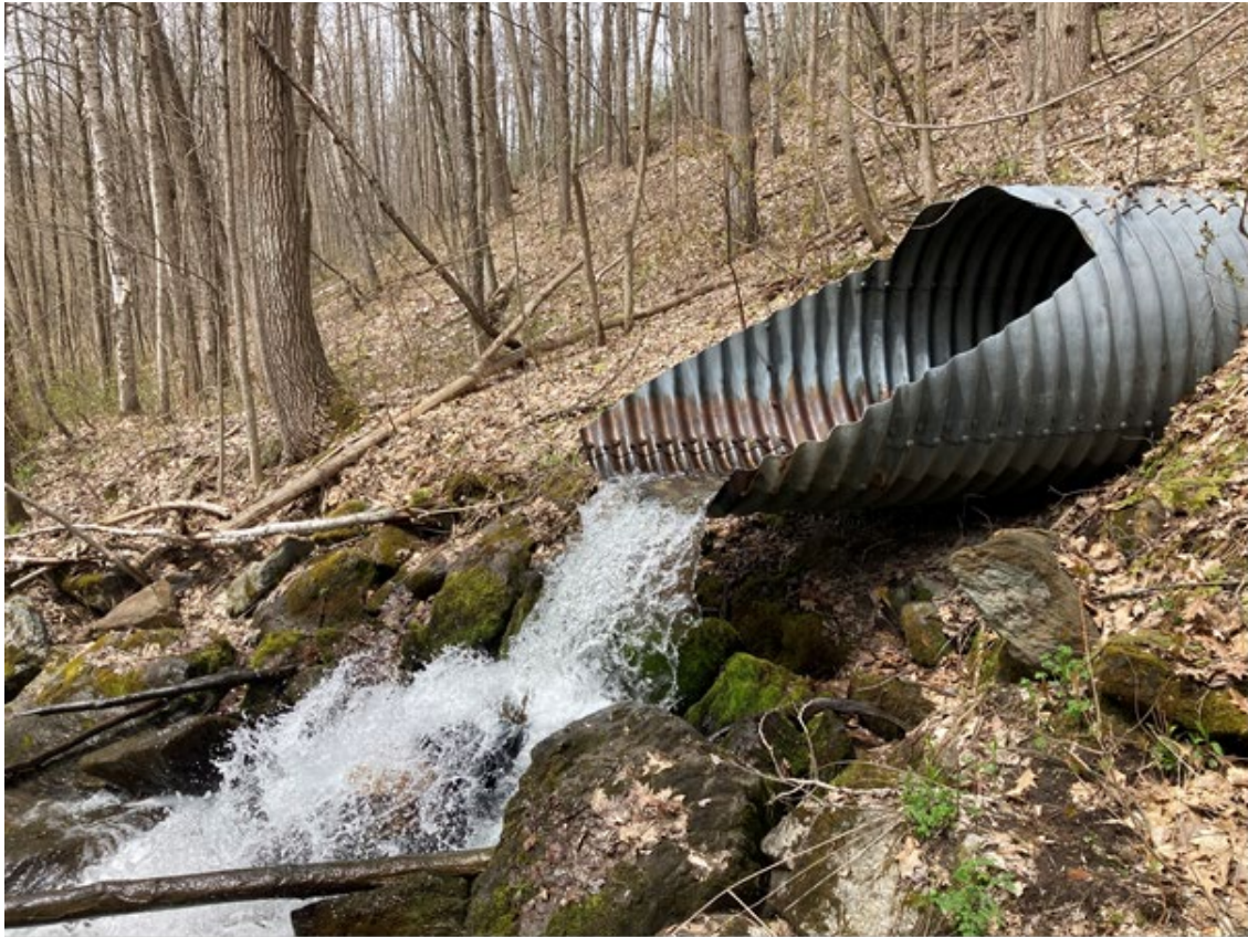
Culvert outlet
