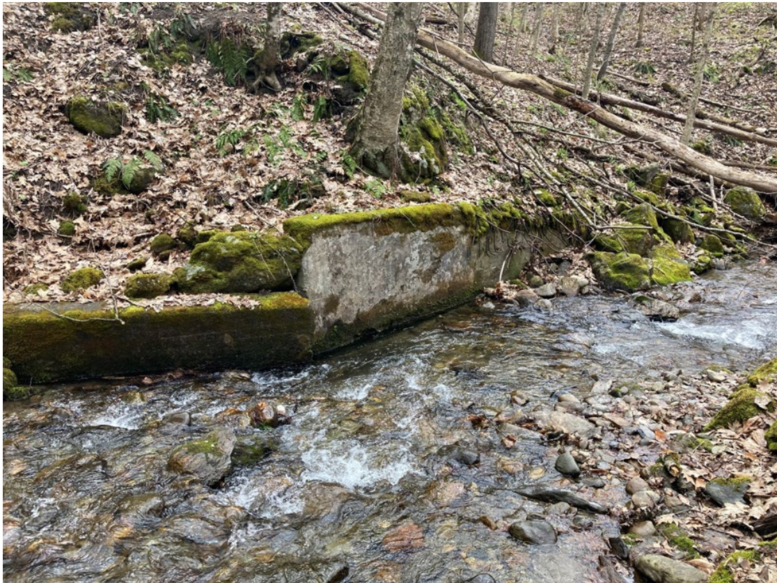
Concrete headwall
