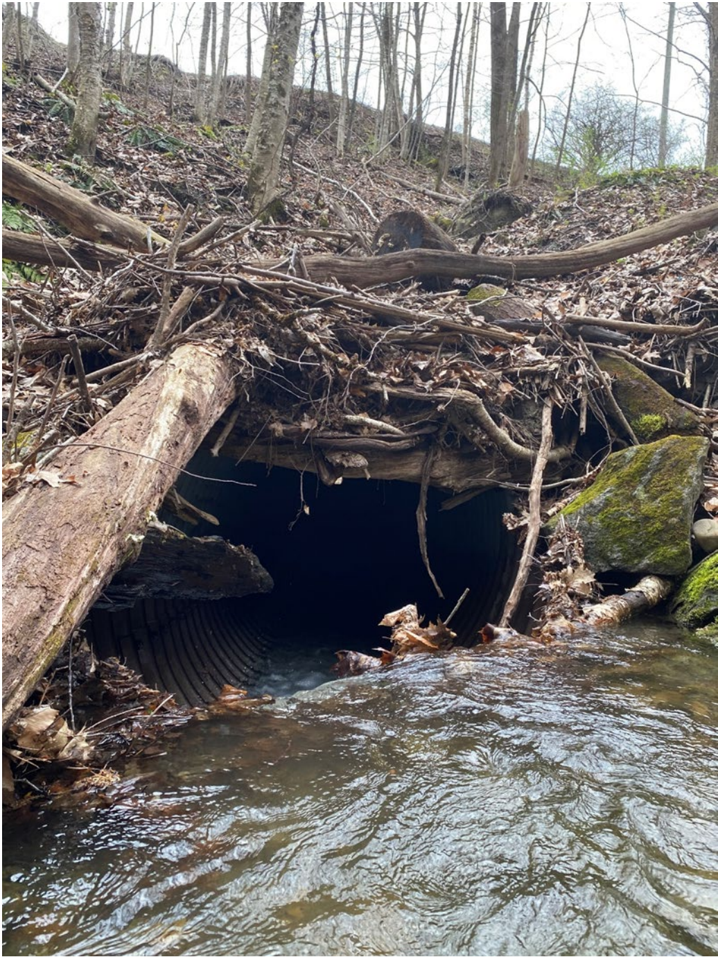
Culvert inlet
