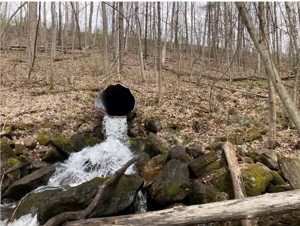
Outlet of PID68002 (looking north)
