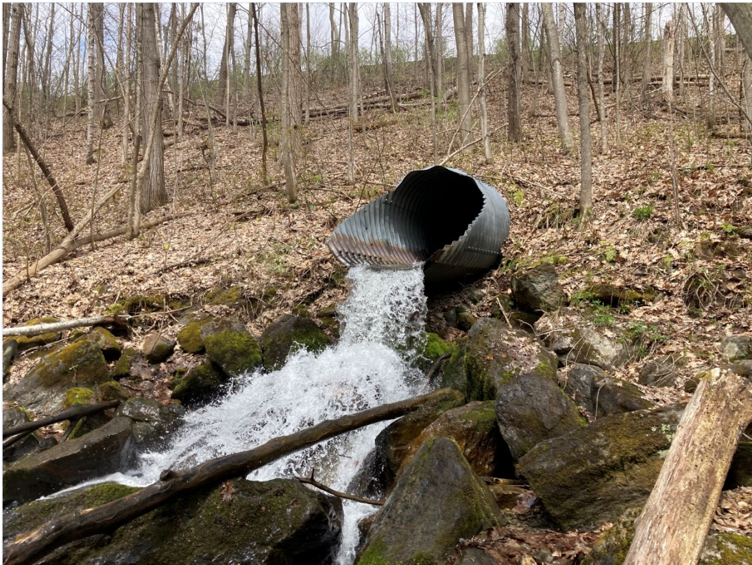
Figure 1: Outlet of the Pipe Showing Steep Wooded Embankment
