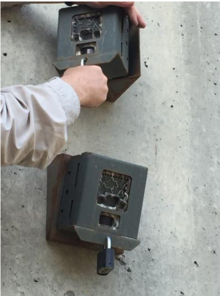
Cameras being installed on abutment, one angled down, the other angled to the side
