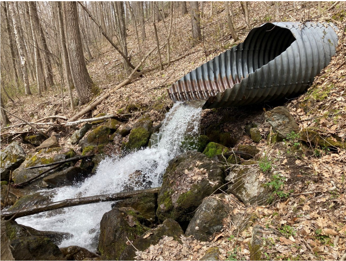
Profile of outlet perch PID68002
