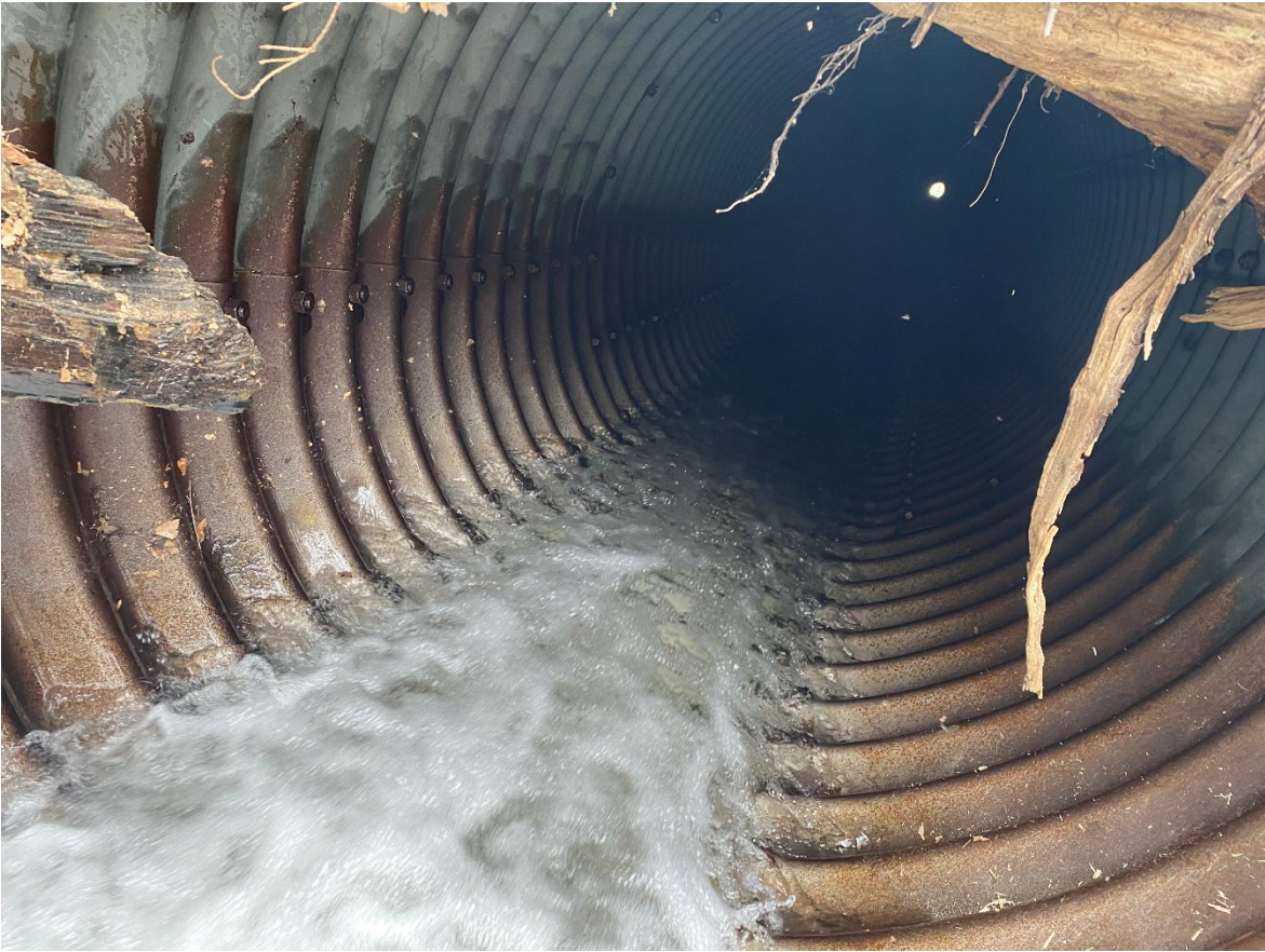
Looking through the culvert from inlet side.
