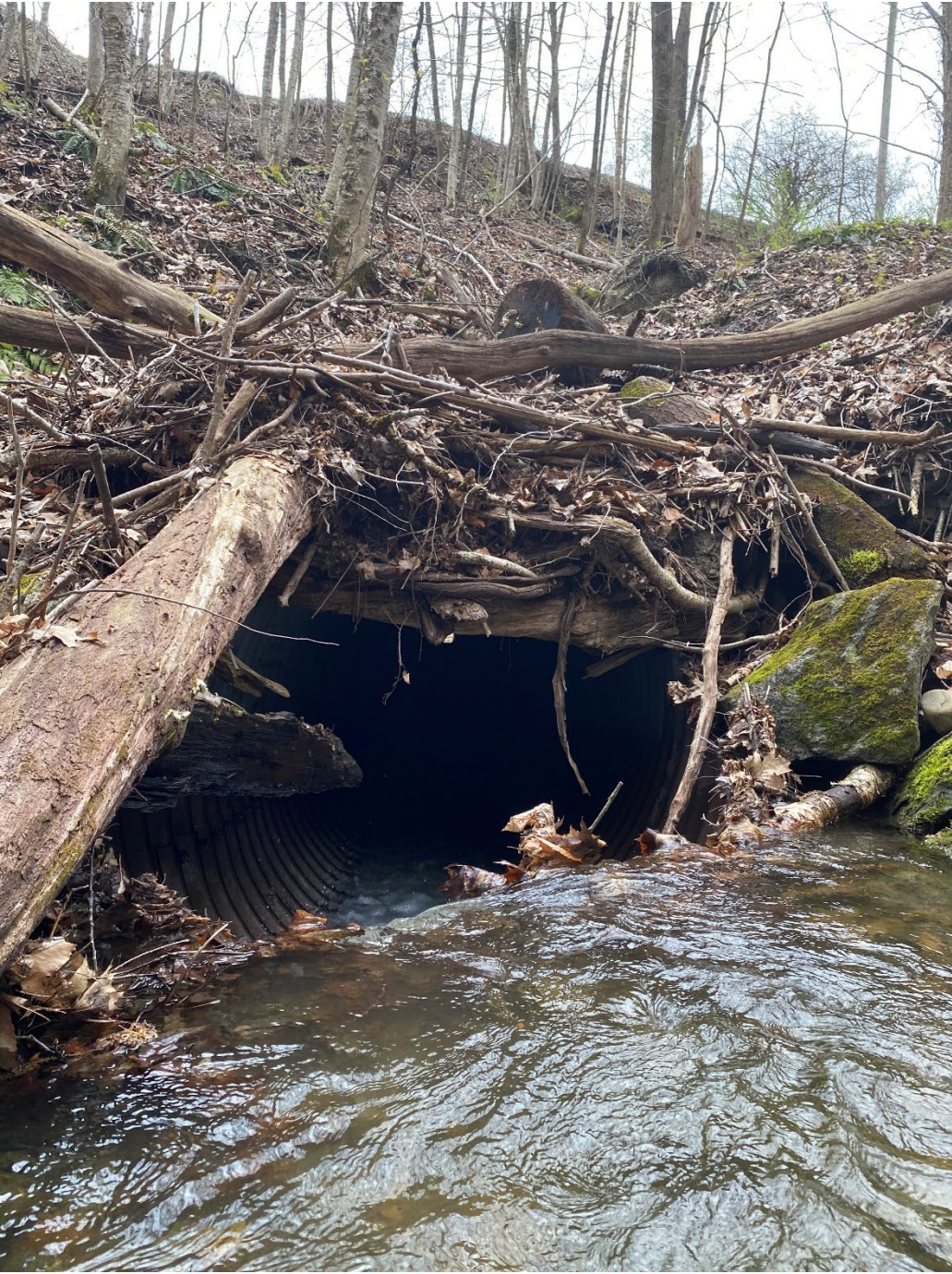
Close up of inlet at PID68002
