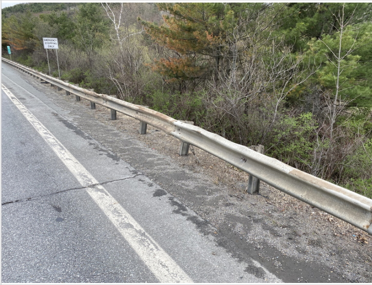
Typical Approach Rail Abutment #1 End West Side
