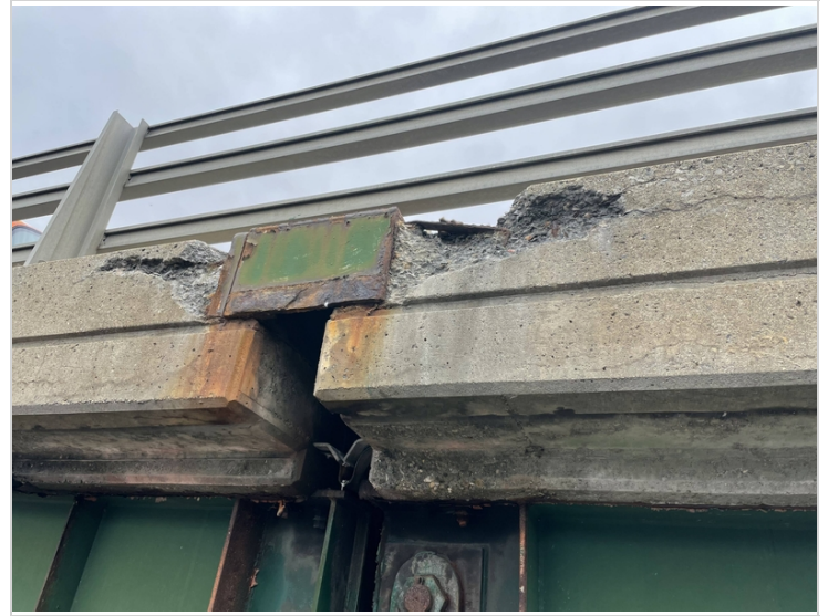
Fascia at Joint in Span #2 West Side
