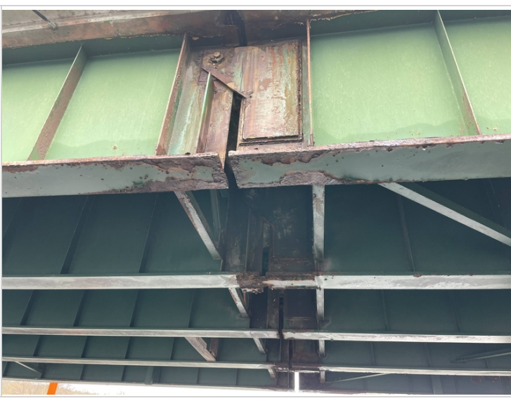
Full View of North Pin Assembly in Span #2
