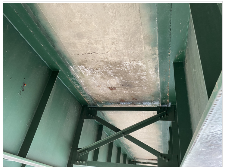
Bay #3 Deck Soffit in Span #3
