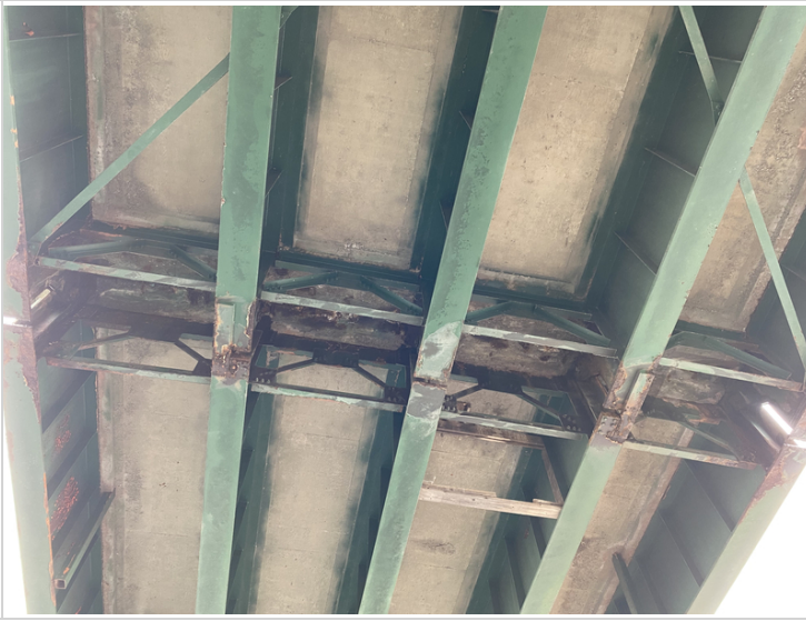
Superstructure at Second Pin Segments
