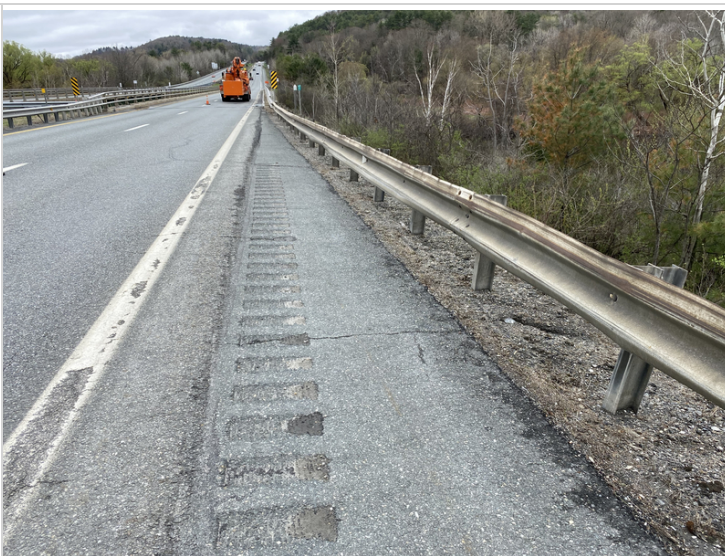
Western Approach Rail at Abutment #2
