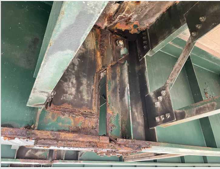
Northern Set of Pins on Beam #2 in Span #2
