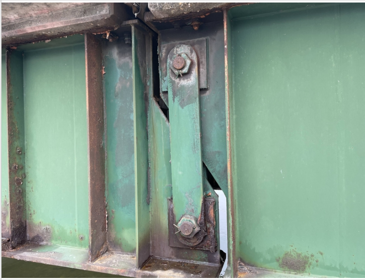
Beam #5 Span #2 First Pin Assembly
