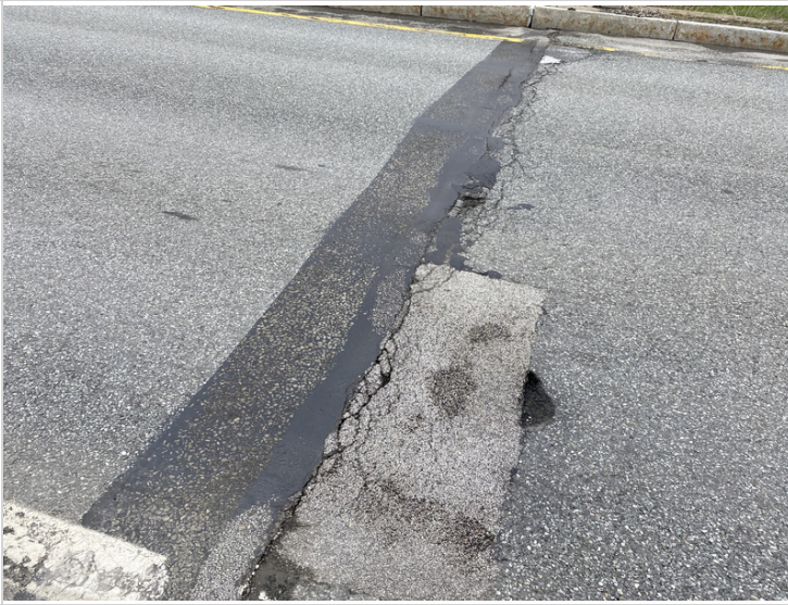
Asphaltic Plug Joint over Abutment #1
