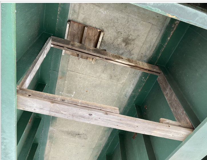
Bay #2 Span #2 Timber Bunking
