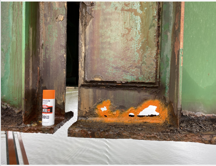
Beam #5 in Span #2 at Second Pin Section
