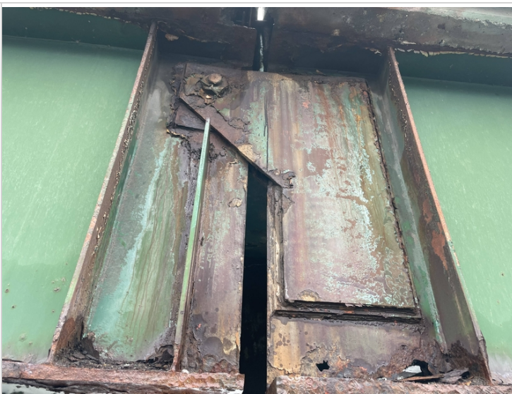
Beam #5 North Side of Span #2 Pin
