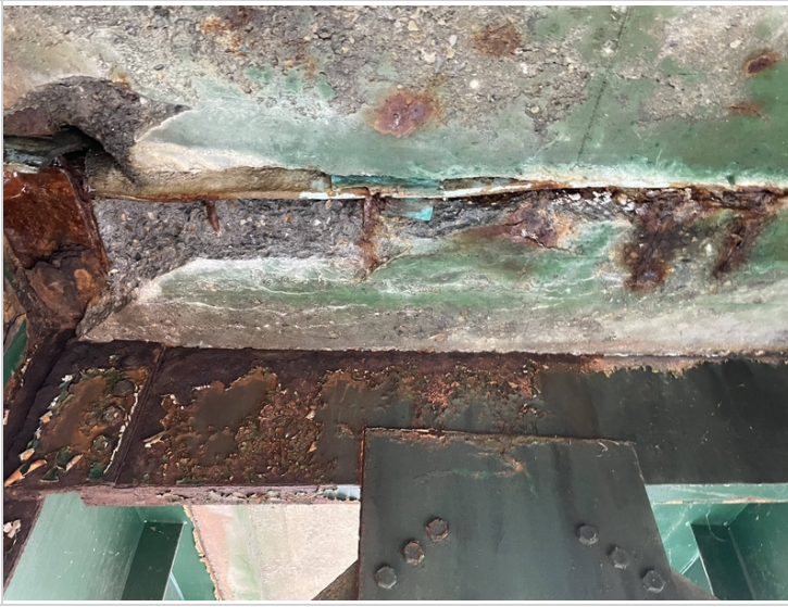
Concrete Underside at Joint over Span #2 Second Pin Assembly
