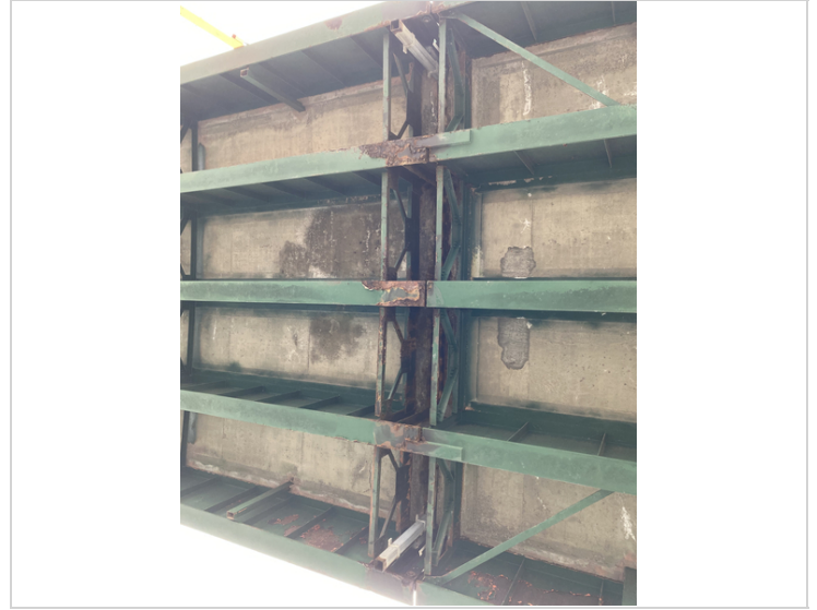
First Section of Pins in Span #2 Superstructure
