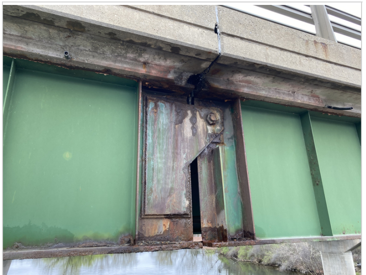
Beam #1 Second Pin Span #2
