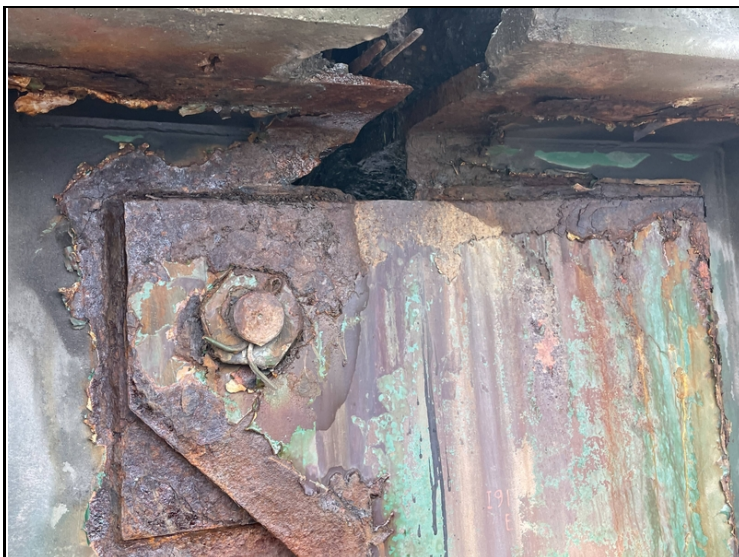
Beam #5 Pin Joint Top Flange (A1)
