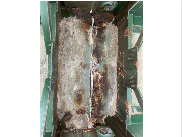
Bay #3 Deck Soffit at Second Pin Segment in Span #2
