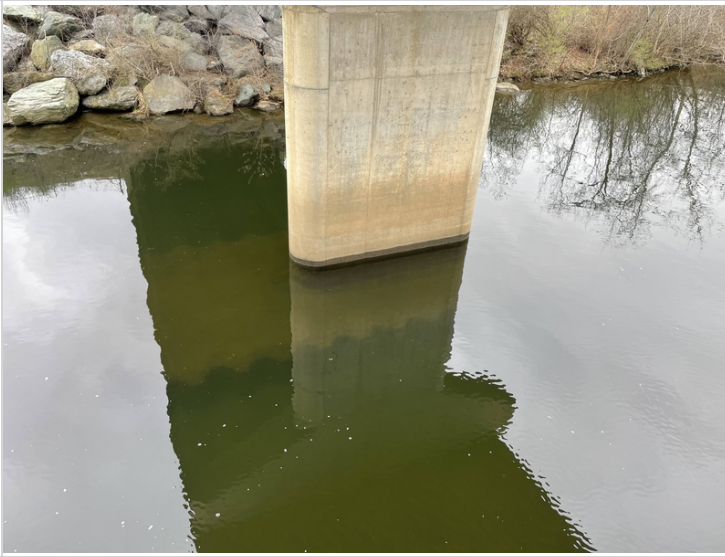
Pier #1 Footing and Steel pile
