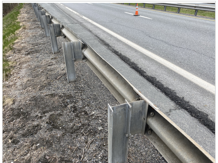
Typical Rail West Side
