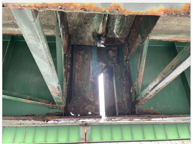
Pin at North Set of Pins on Beam #5 in Span #2
