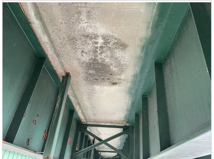
Span #3 Bay #4 Deck Underside
