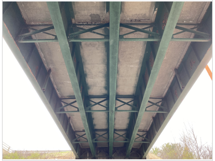
Deck Soffit Span #1
