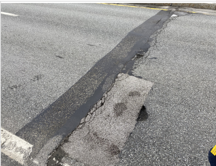
Abutment #1 Asphaltic Plug Joint
