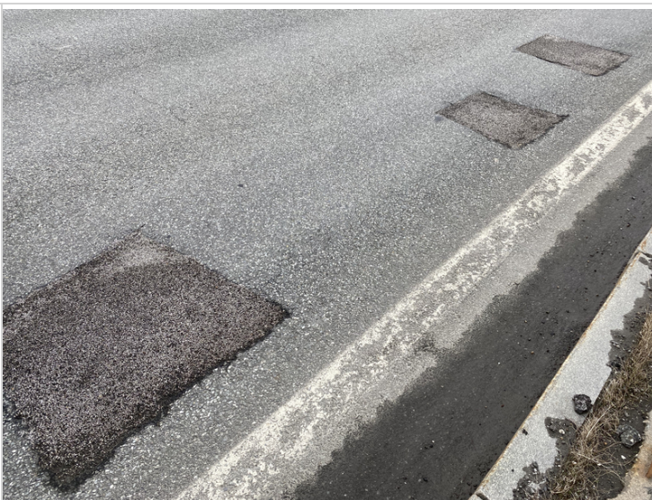
Span #3 Deck Wearing Surface
