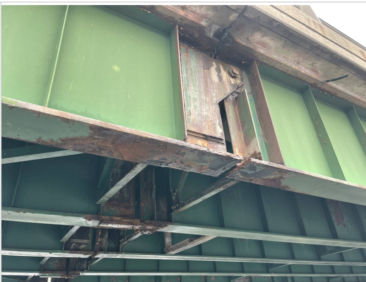
Span #2 Northern Sections of Pins from Beam #1
