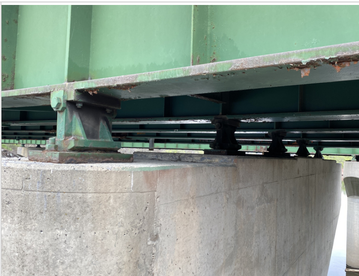
Rocker Bearings over Pier #1
