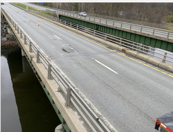
Deck Wearing Surface from Span #1
