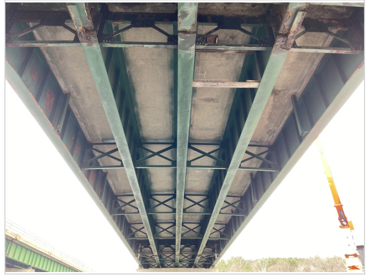
Span #2 Deck Soffit from Pier #2
