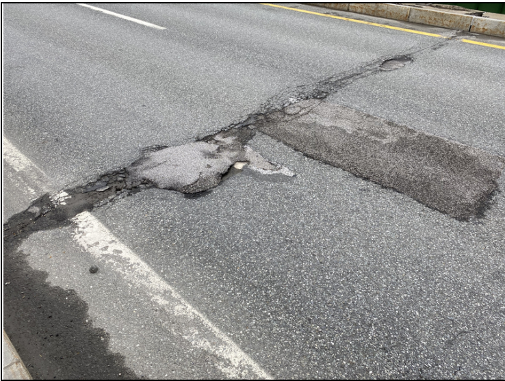
Joint / Asphalt over Second Pin Section in Span #2
