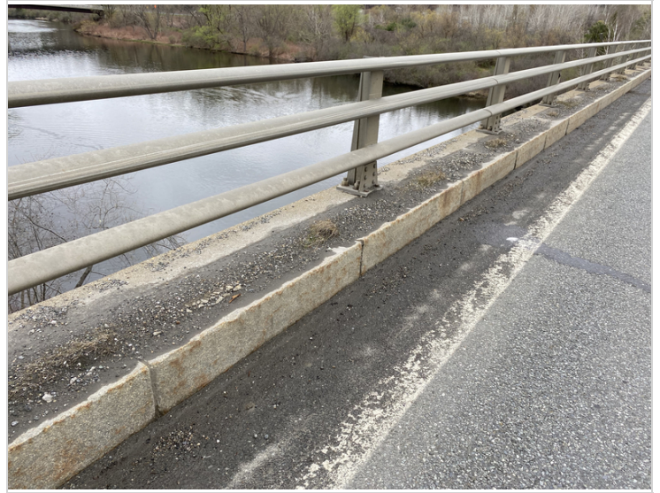
Typical Bridge Rail
