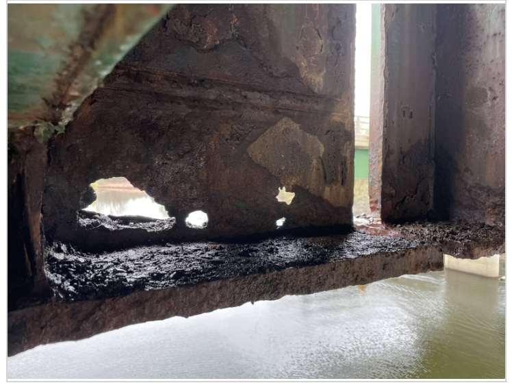
Beam #5 North Side of Span #2 Pin
