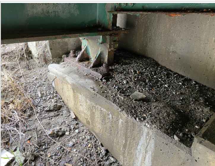
Bearing #5 at Abutment #1
