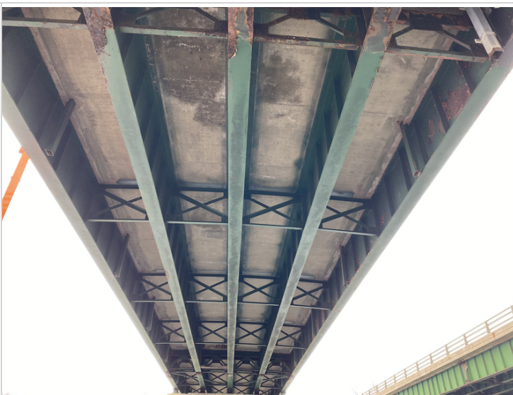
Span #2 Deck Soffit
