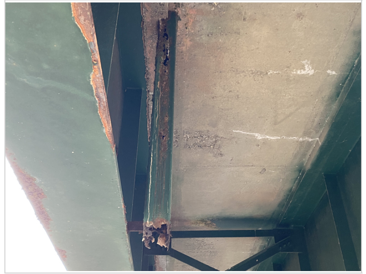
Deck Drain along Bay #4 in Span #1
