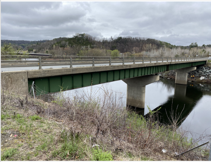
Downstream Elevation (Southeast Corner)
