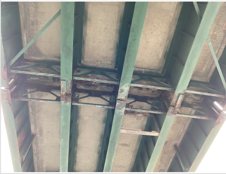
Span #2 Second Section of Pins
