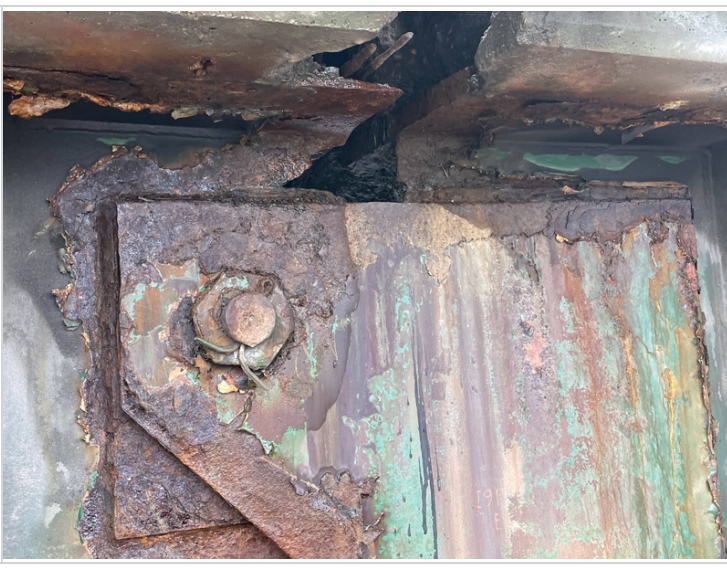
Beam #5 Pin Joint Top Flange (A1)
