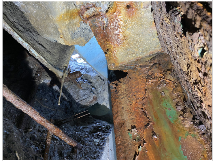
Girder #5 End over Abutment #2
