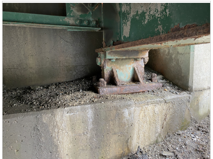
Bearing #1 at Abutment #1
