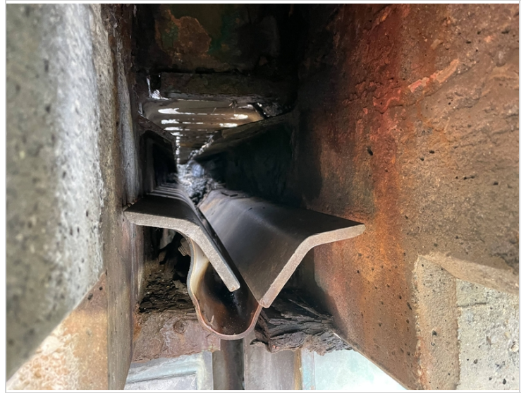
Joint Trough over First Pin Section in Span #2
