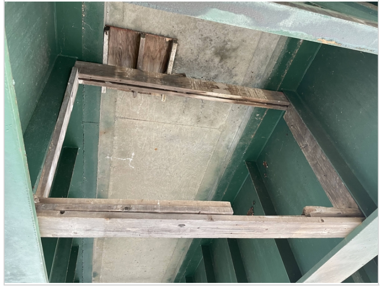
Wood Form along Deck in Span #2
