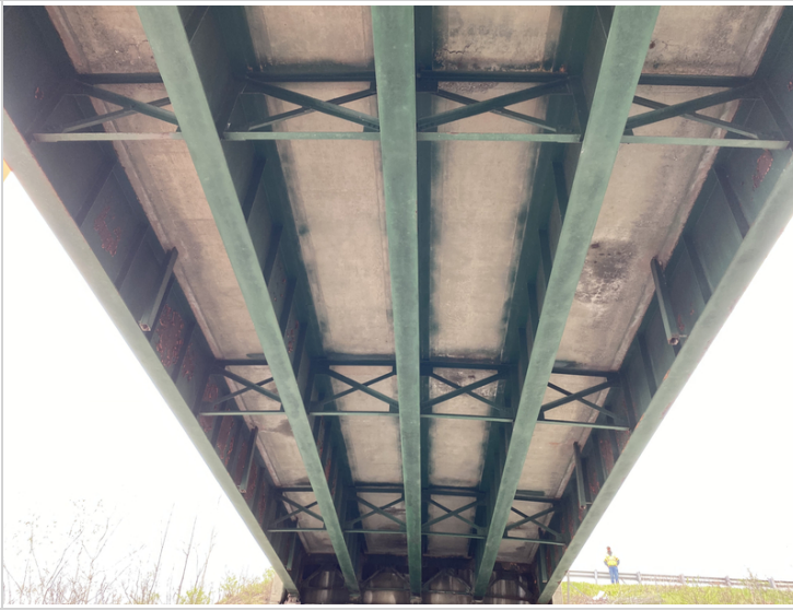
Span #3 Deck Soffit
