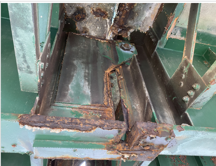
Beam #4 at Second Pin Section in Span #2
