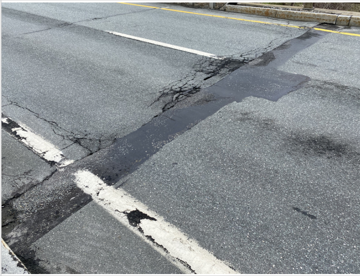
Asphaltic Plug Joint over Abutment #1
