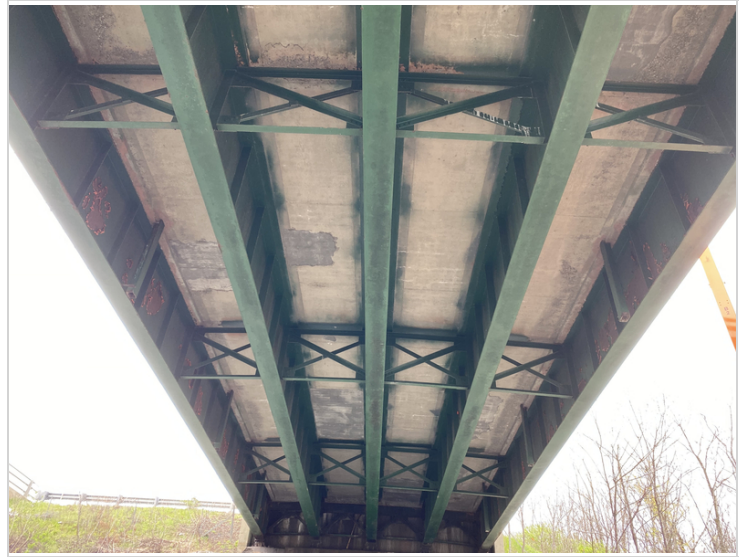
Deck Soffit Span #3
