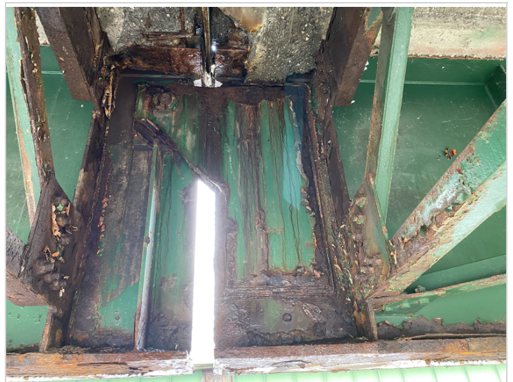
Girder #1 at Second Section of Pins in Span #2
