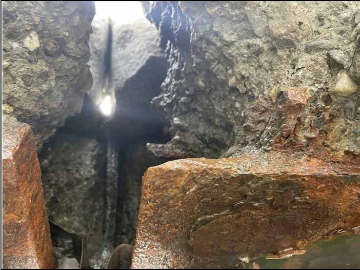
Pin Assembly Girder #1 In Span #2 Second
