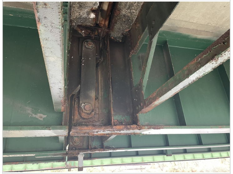
Pin Assembly Girder #3 In Span #2 First Section
