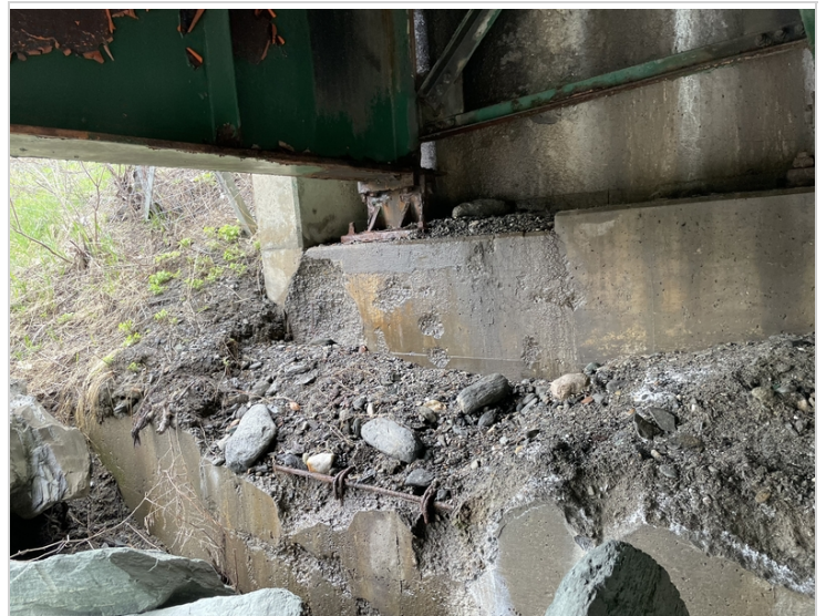
West End of Abutment #2
