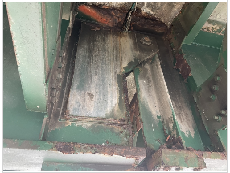
Pin Assembly Girder #4 In Span #2 Second Section
