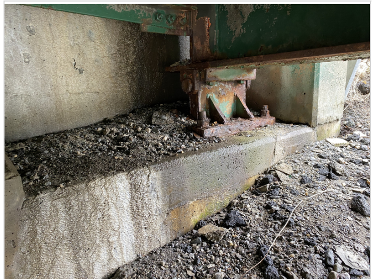
Bearing #1 at Abutment #1
