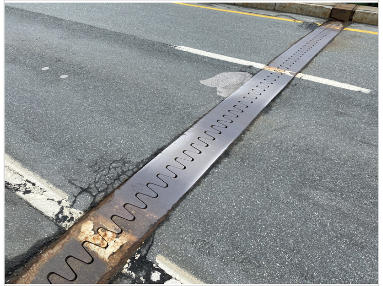
Steel Finger Joint over Pin Section #1 in Span #2
