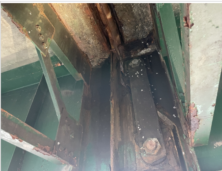
Pin Assembly Girder #2 In Span #2 First Section
