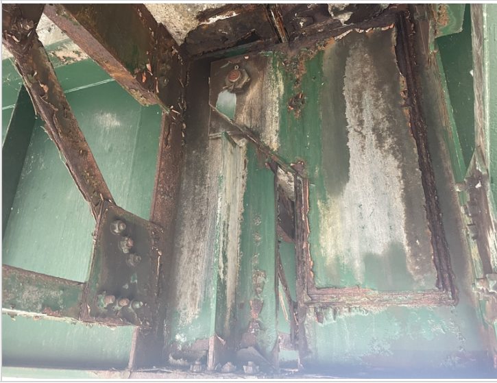
Pin Assembly Girder #3 In Span #2 Second Section
