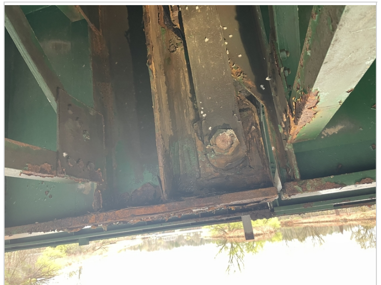
Pin Assembly Girder #2 In Span #2 First Section
