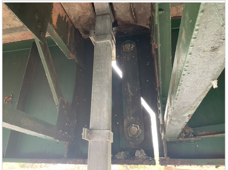
Pin Assembly Girder #5 In Span #2 First Section
