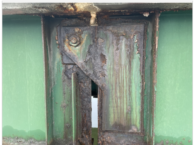
Pin Assembly Girder #5 In Span #2 Second Section
