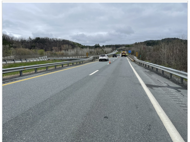
Southern Approach Looking North
