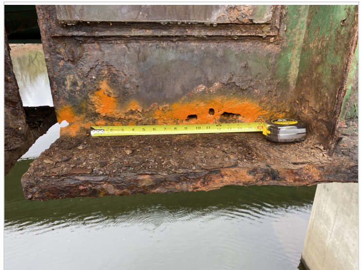
Girder #5 at Second Section of Pins in Span #2
