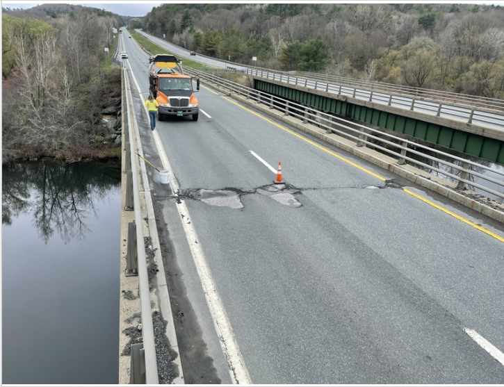
Deck Joint at North Pin Assembly
