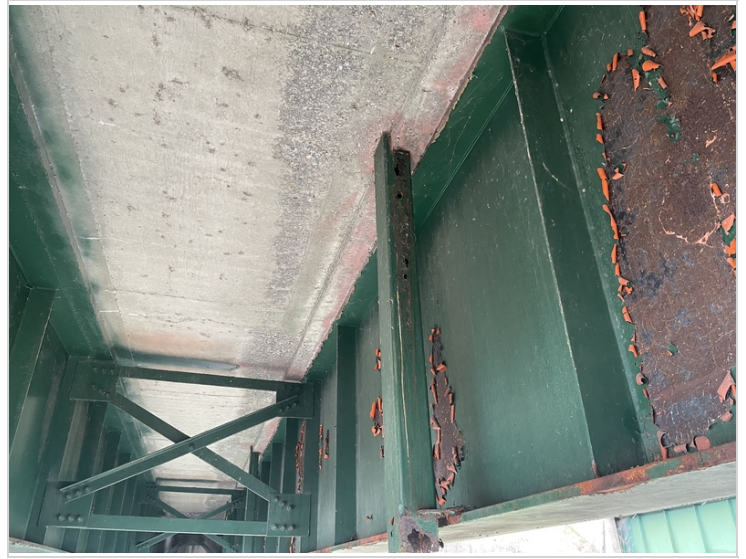
Span #2 Bay #1 Deck Drain Downspout
