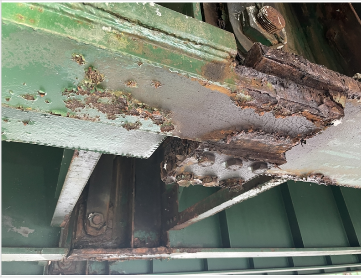
Pin Support at Girder #4 In Span #2 First Section
