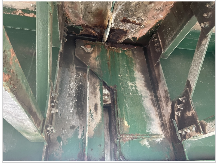
Pin Assembly Girder #4 In Span #2 Second Section
