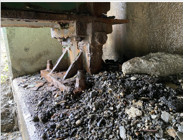
Bearing #1 at Abutment #2
