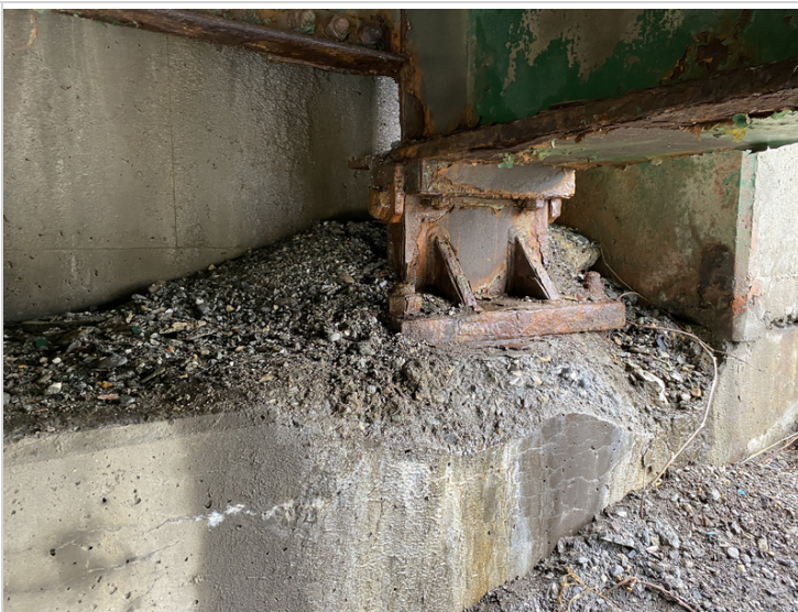
Bearing #5 at Abutment #2
