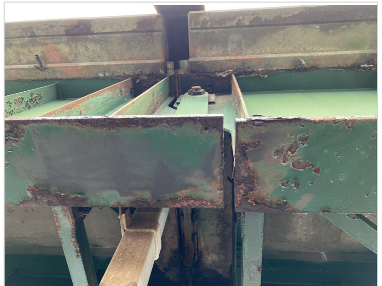
Girder #5 in Span #2 First Pin Section
