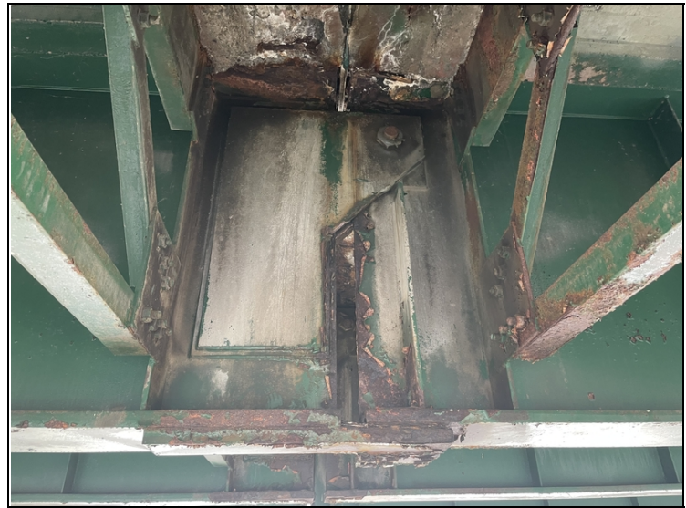
Pin Assembly Girder #2 In Span #2 Second Section
