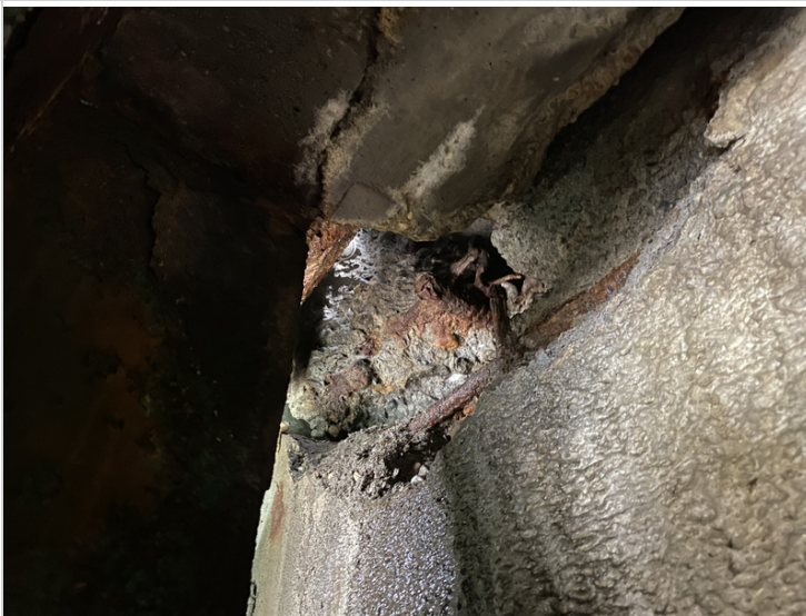
Backwall behind Girder #5 at Abutment #1
