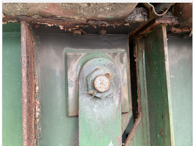
Pin Assembly Girder #1 in Span #2 First Section
