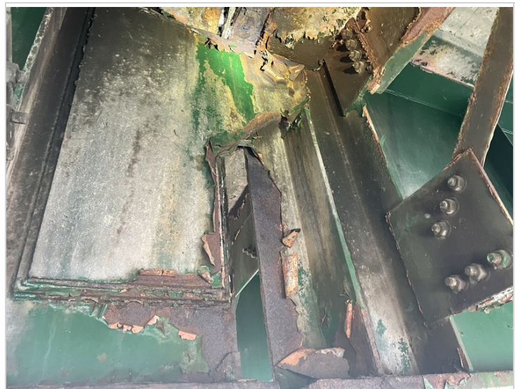
Pin Assembly Girder #2 In Span #2 Second Section
