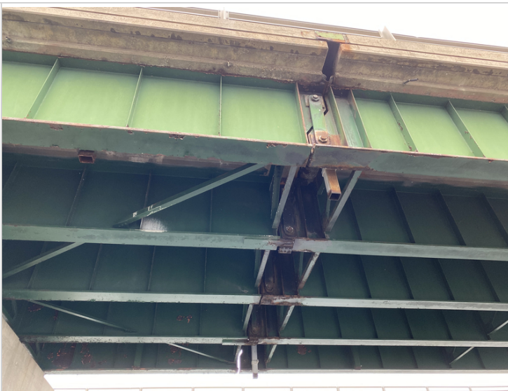
Span #2 First Section of Pins
