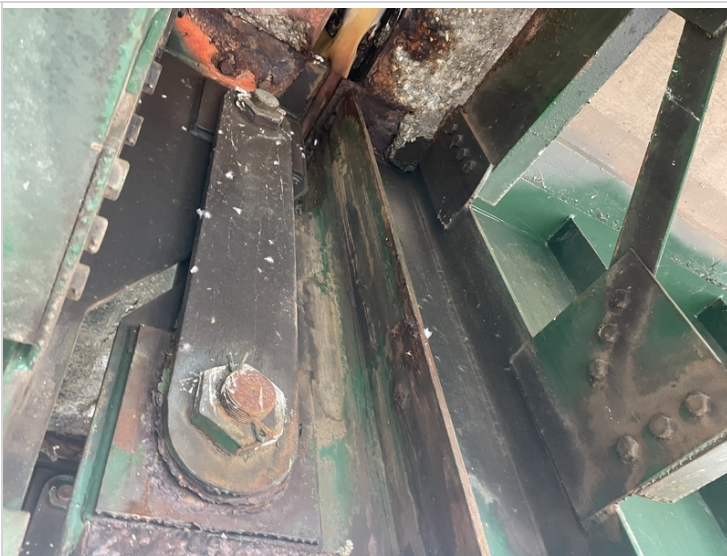
Pin Assembly Girder #4 In Span #2 First Section
