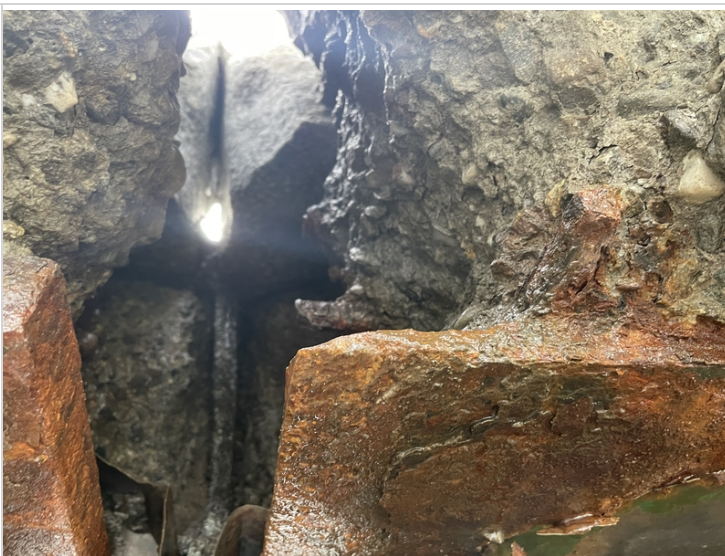
Pin Assembly Girder #1 In Span #2 Second Section Hole Through Curb
