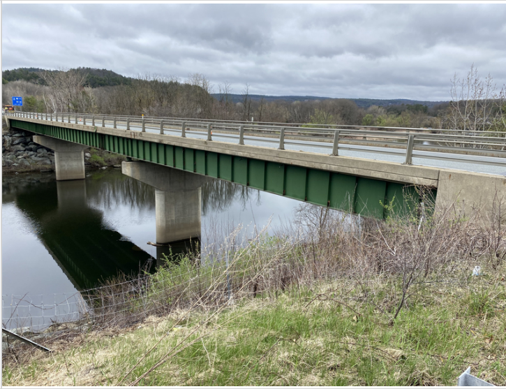
Upstream Elevation from Abutment #1
