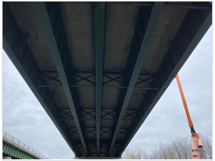
Span #2 Deck Soffit
