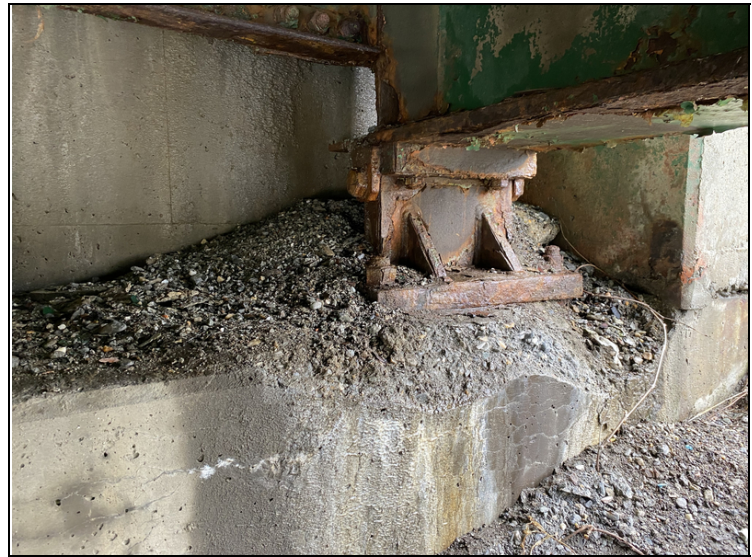
Bearing #5 at Abutment #2
