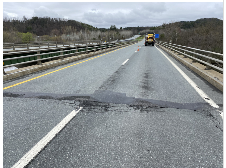
Deck Wearing Surface from Abutment #1
