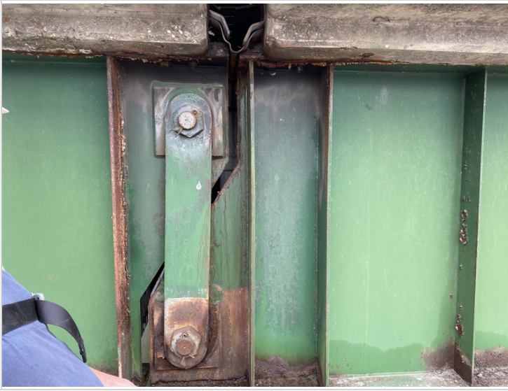
Girder #5 in Span #2 First Pin Section
