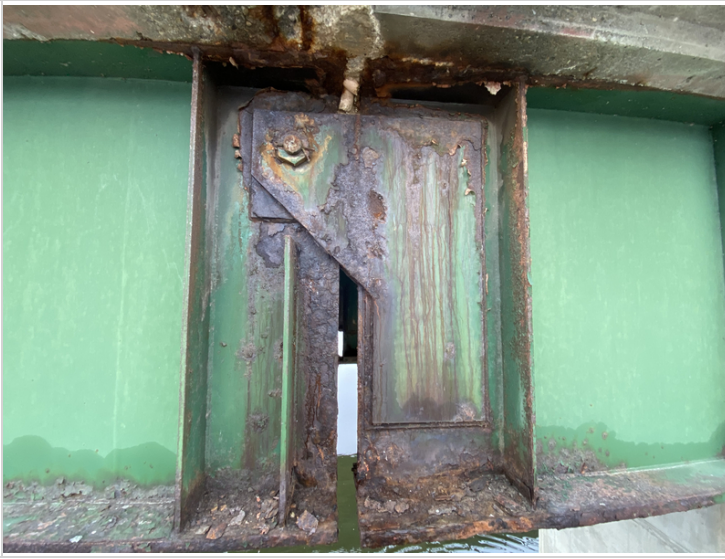
Girder #5 at Second Sections of Pins in Span #2
