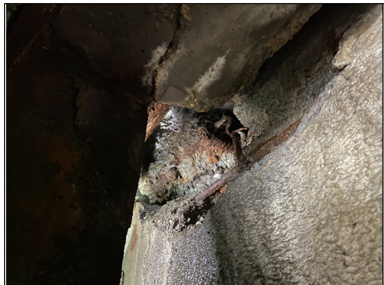
Backwall behind Girder #5 at Abutment #1
