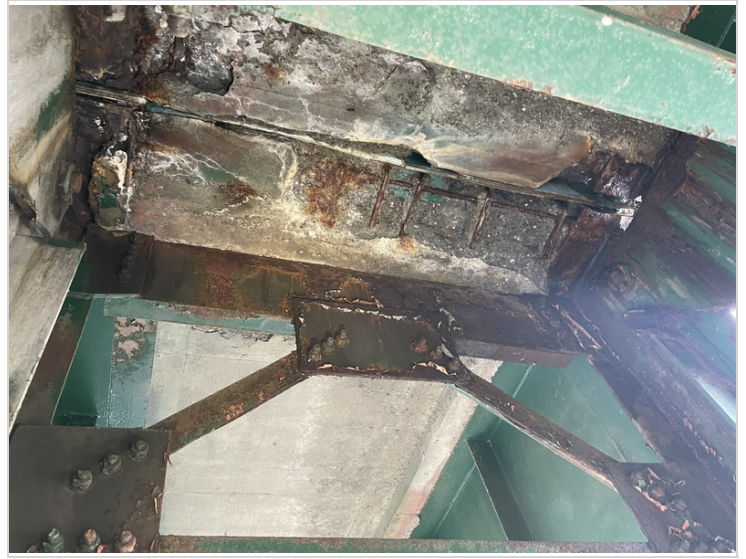
Deck Underside at Second Section of Span #2 Pins
