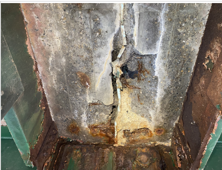
Concrete Deck Soffit over Second Section of Pins in Span #2
