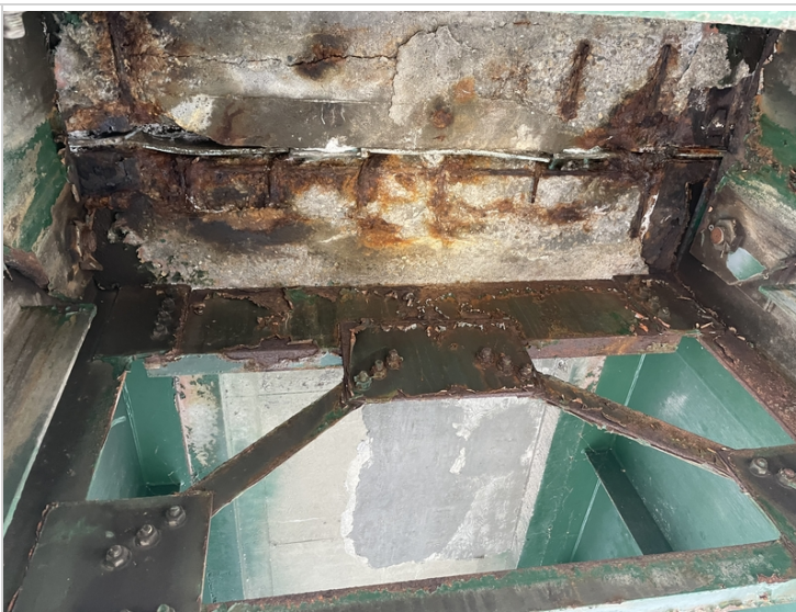
Deck Underside at Second Section of Span #2 Pins
