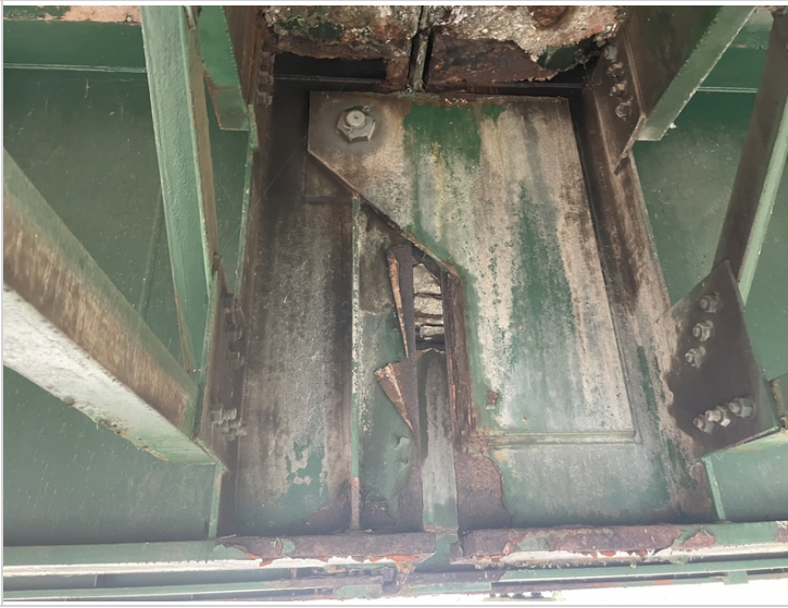
Pin Assembly Girder #3 In Span #2 Second Section
