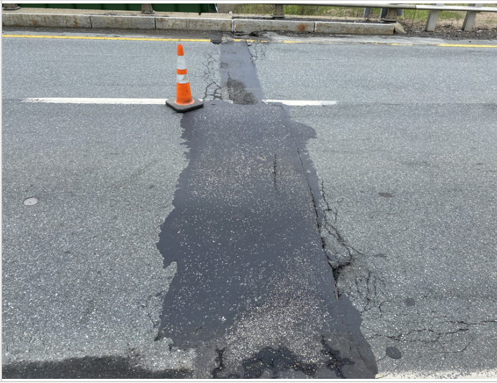
Asphaltic Plug Joint over Abutment #2
