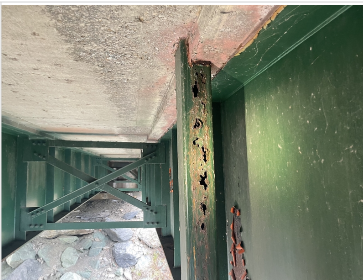
Span #1 Bay #1 Deck Drain Downspout
