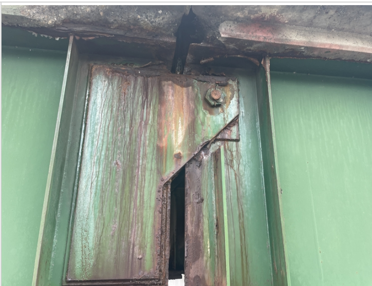
Pin Assembly Girder #1 In Span #2 Second Section
