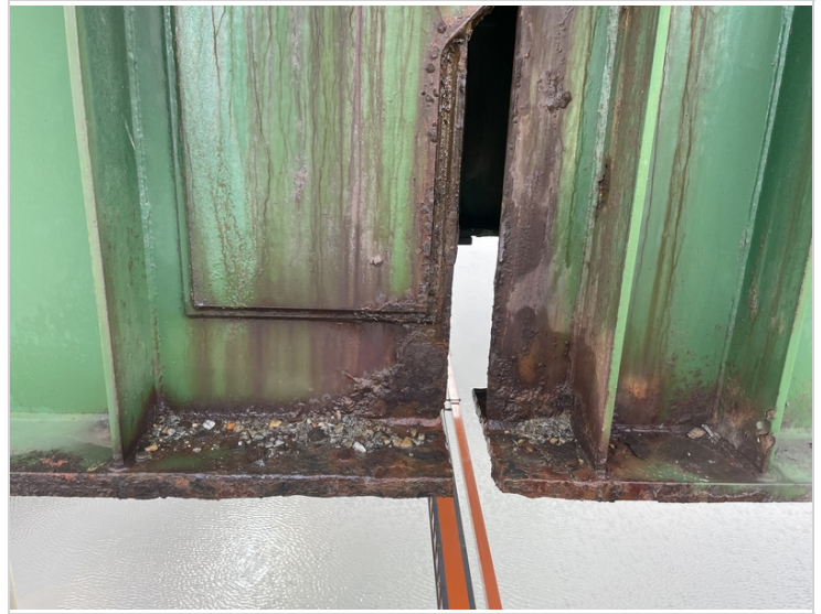
Pin Assembly Girder #1 In Span #2 Second Section
