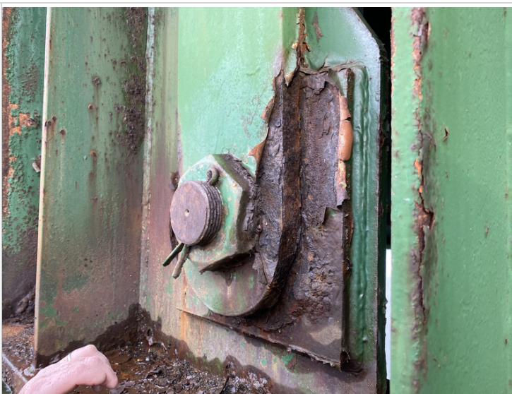
Girder #1 in Span #2 First Pin Section
