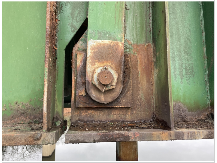
Pin Assembly Girder #5 In Span #2 First Section
