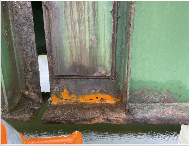
Pin Assembly Girder #5 In Span #2 Second Section
