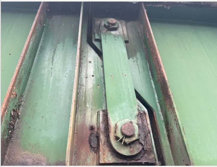
Pin Assembly Girder #1 In Span #2 First Section
