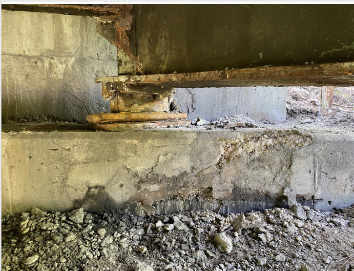
Bearing #1 at Abutment #1
