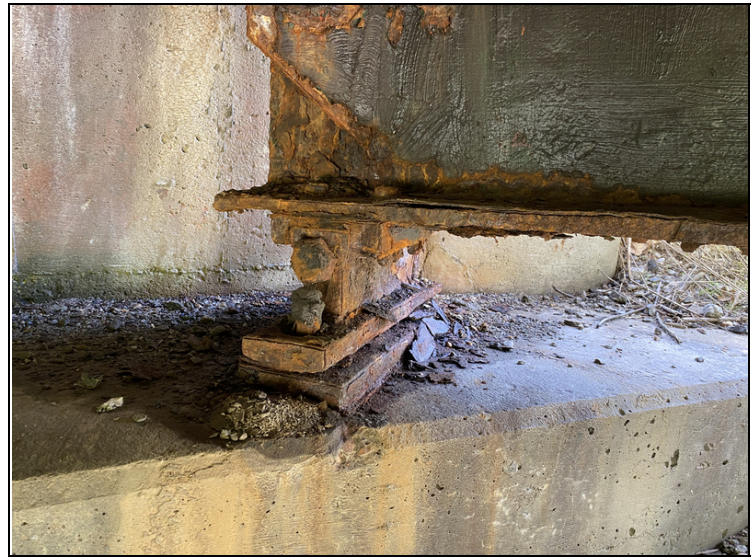
Bearing #5 at Abutment #2
