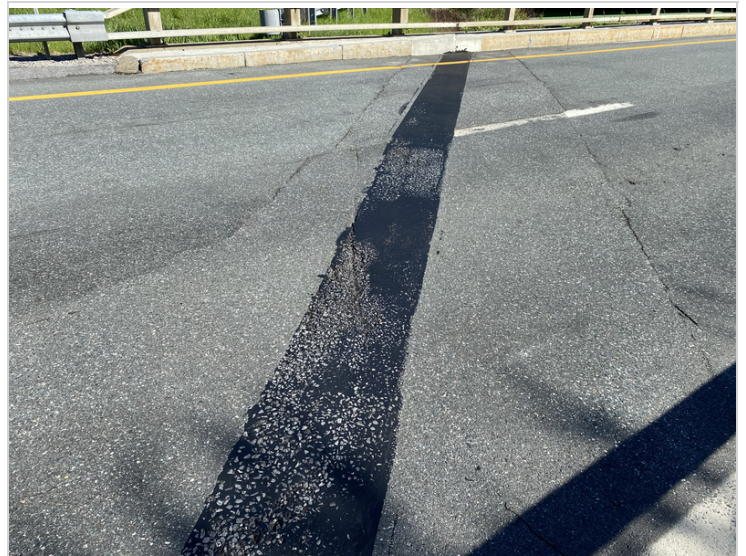
Asphaltic Plug Joint over Abutment #1
