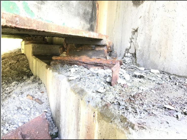
Bearing #1 at Abutment #1
