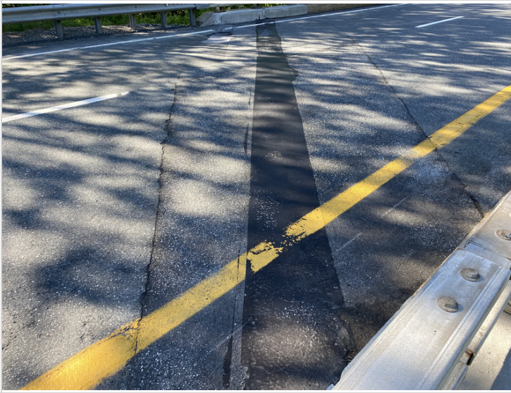
Asphaltic Plug Joint over Abutment #2
