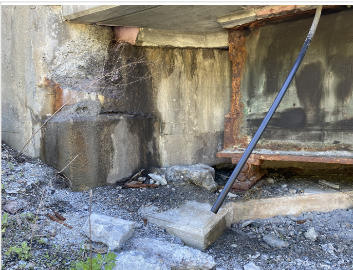
West End Abutment #2
