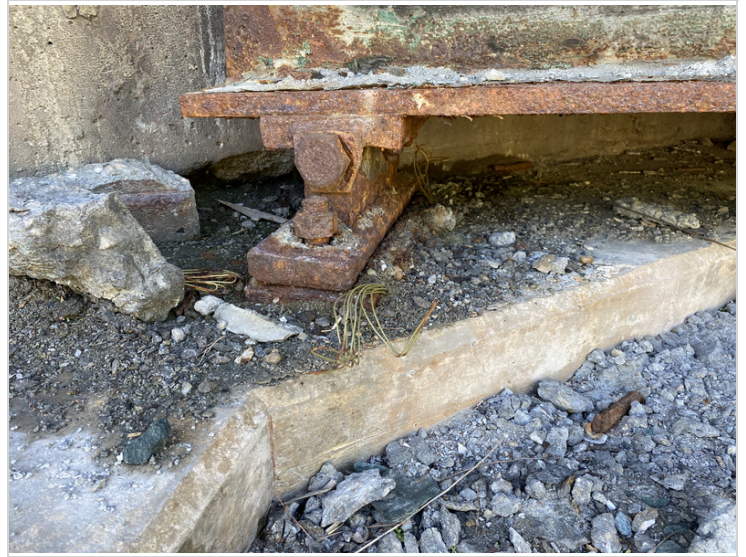
Bearing #1 at Abutment #2
