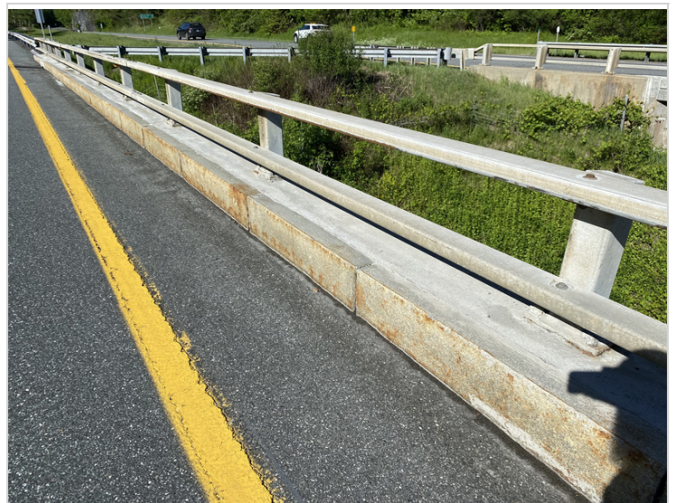
Western Repaired Curb / and Bridge Rail
