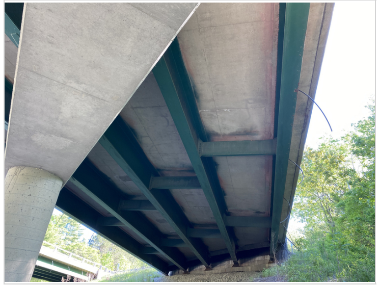
Span #3 Superstructure
