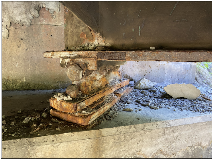
Bearing #5 at Abutment #2
