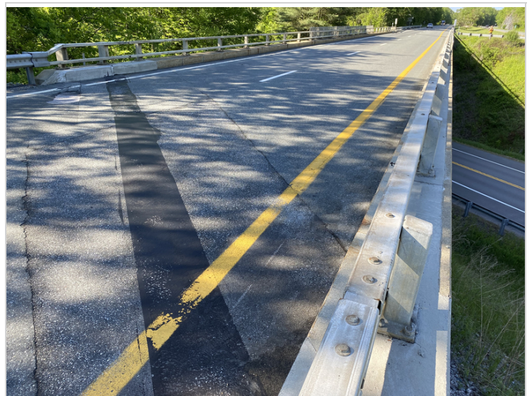
Deck Wearing Surface from Abutment #2
