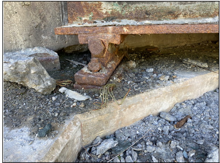
Bearing #1 at Abutment #2
