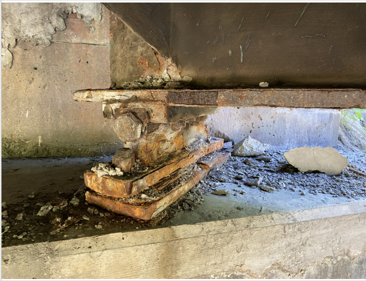
Bearing #5 at Abutment #2
