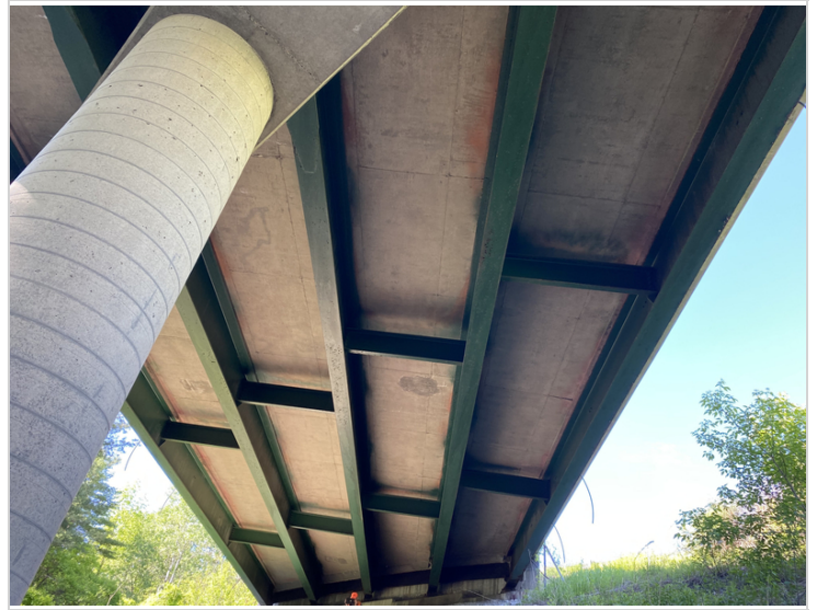
Span #1 Deck Soffit
