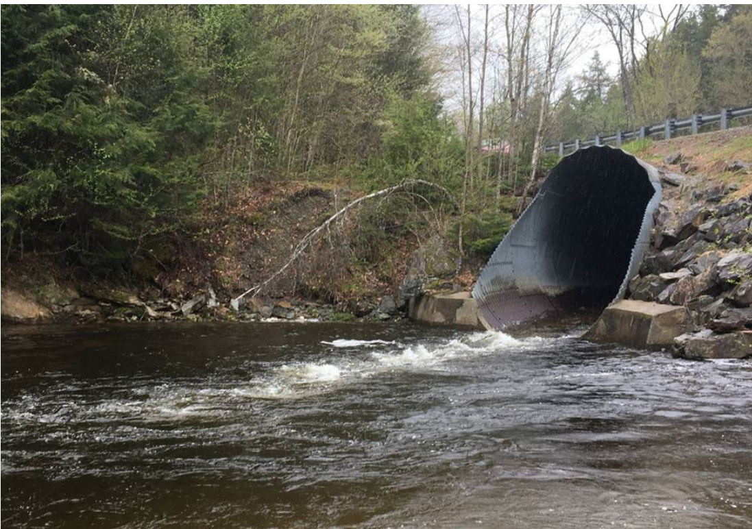
Picture 4: Culvert Outlet
