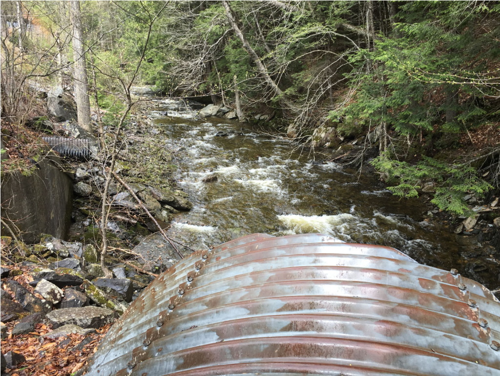
Picture 6: Looking Upstream
