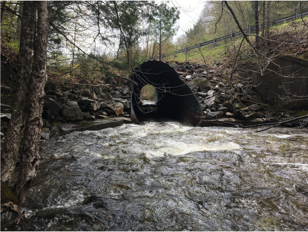
Picture 3: Culvert Inlet
