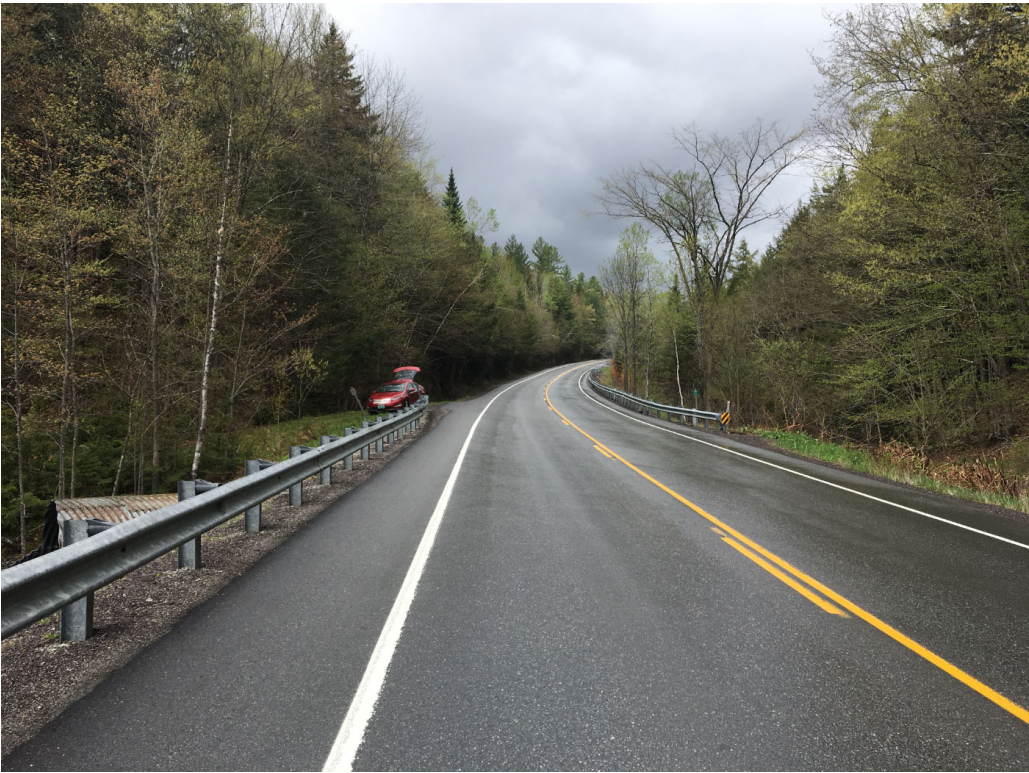
Picture 2: Looking South on VT Route 12 over Bridge 89
