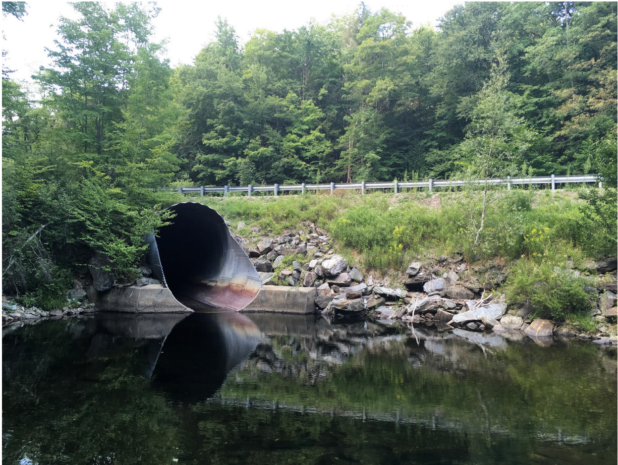
Photo of culvert from west side of the road
