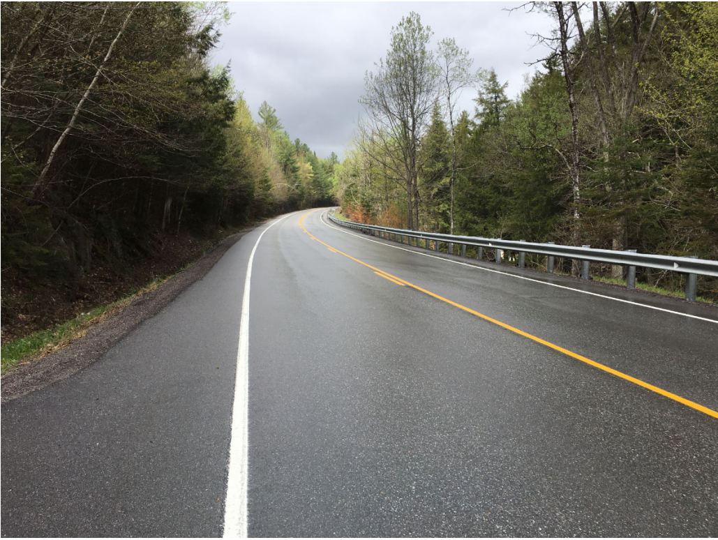
Picture 1: Looking North on VT Route 12 over Bridge 89
