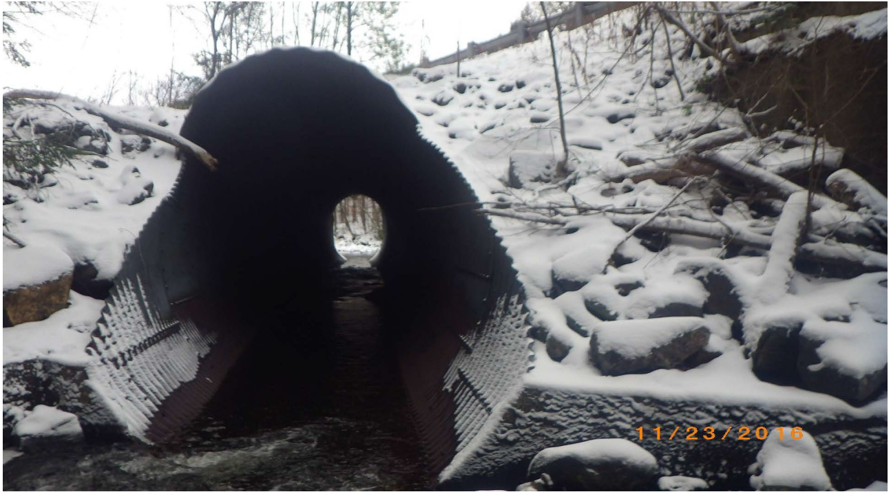
Figure 2: Culvert 89 in Worcester on VT-12.
